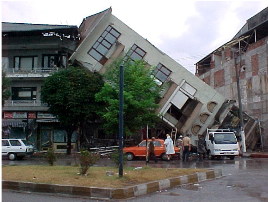
Overturning of slender building on shallow foundation in Adapazari, Turkey during the 1999 Kocaeli Earthquake (Observation made at N40.7841 E30.3998 on 8/25/99 at 1240).
