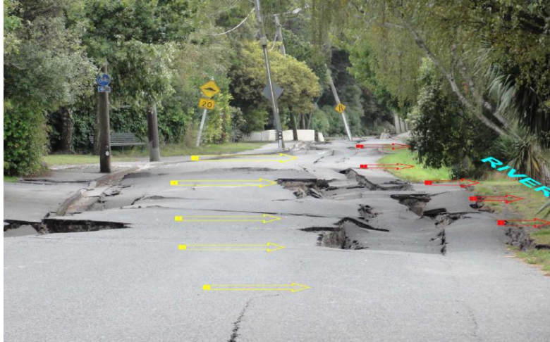
Figure 4-23. Example of lateral spreading along the Avon River.
