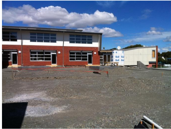
Figure 5-30. Settlement of ground around the roped off buried tank structure. (-43.508389°, 172.612489°)
