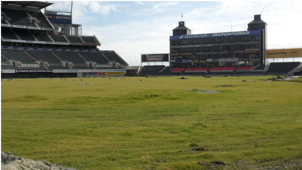
Figure 5-8. Liquefaction “blisters” and sand boils on the AMI Stadium field. (-43.541397°, 172. 654521°)
