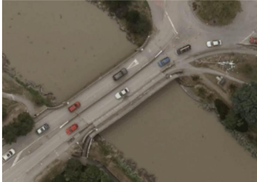
Figure 7-25. Satellite image of Wainoni Road Bridge post-earthquake (LINZ 2011). (-43.5034°, 172.7076°)
