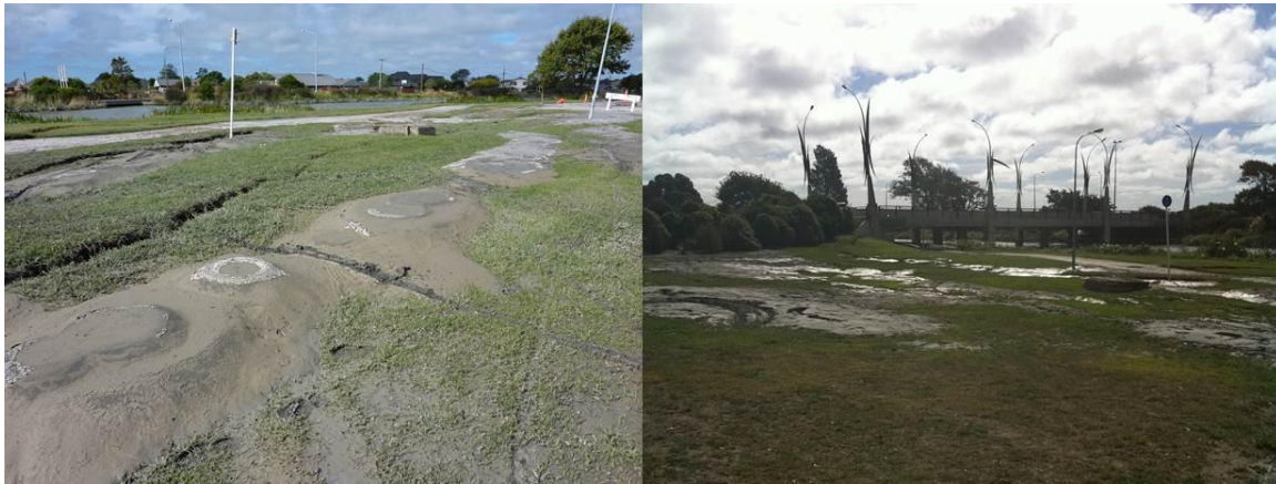
Figure 7-21. Photographs of the lateral spreading and sand boils to the southeast of Anzac Drive Bridge. (-43.50144°, 172.702046°)
