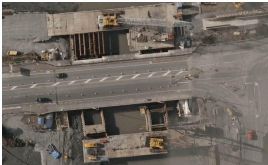
Figure 7-34. Satellite image of Ferrymead Bridge post-earthquake (LINZ 2011). (-43.5584°, 172.7088°)
