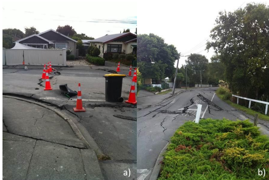
Figure 7-13. Photograph on the (a) east approach looking east and (b) west approach looking north. (-43.5222°, 172.6601°)
