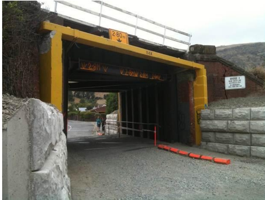
Figure 7-44. Photograph of Railway Bridge 3 after repairs had been made. (-43.575963°, 172.706382°)
