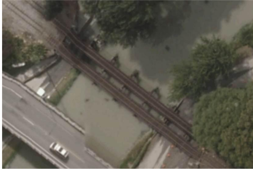
Figure 7-45. Satellite image of Railway Bridge 7 post-earthquake (LINZ 2011). (-43.5529°, 172.6676°)
