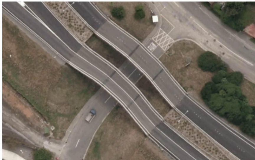
Figure 7-41. Satellite image of Horotane Bridge post-earthquake (LINZ 2011). ( -43.5725^{\circ} , 172.6947^{\circ} )
