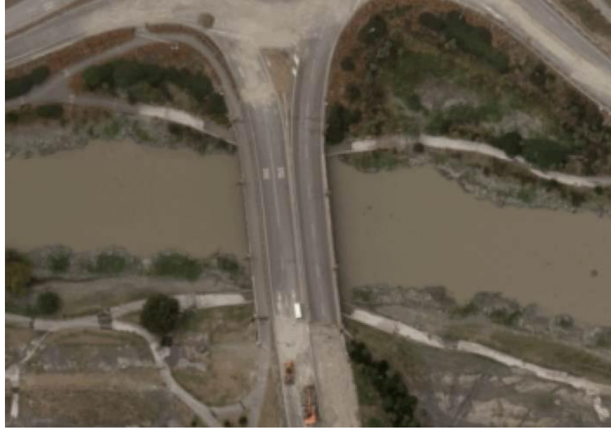
Figure 7-20. Satellite image of Anzac Drive Bridge post-earthquake (LINZ 2011). (-43.5009°, 172.7012°)
