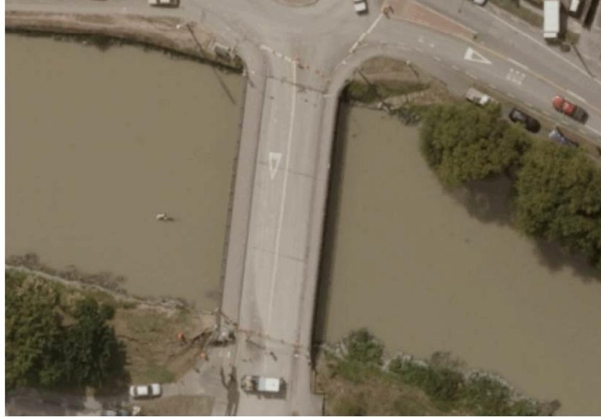
Figure 7-18. Satellite image of Avondale Road Bridge post-earthquake (LINZ 2011). (-43.5005°, 172.6878°)
