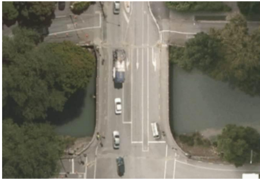
Figure 7-10. Satellite image of Stanmore Road Bridge post-earthquake (LINZ 2011). ( -43.5252^{\circ} , 172.6571^{\circ} )
