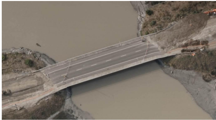
Figure 7-27. Satellite image of South Brighton Bridge post-earthquake (Land Information New Zealand 2011). (-43.5253°, 172.7242°)
