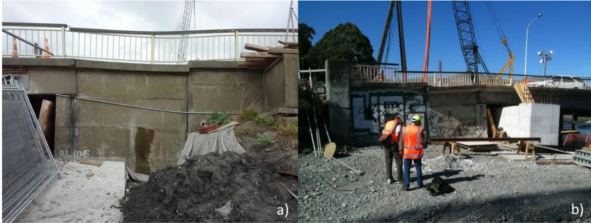
Figure 5-35. Photograph of the east abutment a) looking north and b) looking south. Note the back rotation of the existing abutments and front rotation of the new concrete bridge girder. (-43.5584°, 172.7088°)
