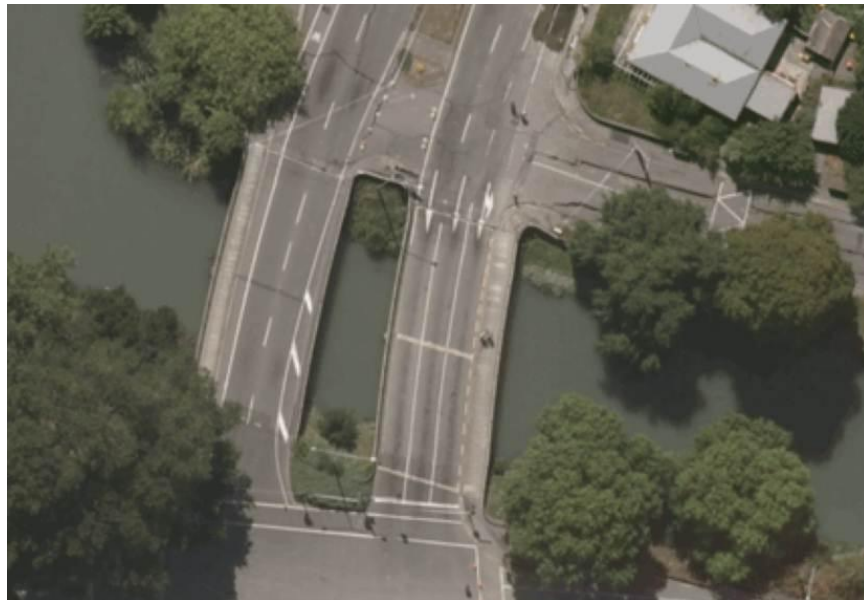
Figure 7-5. Satellite image of Fitzgerald Avenue Bridge post-earthquake (LINZ 2011). (-43.5263°, 172.6506°)
