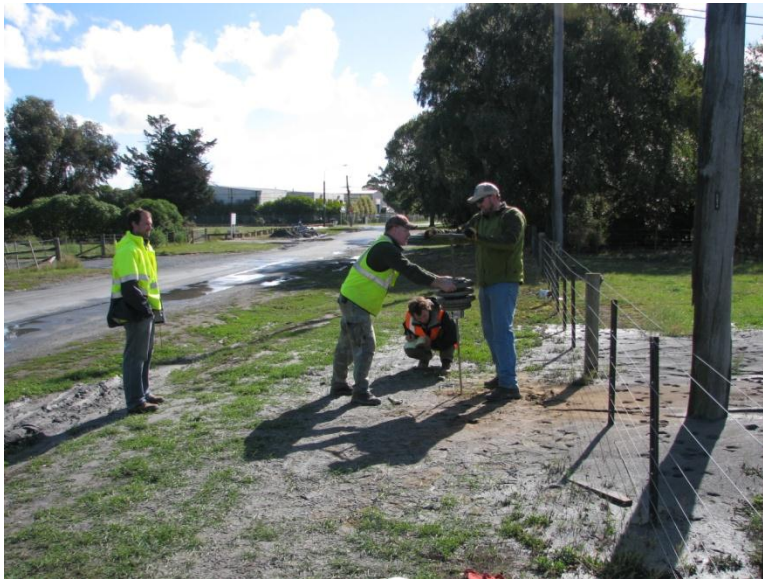
Figure 8-13. Swedish Weight Sounding (SWS) Testing at Bromley Substation (-43.531534°, 172.697942°)
