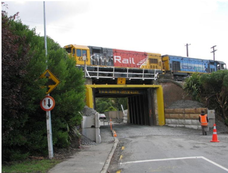
Figure 8-3. Bridge No. 3 at Martindales Road in the Heathcote Valley (-43.576013°, 172.706567°).
