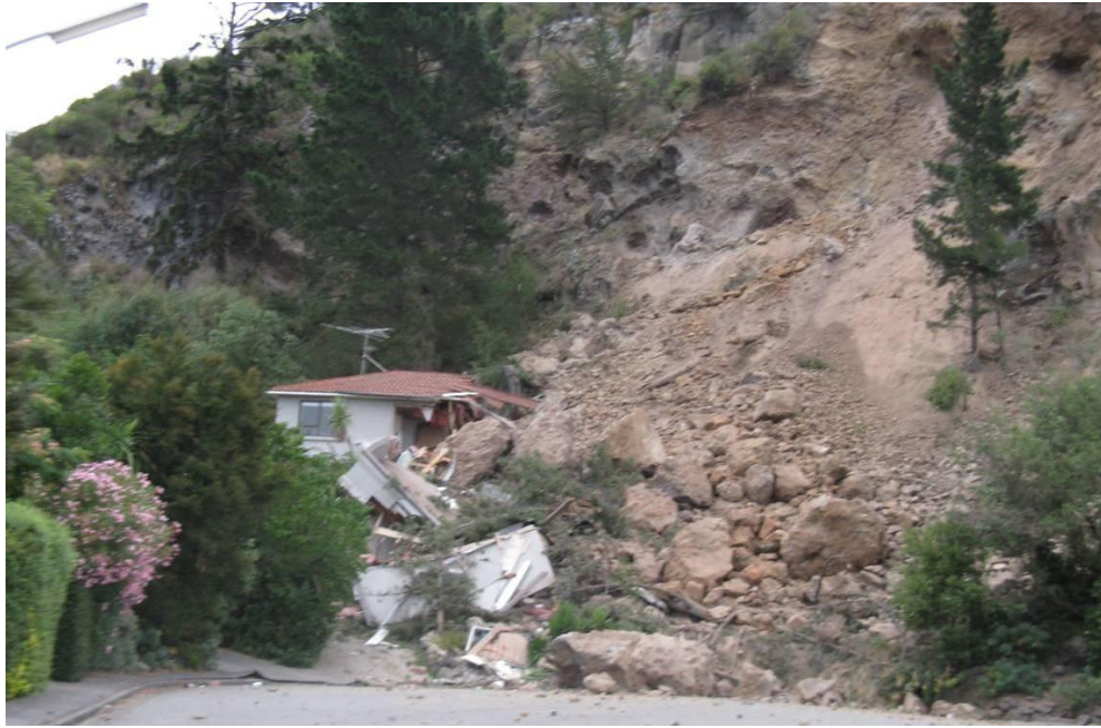
Figure 9-8. Home at the base of cliff in Redcliffs with wedge of talus boulders inundating the structure and roundabout, taken 22 Feb 2011. (-43.5610°, 172.7341°).
