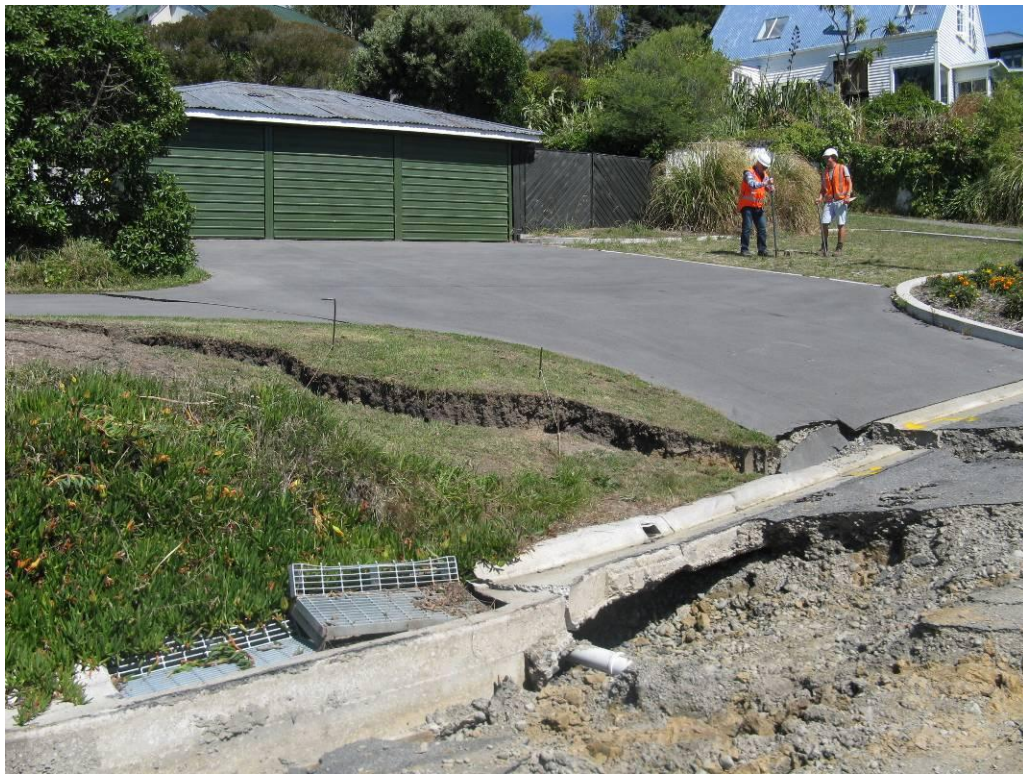
Figure 9-23. Landslide headscarp on Clifton Terrace with monitoring stakes. (-43.56543°, 172.75204°).
