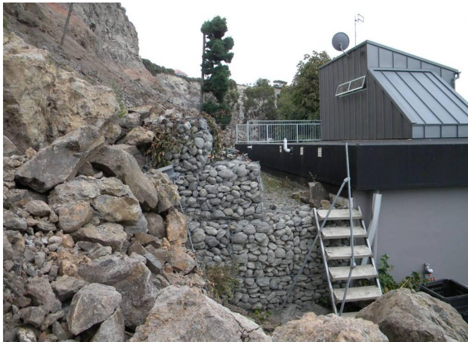
Figure 9-9. Photo showing the gabion behind house at base of cliff in the suburb of Redcliffs. No damage to house from rockfalls was observed (-43.56074°, 172.73379°).
