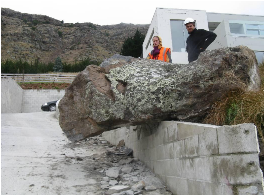
Figure 9-17. Boulder perched on driveway with source area above \sim 400 m away ( -43.58202^{\circ} , 172.7177^{\circ} ).
