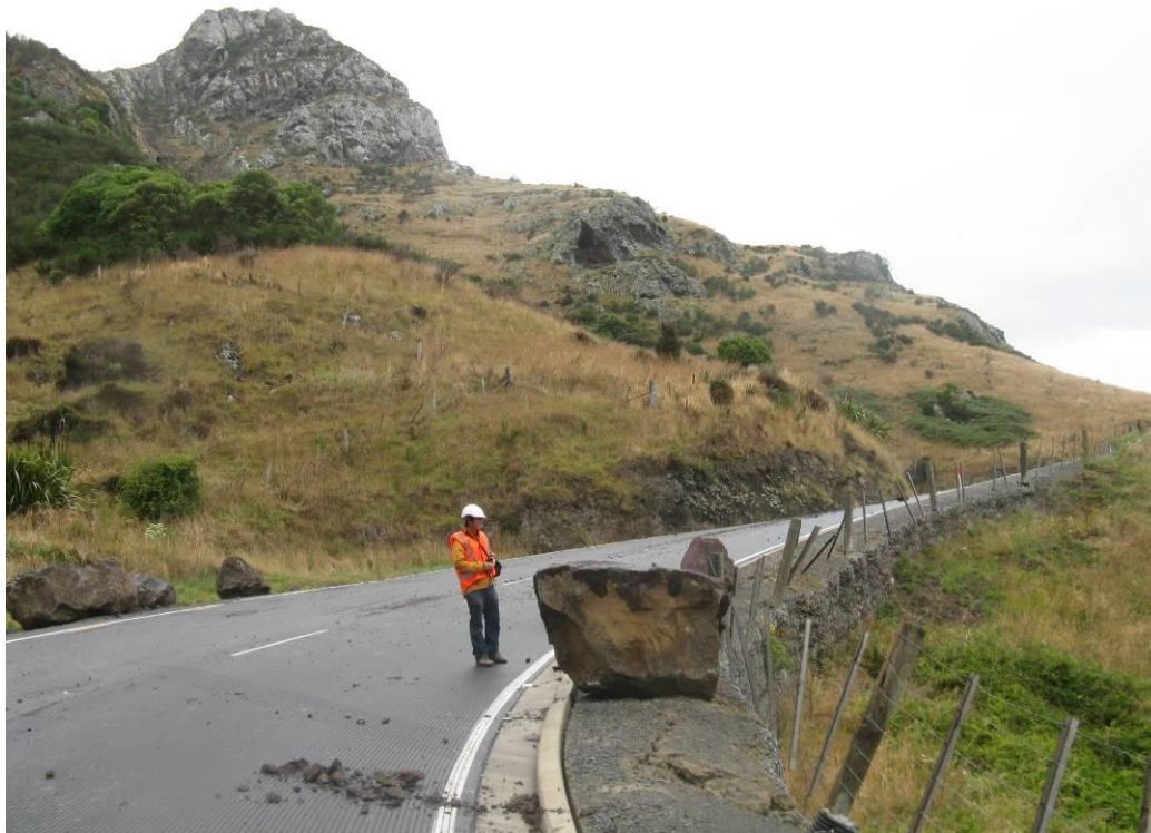
Figure 9-13. Rockfall along Evan's Pass Road, with columnar jointed source areas above road in background. (-43.6007°, 172.7354°).
