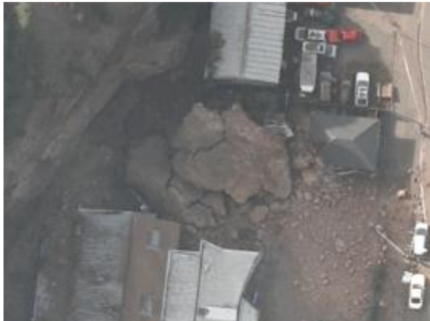
Figure 9-5. The Sumner RSA building was destroyed by a massive block that fell from the cliff-face (-43.5700°, 172.7586°). Top – Street view. Bottom – Aerial view (New Zealand Land Information Post-Earthquake Imagery)
