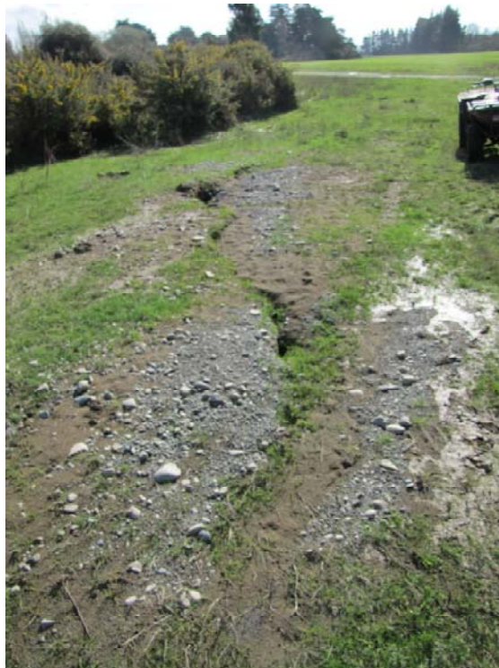
Figure 4.39 Material ejected from a fissure on the Selwyn Forks farm (front paddock). Note the gravel overlying the brown colored sand. This is what was visible after a night of rain. (Position marked as Photo 3 in Fig. 4.36.)
