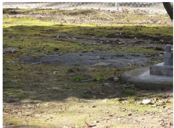
Figure 4.12 Evidence of limited/partial liquefaction in areas of Christchurch: (a) Evidence of liquefaction at Peterborough St - Madras St (CBD) ; (b) Sand boil in the foundation soils of a transmission tower (sub-station northeast of Greers Rd – Ruddenklau Ln, Bishopdale) (-43.4928055°, 172.5918055°).
