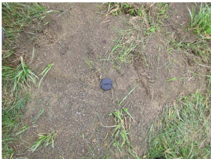
Figure 4.38 Liquefaction on the grass verge adjacent to the end of Gillanders Rd (Darfield side). Note the fine gravel particles on the surface and the fissure towards the top right hand side - it was possible to push the sampling spoon to a depth of about 300 mm into the fissure. (Position marked as Photo 2 in Fig. 4.36)
