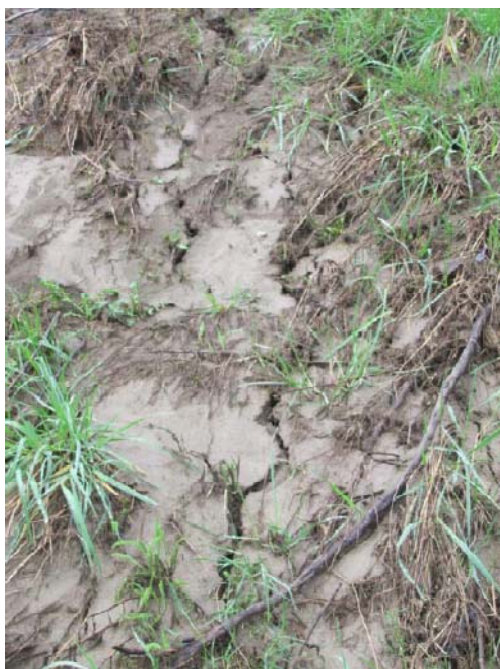
Figure 4.37 Ground damage adjacent to the bank of the Selwyn tributary near the end of Gillanders Rd (Darfield side). (Position marked as Photo 1 in Fig. 4.36; -43.596667^{\circ} , 172.080000^{\circ} )
