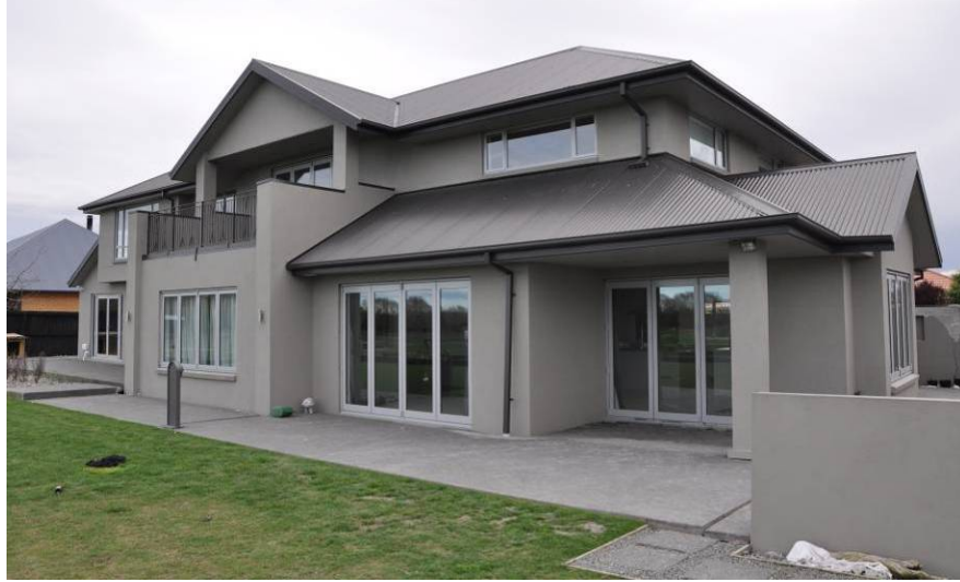
Figure 5.23 Damage to a residence along Courtenay Dr in the South Kaiapoi residential community. Backside of home facing Paddocks field articulates relatively no damage. (-43.391168°, 172.661894°; 1600 hrs on 11 September 2010)
