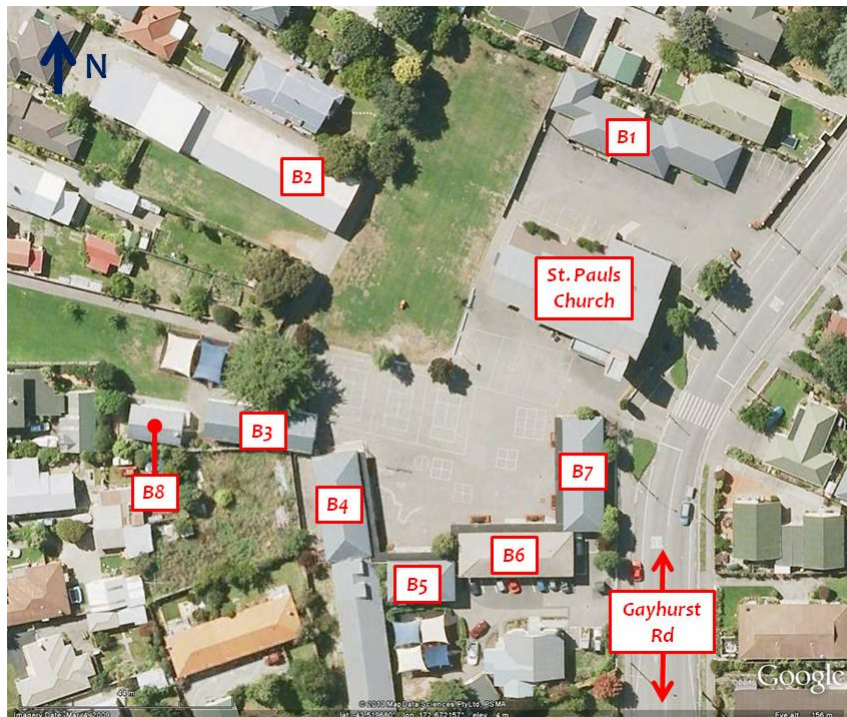
Figure 5.28 St Paul’s church and school in Dallington area (-43.5196°, 172.6725°). Notation “B#” is used for reference only to identify adjacent buildings (see discussion). The distance from the left to right edge of this image is ~0.17 km. (Annotated GoogleEarth image).
