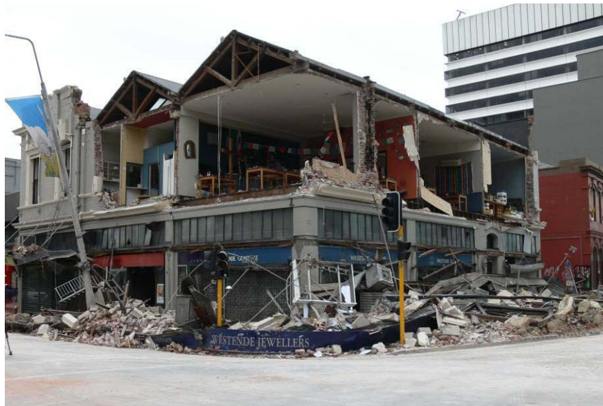
Figure 5.1 Structural collapse of a URM in the Christchurch Business District, 184 Manchester St. (Photograph courtesy of Prof Jason Ingham)
