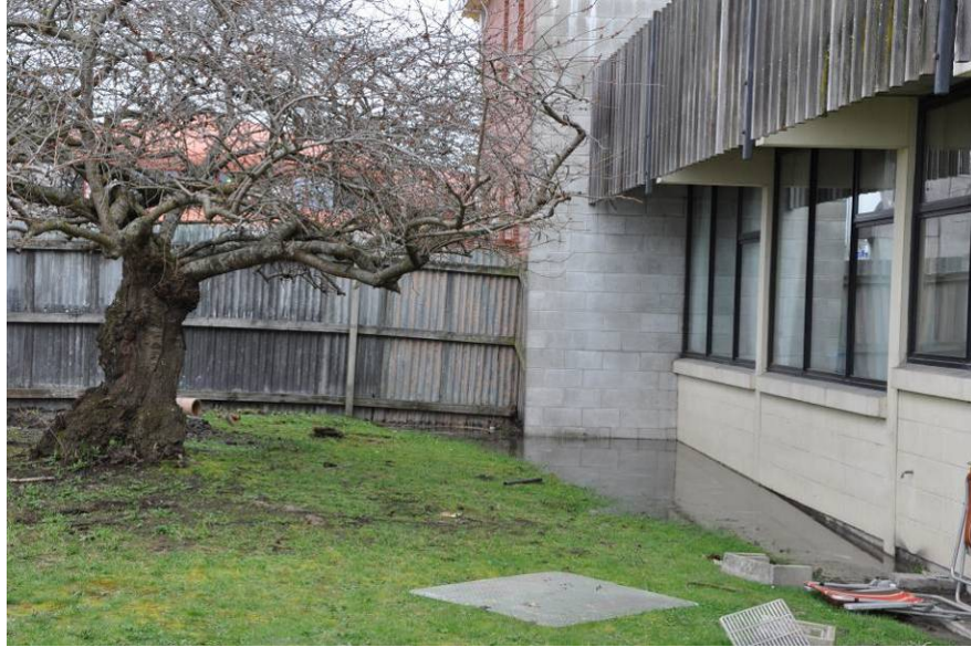
Figure 5.8 Property and Family Law Offices in Kaiapoi business district, 190 Williams St. View looking at west short axis end of the building (-43.3819°, 172.6591°; 1100 hrs on 11 September 2010)
