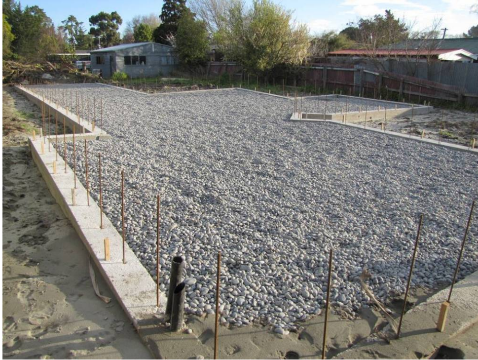
Figure 5.41. Site at Pines Beach which appears to be using the same slab-on-grade system as at Bexley (Chichester St; -43.3877°, 172.70304°; 1800hrs on 12 September 2010)
