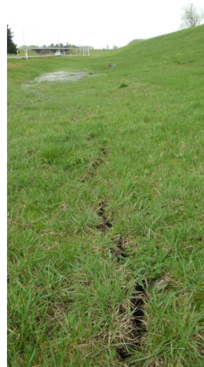
Figure 6.17 Photos 9 and 10: ~5-cm wide longitudinal cracks running along the crest (left) and base (right) of a secondary levee for the Waimakariri River. Photo taken looking southwest; SH1 on left of levee. The locations of these photographs are denoted in Figure 6.4. (-43.430108°, 172.643434°)
