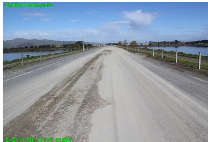
Figure 6.32 Repaired Dyers road that runs between Ponds 2A and 3. (-43.529933°, 172.715200°)
