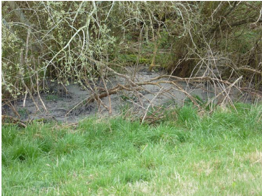
Figure 6.8 Photo 3: Liquefaction ejecta (center of photo) along the base of the levee on Coutts Island Rd (riverside). The location of this photograph is denoted in Figure 6.4. (-43.424093°, 172.630468°)
