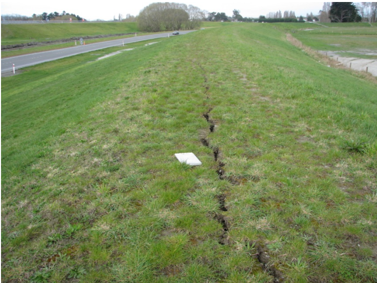
Figure 6.17 Photos 9 and 10: ~5-cm wide longitudinal cracks running along the crest (left) and base (right) of a secondary levee for the Waimakariri River. Photo taken looking southwest; SH1 on left of levee. The locations of these photographs are denoted in Figure 6.4. (-43.430108°, 172.643434°)
