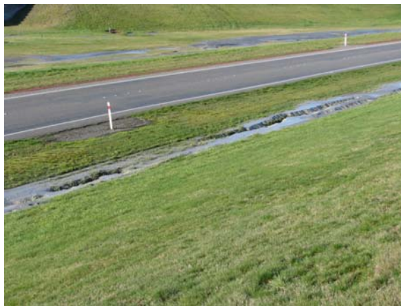
Figure 6.18 Photos 11 - 14: Liquefaction ejecta on both the river and landsides of the levee. The locations of these photographs are denoted in Figure 6.4. (-43.428968°, 172.645435°)
