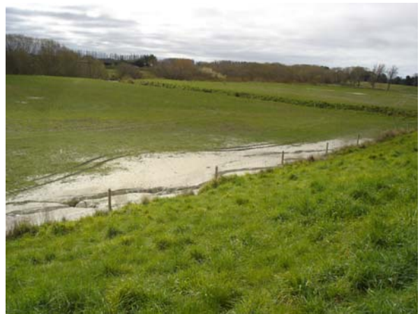
Figure 6.18 Photos 11 - 14: Liquefaction ejecta on both the river and landsides of the levee. The locations of these photographs are denoted in Figure 6.4. (-43.428968°, 172.645435°)
