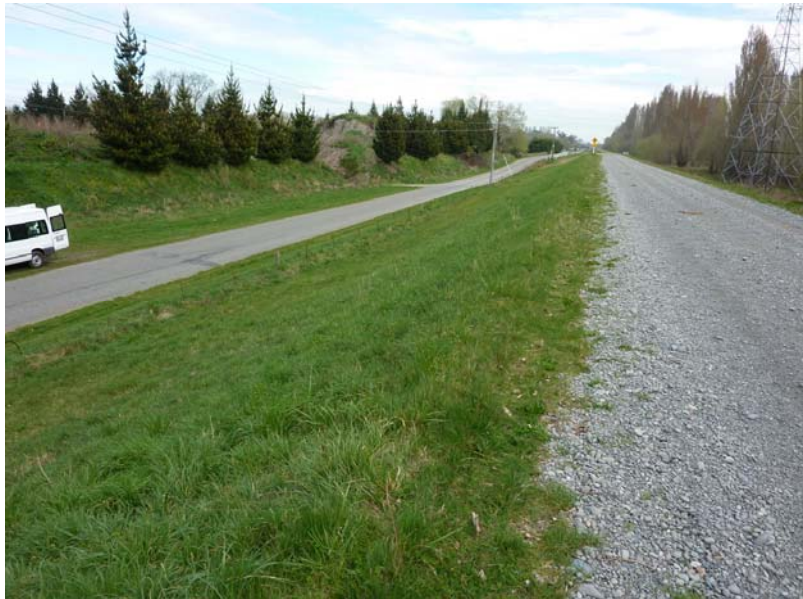
Figure 6.11 Photo 6: Stretch of levee without evidence of liquefaction. In the distance, a small rise can be seen in the road. This rise is the start of the ~0.5 km stretch where liquefaction was observed along the base of the levee. The location of this photograph is denoted in Figure 6.4. (-43.4225°, 172.6350°)
