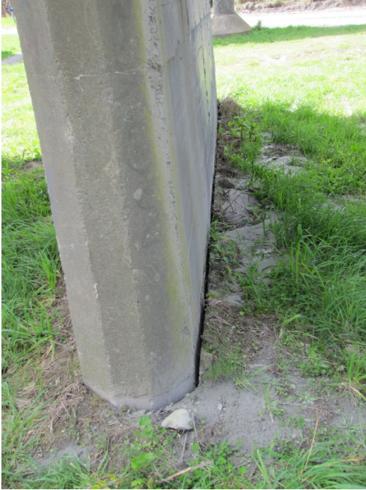
Figure 7.29 Evidence of liquefaction at Highway 1 bridge piers on the north side of the Waimakariri River. (-43.4153°, 172.6467°)
