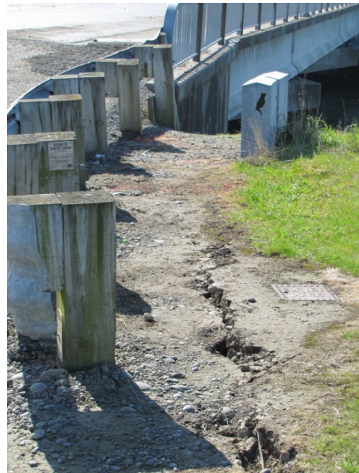
Figure 7.2 Cracking on margins of west approach embankment, Bridge Street Bridge. (-43.5253°, 172.7242°)
