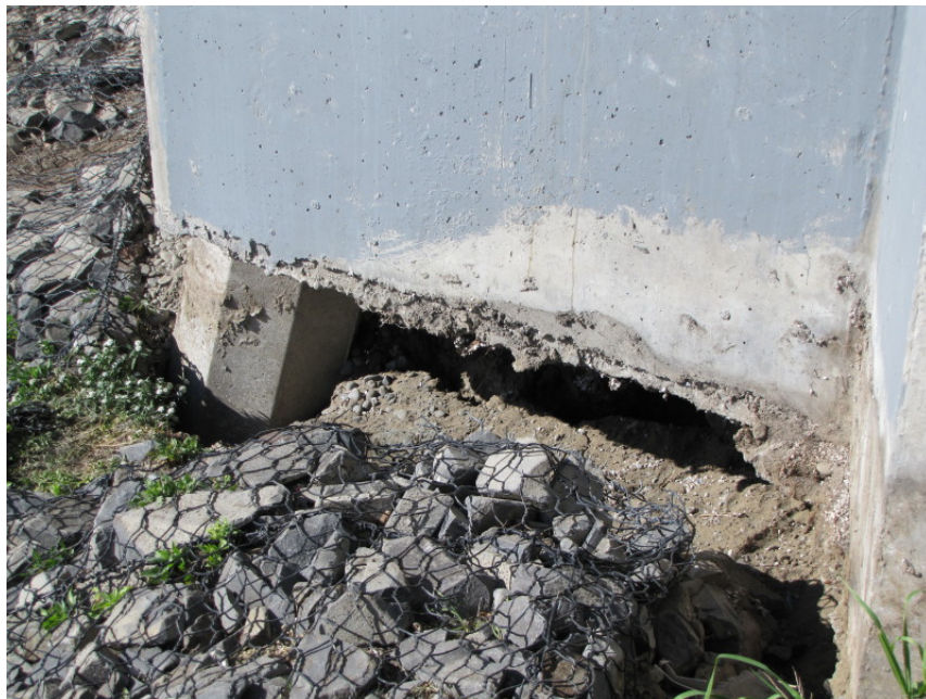
Figure 7.6 West abutment battered pile, Bridge Street Bridge. (-43.5253°, 172.7242°)
