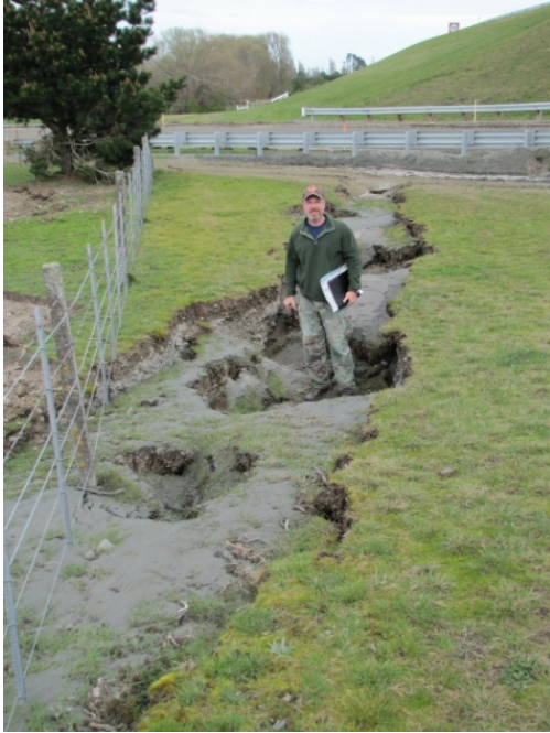
Figure 7.25 Evidence of liquefaction adjacent to Chaney's Overpass. (-43.4300°, 172.6464°)
