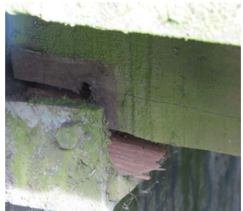
Figure 7.16 Footbridge on the Avon River near Medway Road: (a) Buckled span; and (b) Sheared bearing on east bank. (-43.5310°, 172.6656°)
