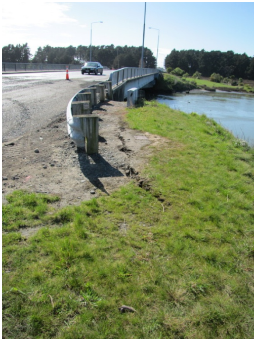
Figure 7.2 Cracking on margins of west approach embankment, Bridge Street Bridge. (-43.5253°, 172.7242°)
