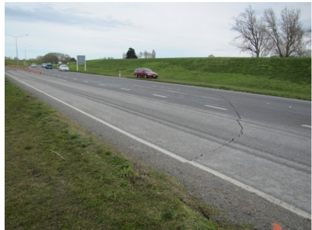
Figure 7.26 Cracking in and along roadway adjacent to Chaney's Overpass. (-43.4300°, 172.6464°)
