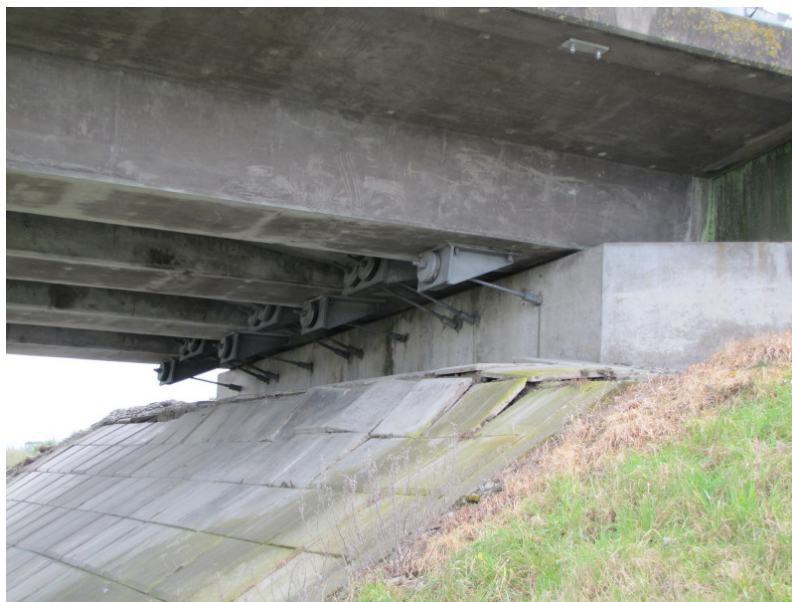
Figure 7.22 Cable Restrainers at north abutment, Chaney's Overpass. (-43.4300°, 172.6464°)
