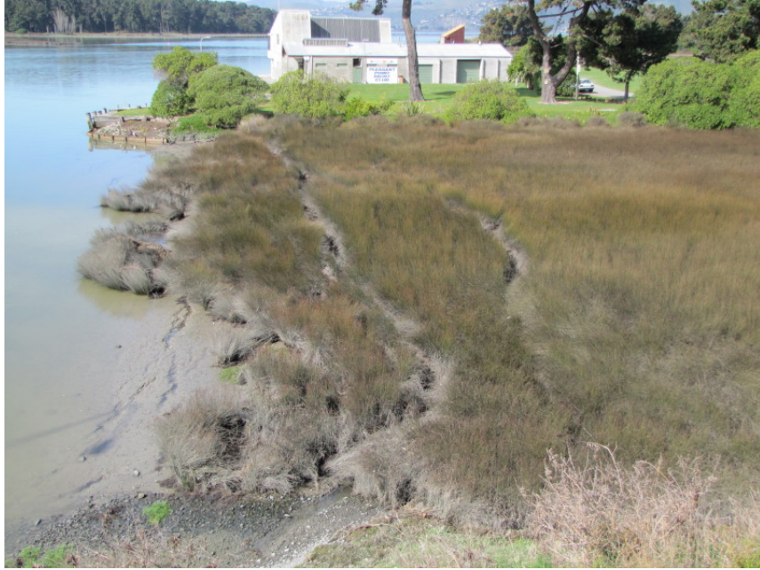
Figure 7.7 Lateral spreading on west bank, Bridge Street Bridge. (-43.5253°, 172.7242°)
