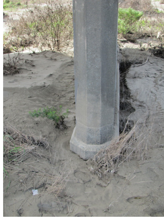
Figure 7.29 Evidence of liquefaction at Highway 1 bridge piers on the north side of the Waimakariri River. (-43.4153°, 172.6467°)
