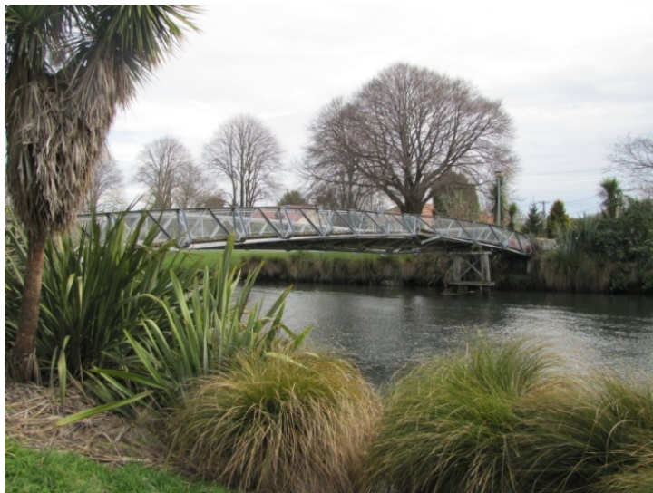
Figure 7.16 Footbridge on the Avon River near Medway Road: (a) Buckled span; and (b) Sheared bearing on east bank. (-43.5310°, 172.6656°)
