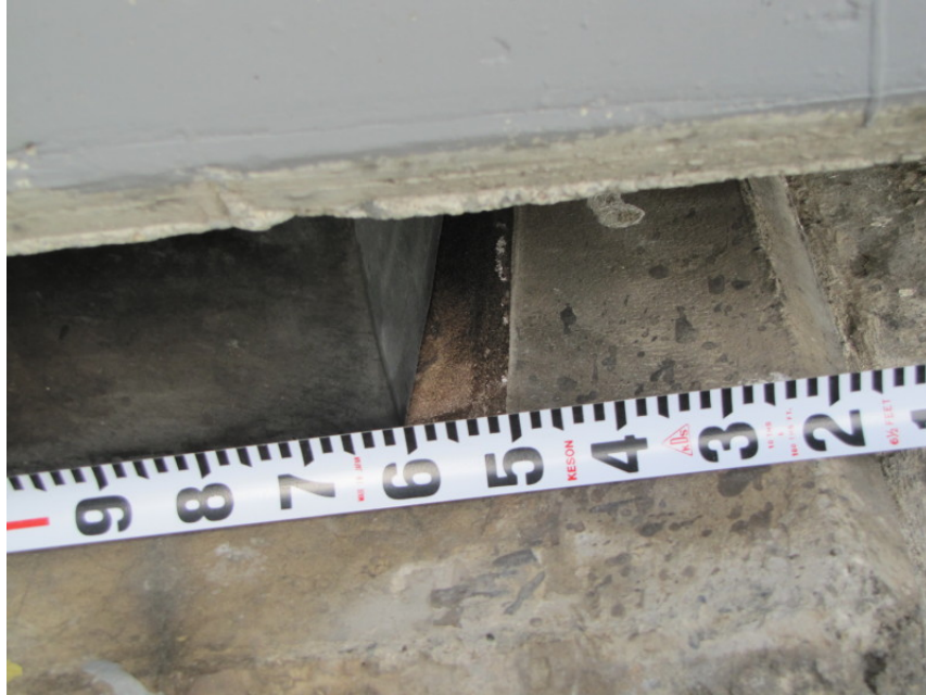
Figure 7.5 West abutment bearing pad displacement, Bridge Street Bridge (scale in Inches). (-43.5253°, 172.7242°)
