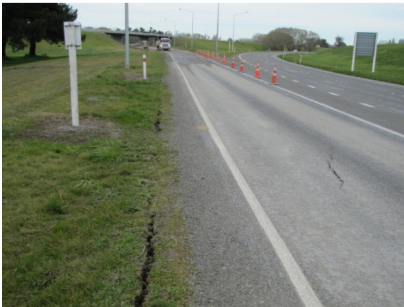
Figure 7.26 Cracking in and along roadway adjacent to Chaney's Overpass. (-43.4300°, 172.6464°)
