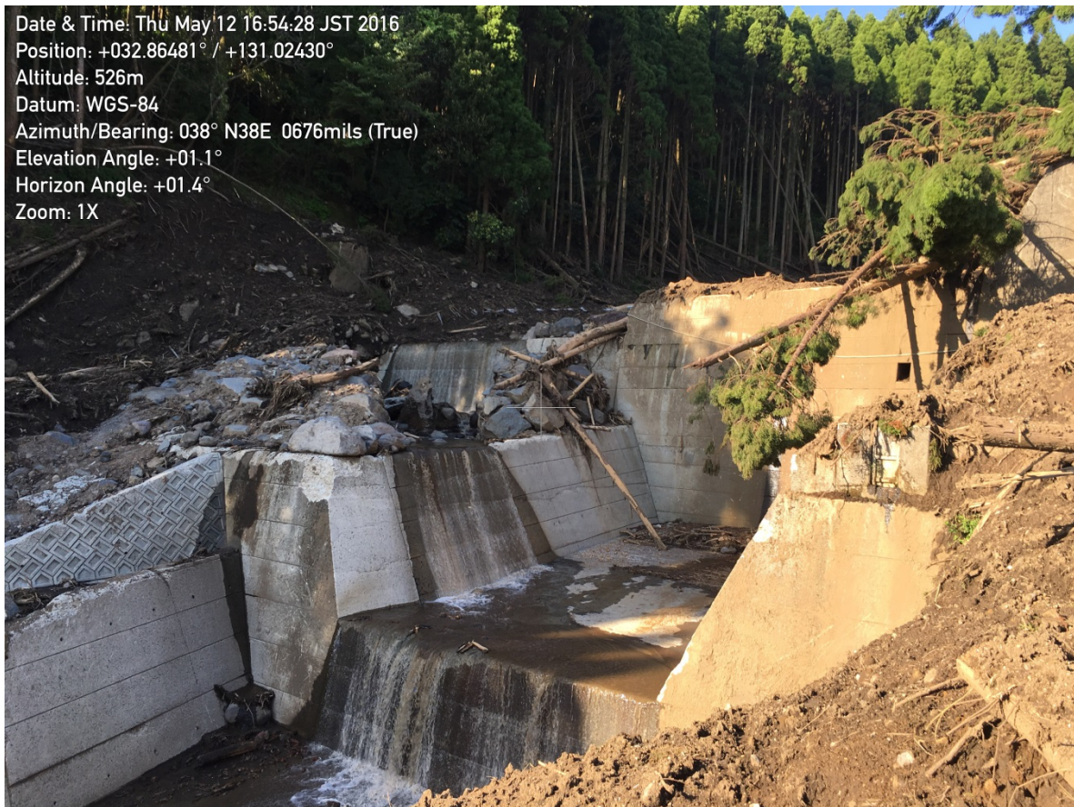
Figure 5-11. Close up of the dam. Note the right side of the dam is missing, in contrast to the left side which is intact.
