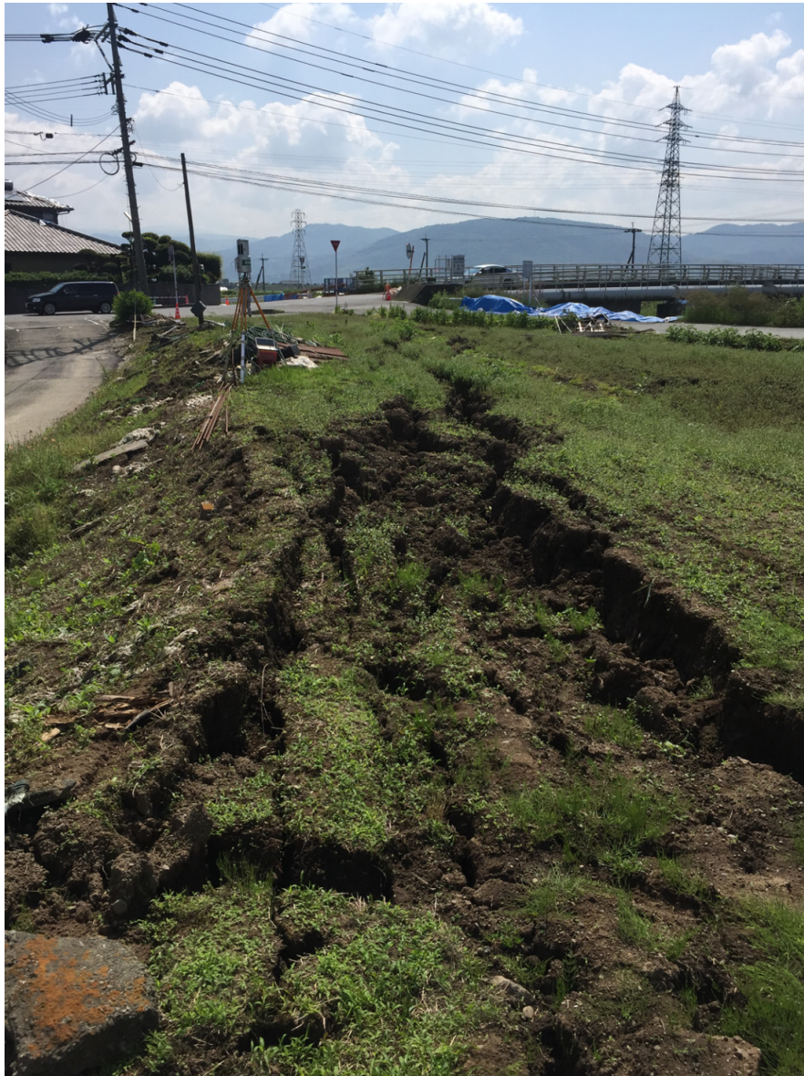
Figure 6-15. Section of lateral spread relative to location of LIDAR setup and pipeline bridge (32.77369° N 130.78384° E).
