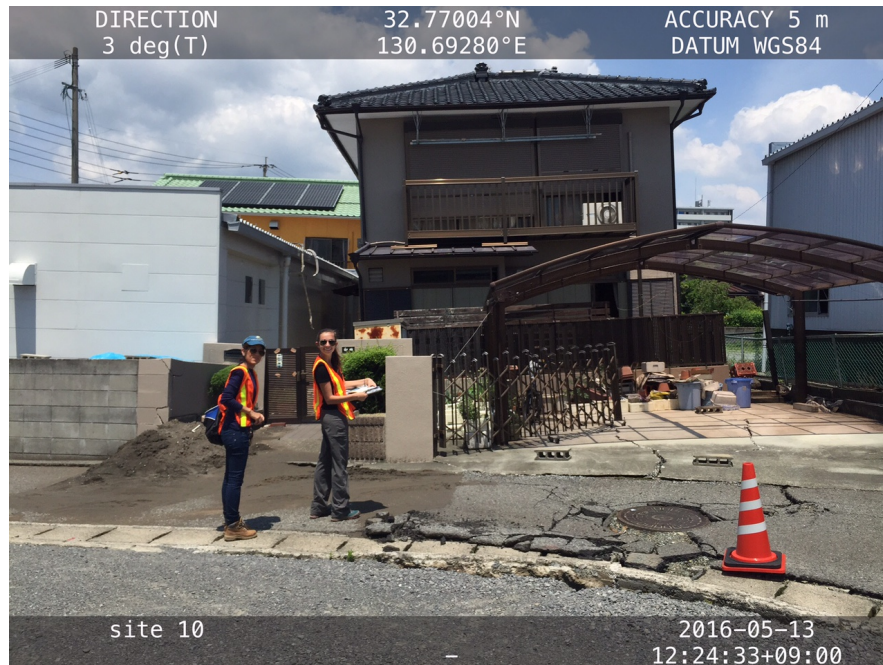
Figure 6-13. Picture of building settlement and tilt due to soil liquefaction in the south-east corner of the Shirakawa River. Building settlement with respect to the surrounding ground in the order of 10 cm and tilt of 2 degrees.
