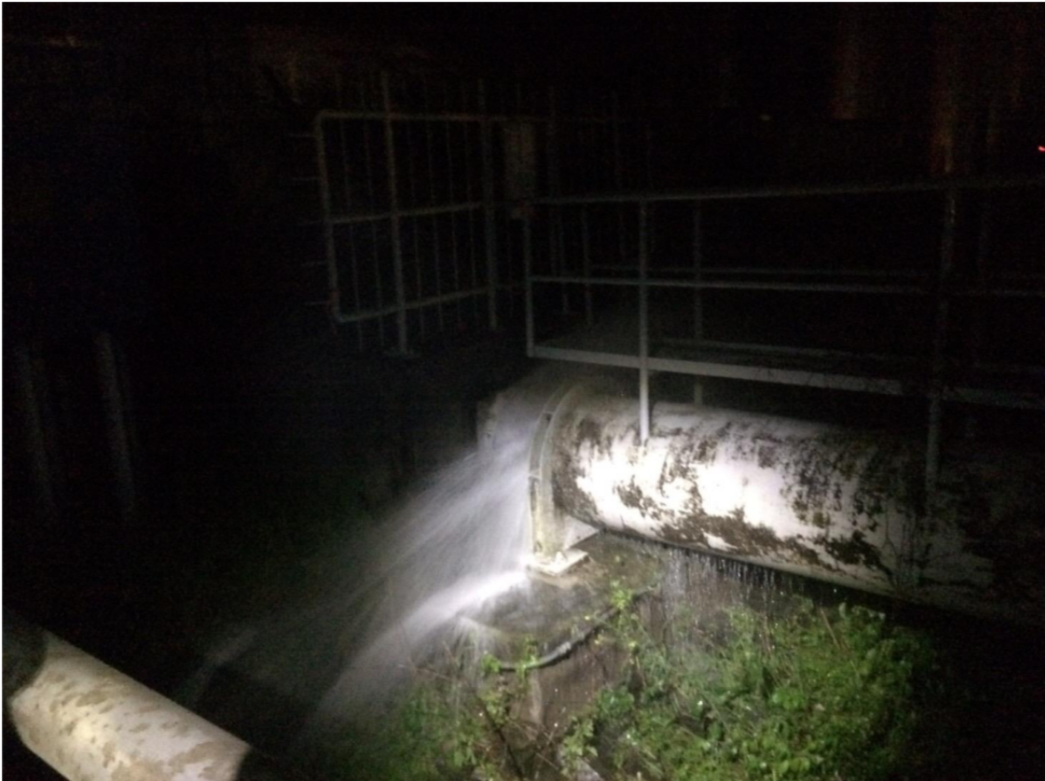
Figure 7-3. Leakage of 800 mm diameter bridge pipeline (courtesy of Kumamoto City Water and Sewer Bureau) (32.77326, 130.78428).
