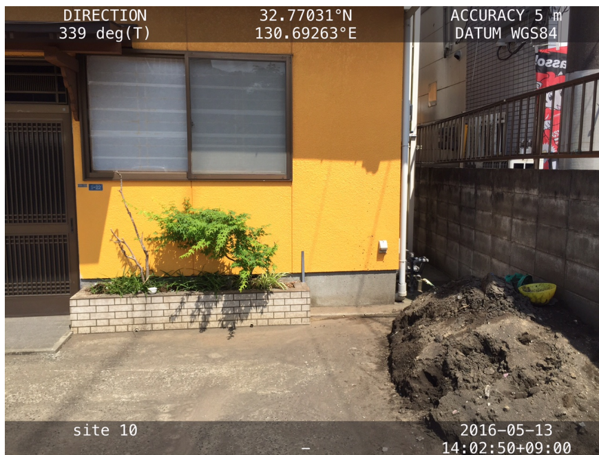
Figure 6-12. Picture of building with no damage but evidence of sand boil in the south-east corner of the Shirakawa River. Building settlement in the order of 5 cm and tilt 1 to 3 degrees.
