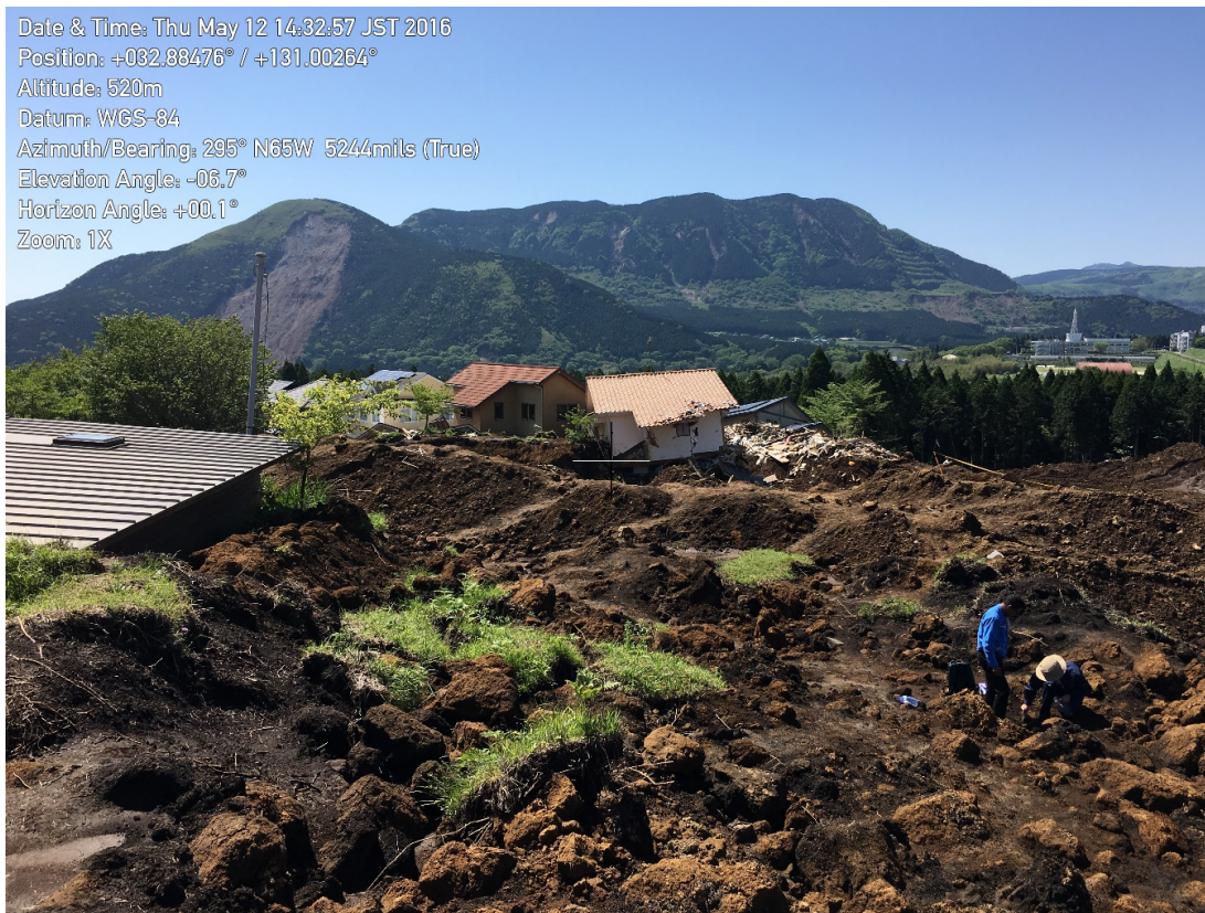
Figure 5-5. Damage to a residential area as a result of the landslide runout. Several structures are missing that would have previously fit within the frame of the photo.
