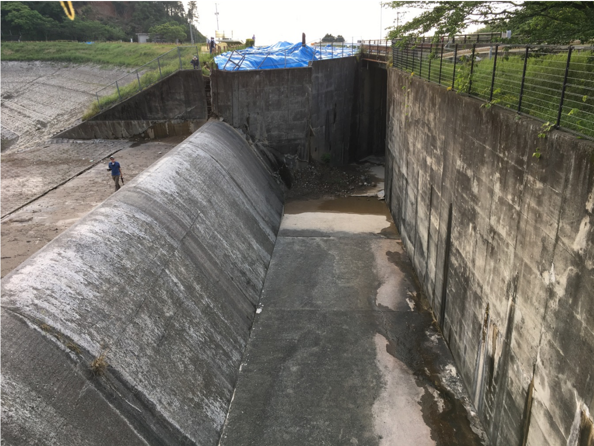
Figure 9-9. Overview of the condition of the spillway.
