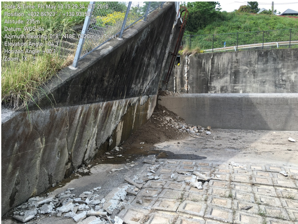
Figure 9-17. A close up of the left spillway training wall.
