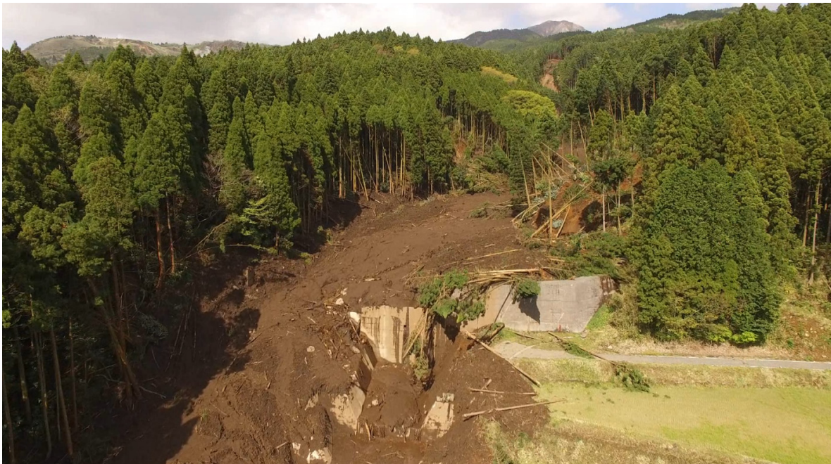
Figure 5-13. Still image from UAV video footage produced by the Geospatial Information Authority of Japan (GSI, 2016), showing the upstream condition of the dam and the sediment flow, soon after the earthquake.
