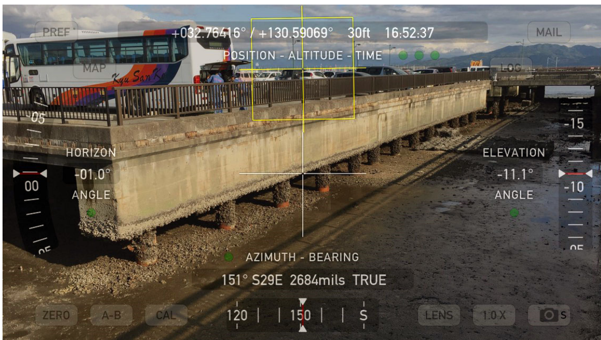
Figure 6-4. Volumetric reconsolidation in native silt apparent from the estimated 25 cm of newly-exposed red steel at the base of the piles supporting the pier.
