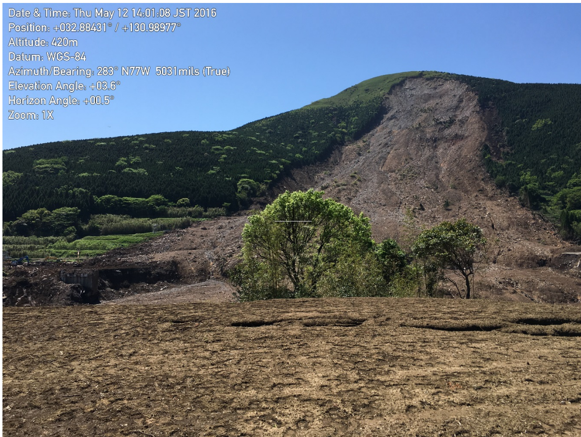
Figure 5-3. Front view of the Great Aso Landslide that likely destroyed a bridge, the remnant abutment of which is visible on the left side of the photo. The nearby fault displacement may have also contributed to the bridge collapse.
