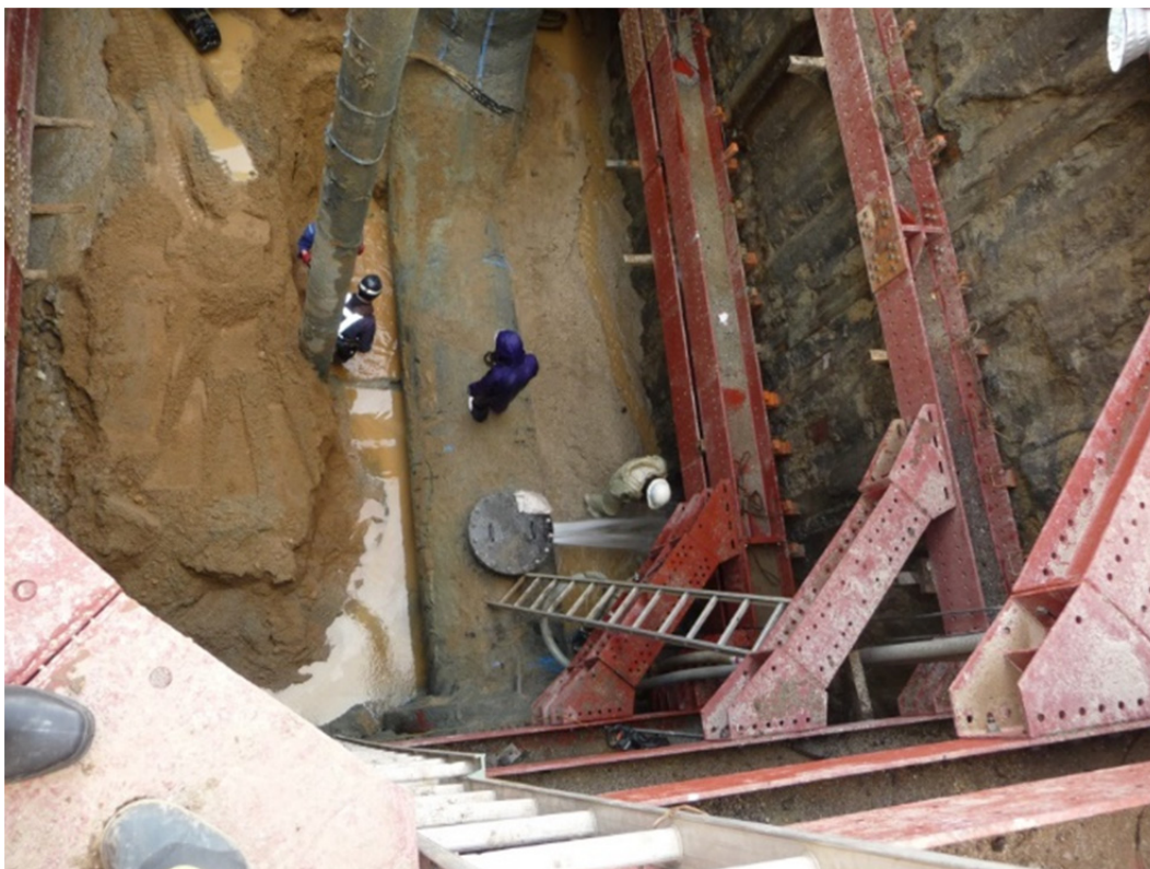
Figure 7-4. Repair of a 1350 mm transmission main with leakage from 600 mm flange cap (courtesy of Kubota Corp) (32.76382, 130.75117).
