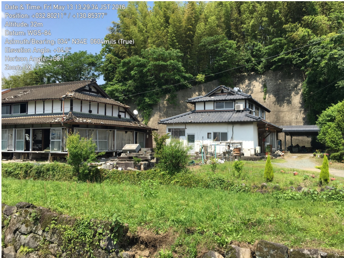
Figure 4-13. Right-lateral offset along the Futagawa Fault likely passed through the large retaining wall behind the residential structures and into the hill behind it; however, we were not able to examine the wall up close and the bamboo jungle behind the wall was too dense to traverse. No visible damage in the retaining wall could be seen from our vantage point.
