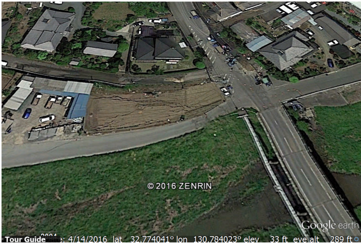
Figure 6-14. Lateral spread feature identified adjacent to a bridge.
