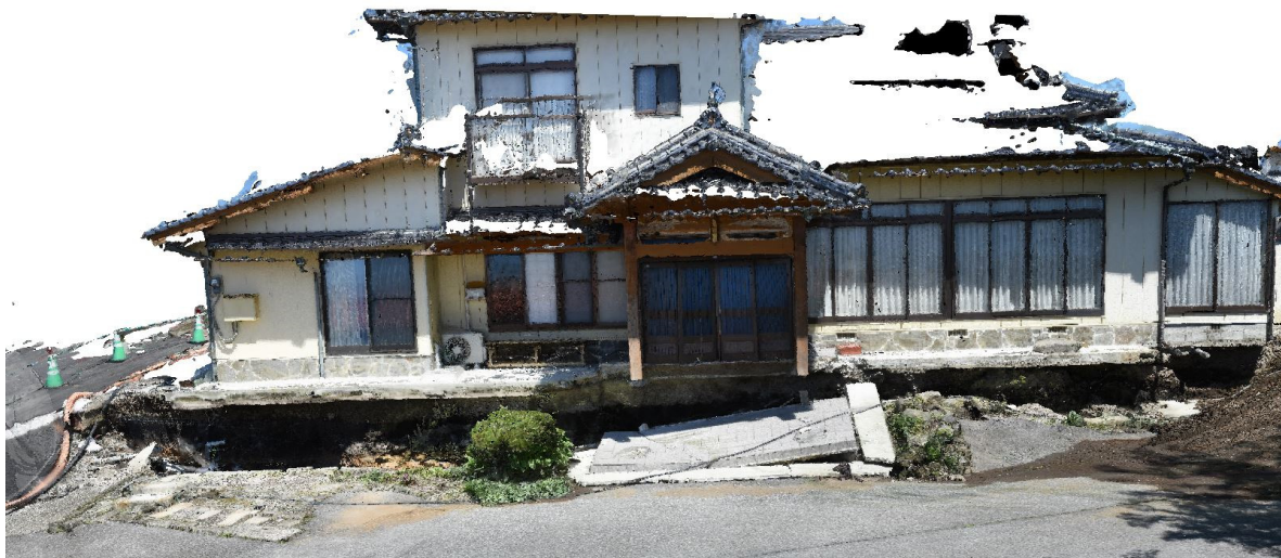
Figure 9-42. Screenshot of a 3D textured model of a house damaged by the depression zone. The model was developed from approximately 50 digital photographs captured with a Nikon D7100 DSLR camera ( 32.95663^{\circ} N 131.03670^{\circ} E).
