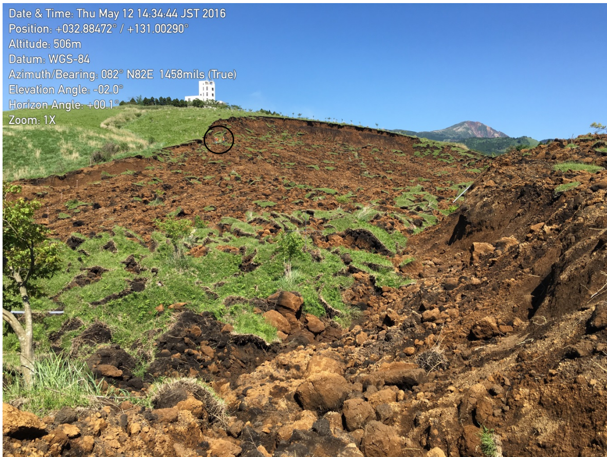
Figure 5-4. The landslide source area, upslope of the residential structures. Note the people in orange on the left side of the slide for scale.
