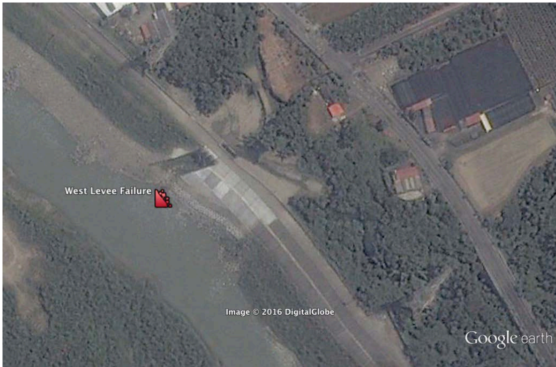
Figure 8-22: Google Image of region where Failure 2 occurred (image date: 8/2014).
