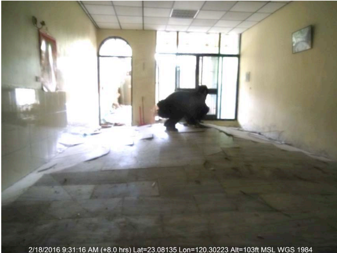
Figure 7-28: Heaving of Unreinforced Interior Slab ( 23.08135, 120.30233 ).
