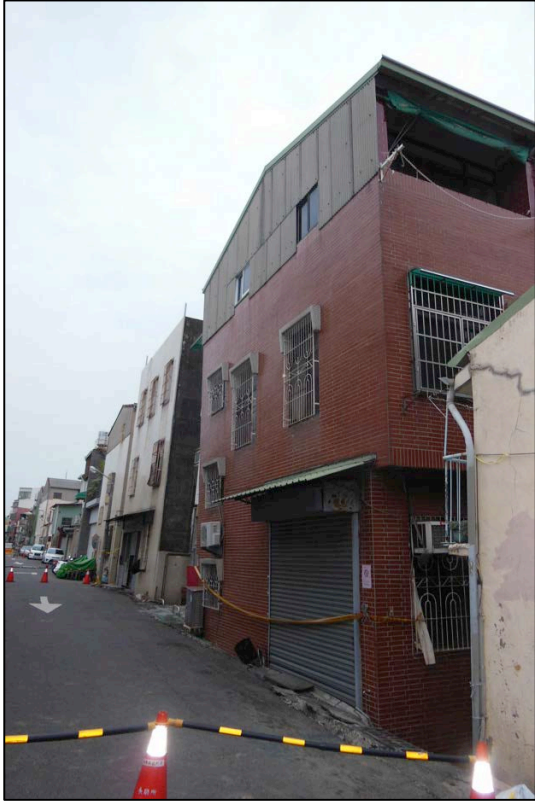
Figure 7-17: Severely tilted building in Wenhe Street and adjacent alley with significant expression of hardscape liquefaction features ( 23°00'12.7"N 120°11'30.5"E ).
