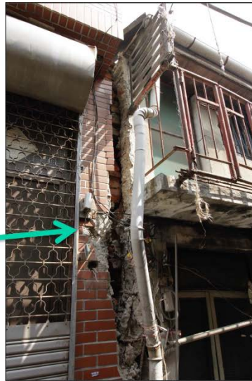
Figure 7-18: Approximately orthogonal perspective and local view (left and right respectively) of the damaged building shown in Figure 7-17; note the well delineated structural hinge that developed along the brick-concrete interface of the right image (older portion of structure on right). The green denotes that the image on the right is taken behind the building. (23.003471°,
