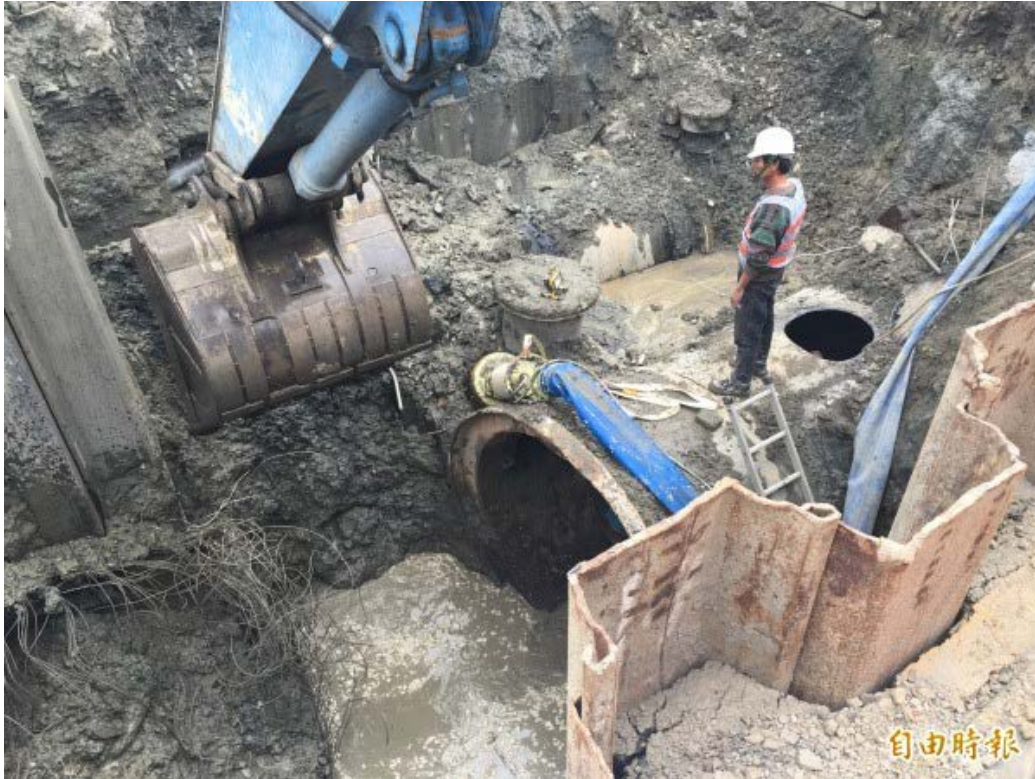
Figure 6-5: Repair of Damage Water Main (image Courtesy of Liberty Times) (23.005214, 120.261222).
