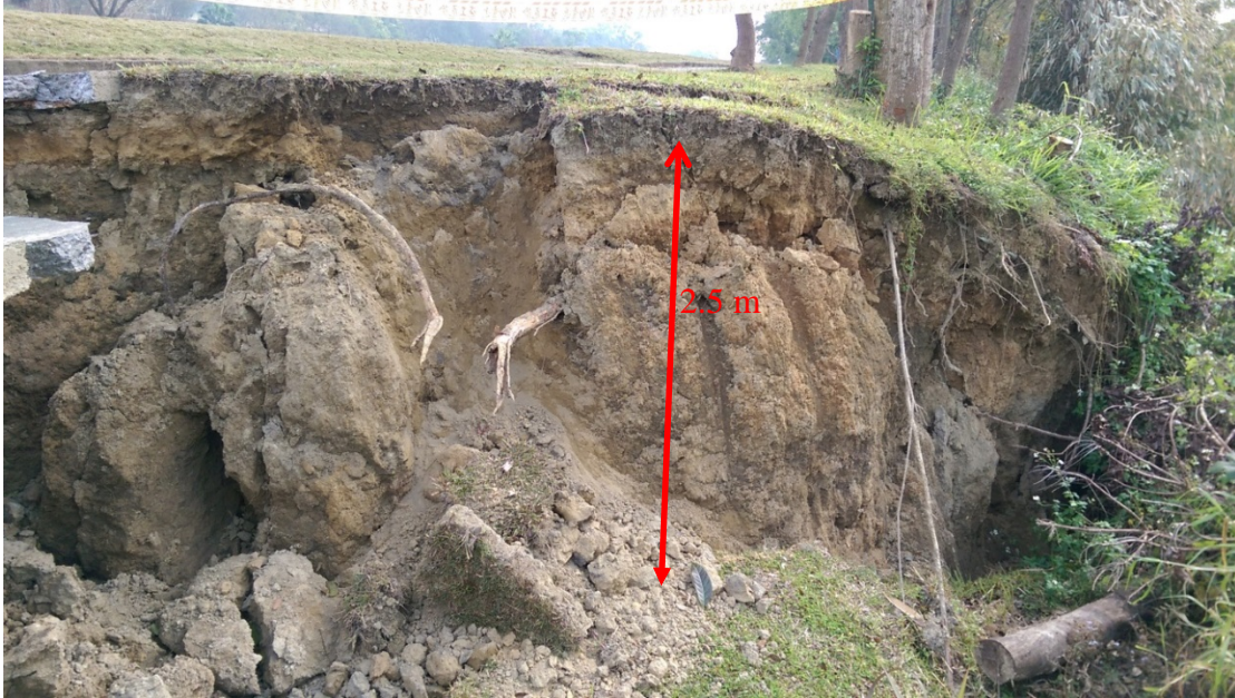
Figure 8-41: Maximum vertical drop at the south end of the Nanboa golf course (23.151721, 120.370245)
