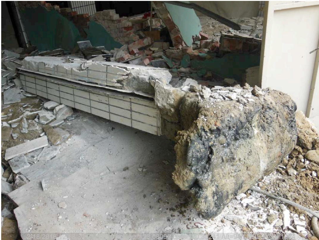
Figure 7-26: Structural column at the interior of a garage, note the lack of foundation support ( 23.08096 , 120.30258 ).
