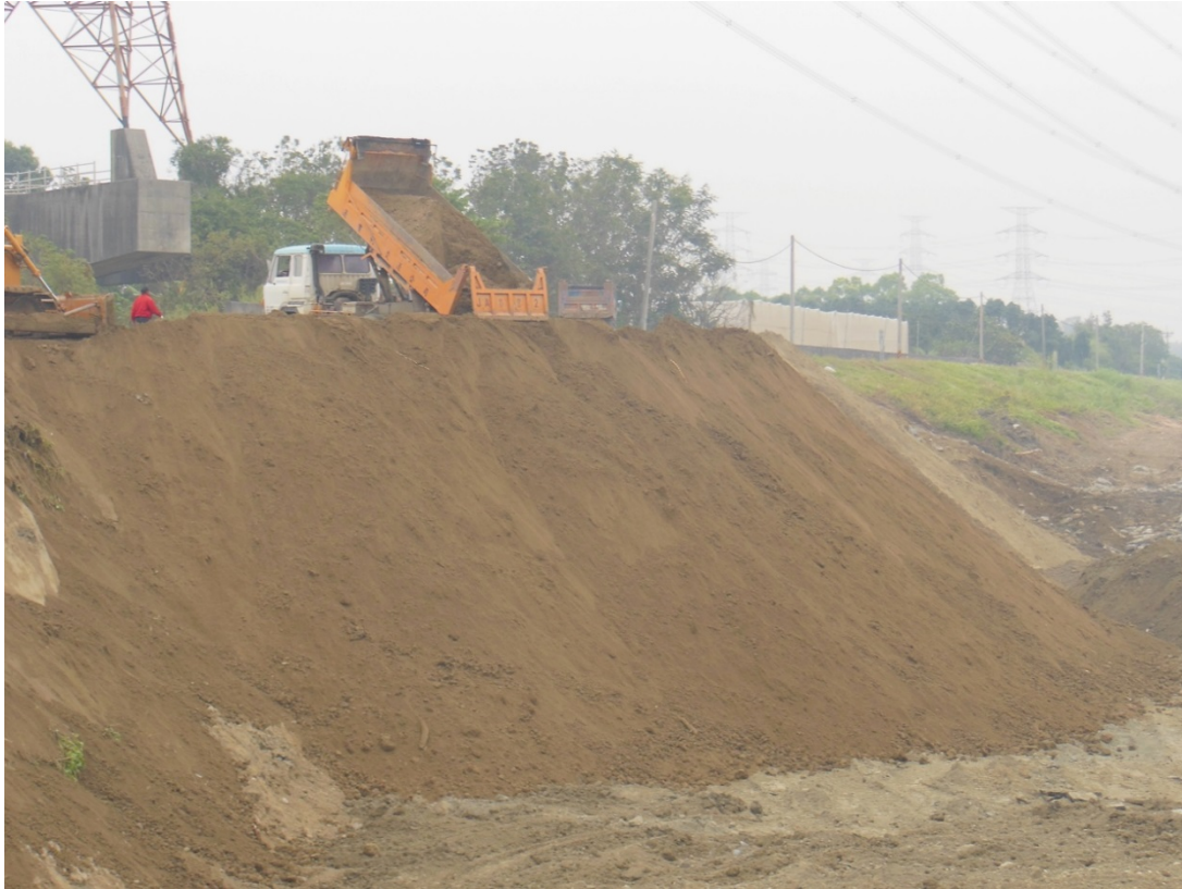
Figure 8-24: Emergency Backfill of the Levee (at Failure 2) (23.150949, 120.346590).
