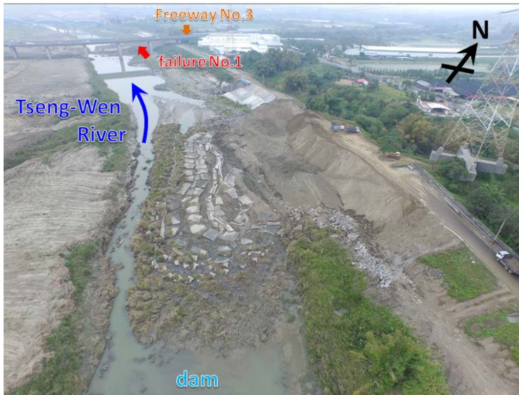
Figure 8-15: Bird's View of failure No.2. (Photo: W.-K. Huang) ( 23^{\circ} 9'3.26'' , 120^{\circ}20'47.59'' ).
