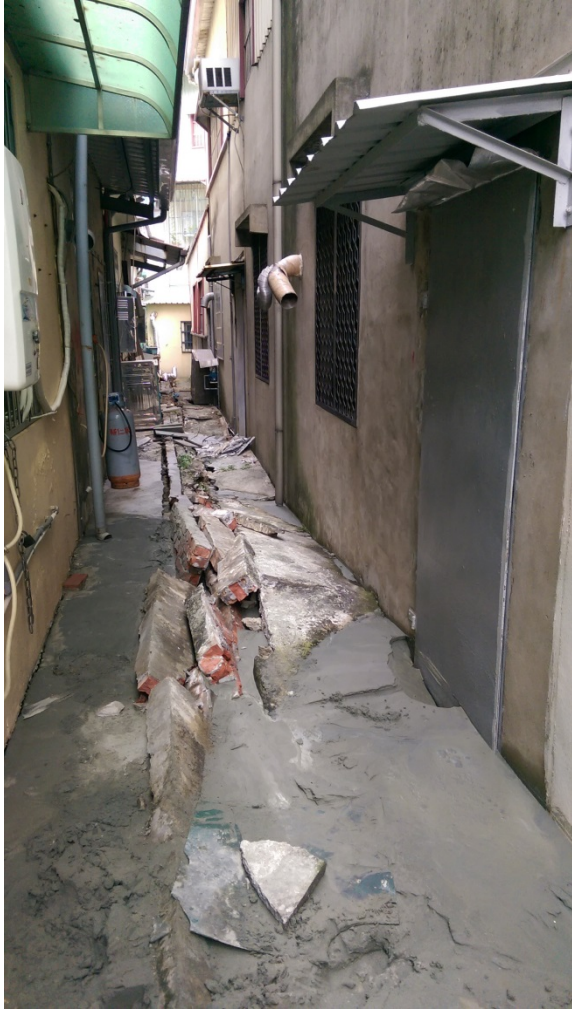
Figure 7-22: Damage to buildings at the Xinshi site (left: fire lane with expressed surface manifestation and building settlement and right: garage expressing significant hardscape damage).
