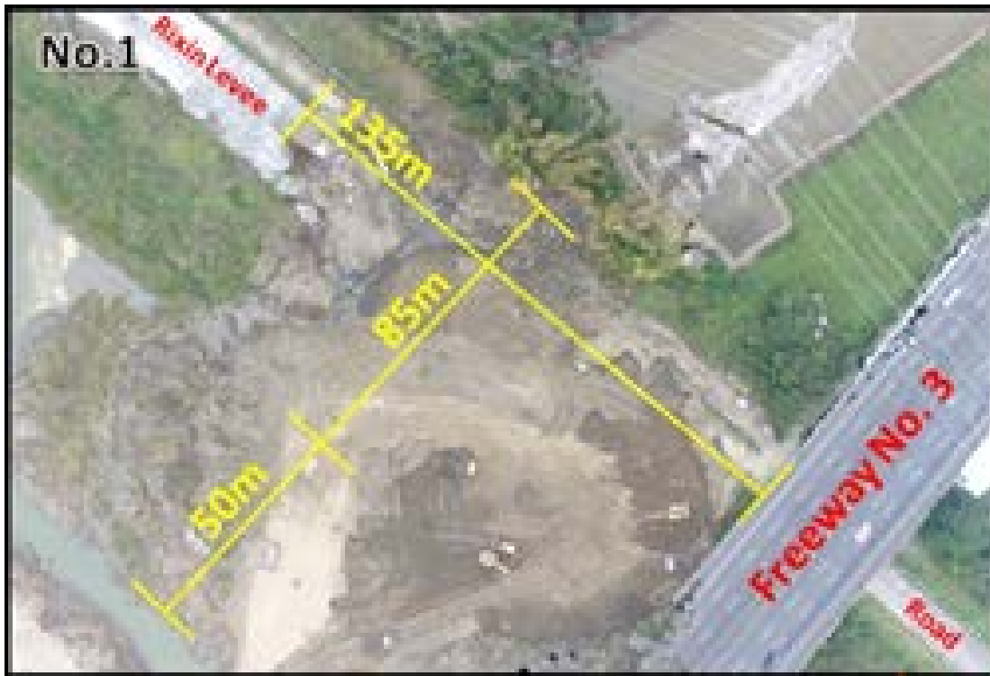
Figure 8-5: Layout of Failure No. 1 (23° 9'12.40", 120°20'37.68").
