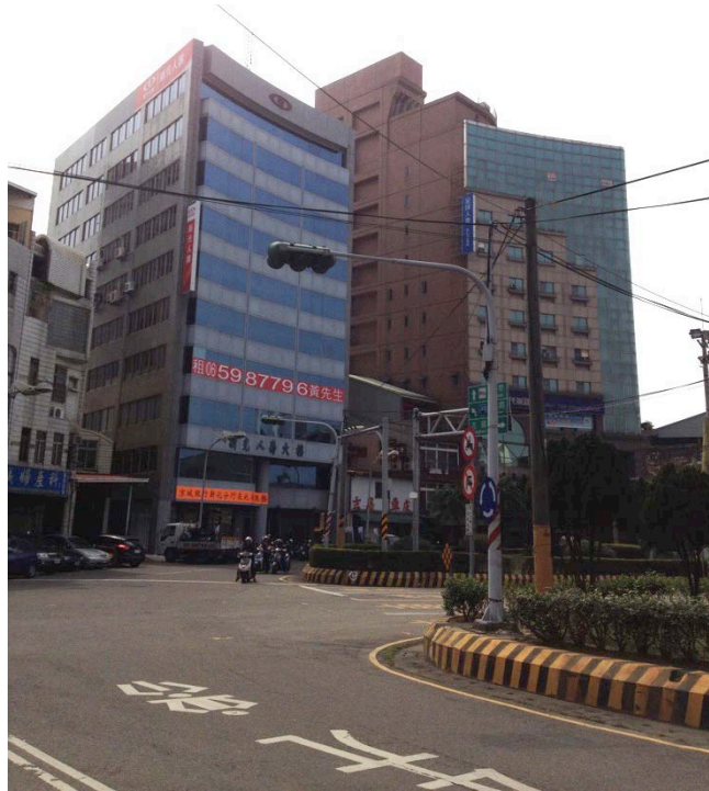
Figure 5-12: Pair of 10 and 12 story buildings about 100m from the King's Town Bank (23.0363, 120.300) – the building on the right suffered minor damage. Both were operational after the earthquake.
