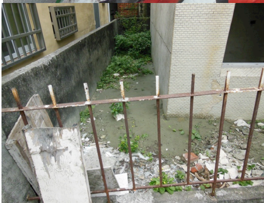
Figure 7-5: Liquefaction surface manifestation in the Annan District ( 23.025697 , 120.207138 ).
