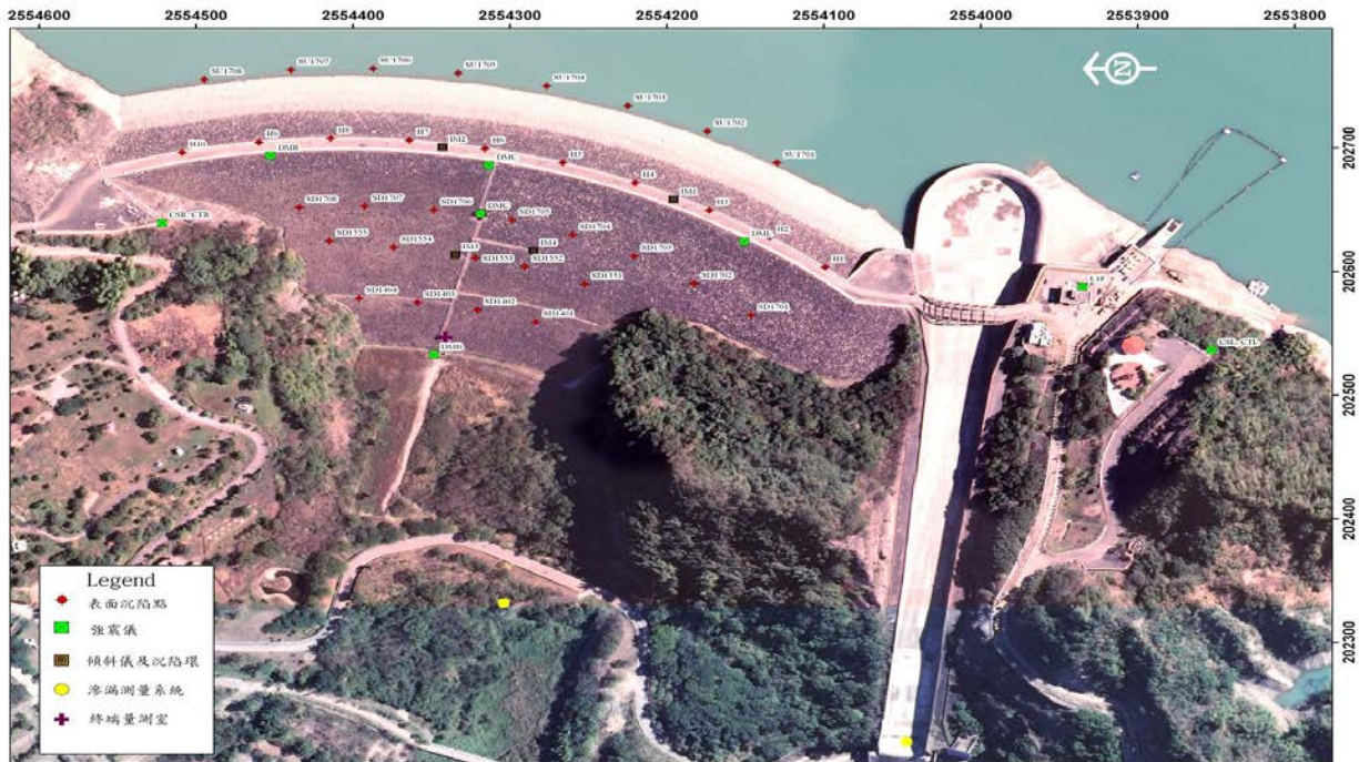
Figure 9-6: Aerial View of Nan Hwa Dam with Instrumentation Locations.
