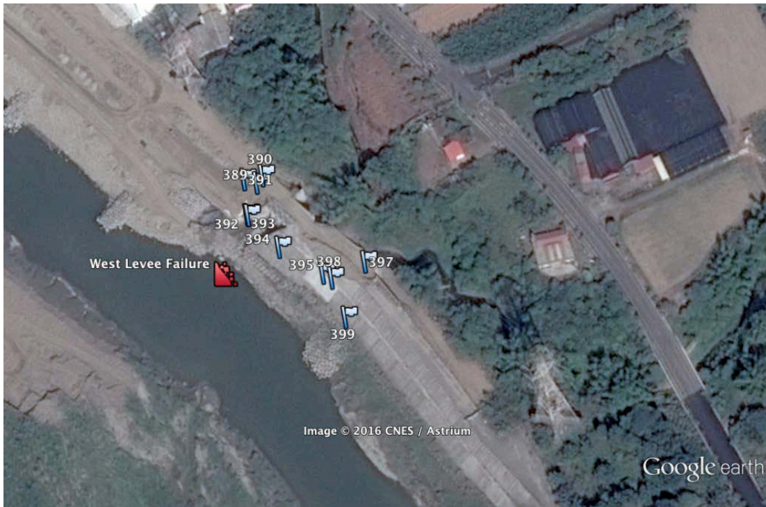
Figure 8-20: Google Image of region where Failure 2 occurred (image date: 2/2014).
