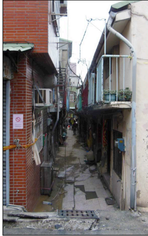
Figure 7-17: Severely tilted building in Wenhe Street and adjacent alley with significant expression of hardscape liquefaction features ( 23°00'12.7"N 120°11'30.5"E ).
