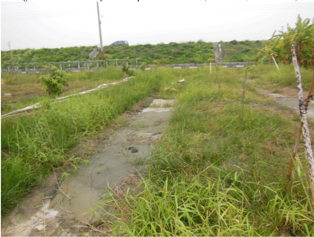
Figure 8-37: Evidence of Liquefaction on Land slide of Levee (23.120823, 120.378989).
