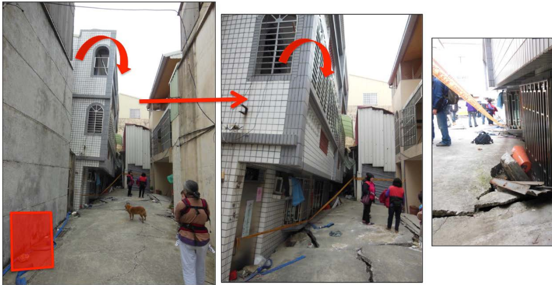
Figure 7-9: Example of mapping worse case ground and structural damage combination (GF3-DF5). ( 23.025442^\circ , 120.207400^\circ ; Lane 161, Hui'an St)
