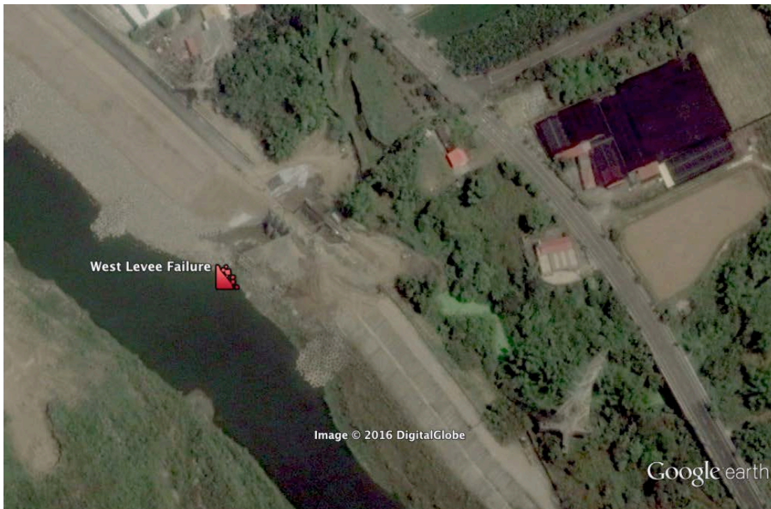
Figure 8-21: Google Image of region where Failure 2 occurred (image date: 5/2014) – note the visible constructed structural spillway.
