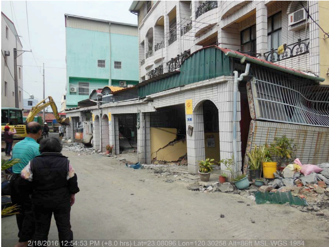
Figure 7-24 Damage to illegal add-on car port ( 23.08096, 120.30258 ).
