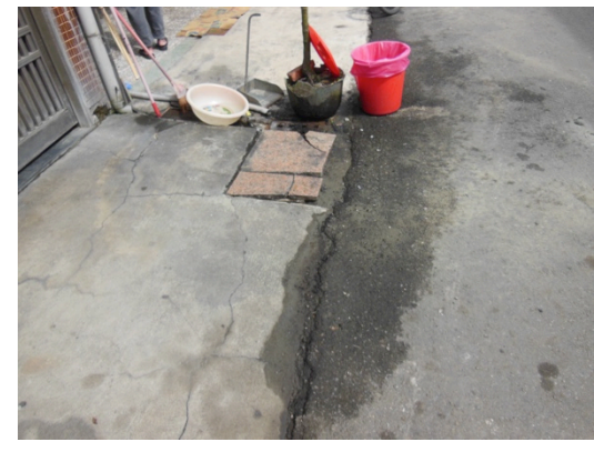
Figure 7-5: Liquefaction surface manifestation in the Annan District ( 23.025697 , 120.207138 ).
