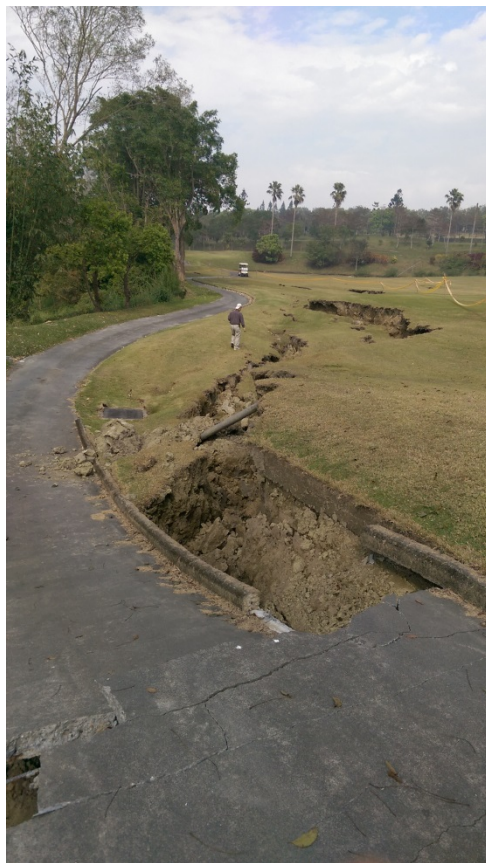
Figure 8-42: Surface rupture at the crest of sliding mass at Nanboa golf course (23.151721, 120.370245).
