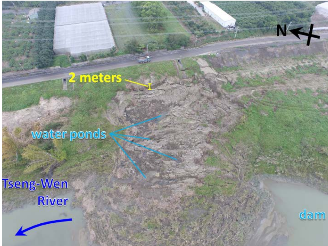
Figure 8-28 Bird's view of failure No.3. (Photo: W.-K. Huang). ( 23.148325, 120.347631)
