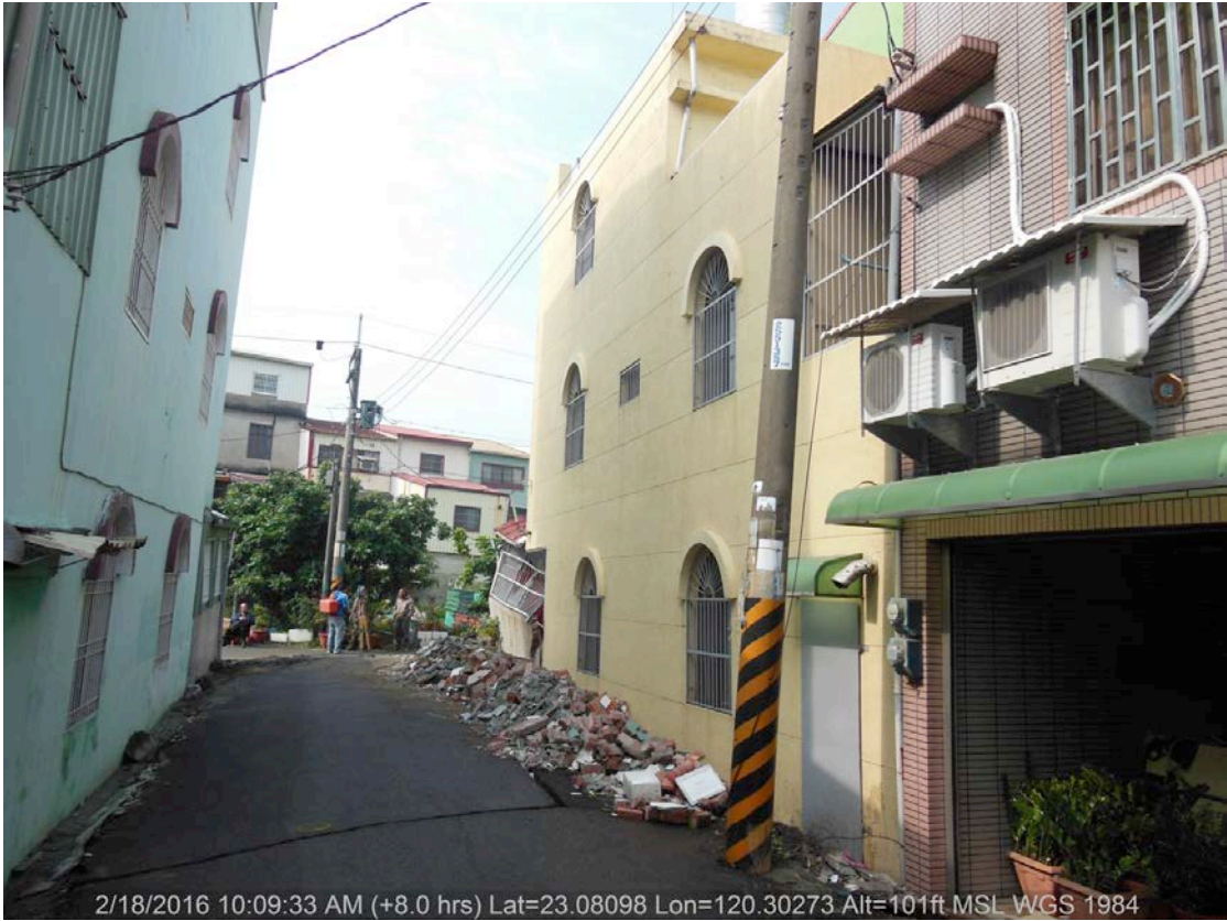
Figure 7-23: Ground heave along an alley between two settling buildings ( 23.08098, 120.30237 ).
