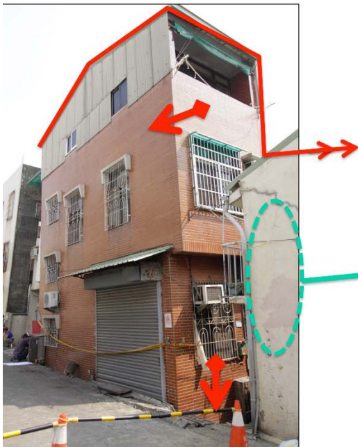
Figure 7-18: Approximately orthogonal perspective and local view (left and right respectively) of the damaged building shown in Figure 7-17; note the well delineated structural hinge that developed along the brick-concrete interface of the right image (older portion of structure on right). The green denotes that the image on the right is taken behind the building. (23.003471°,
