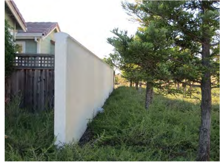
Figure E.19: Soundwall alignment, no deformation [NSF-GEER; GPS N38.096, W122.276; 08/24/14; 17:31]
