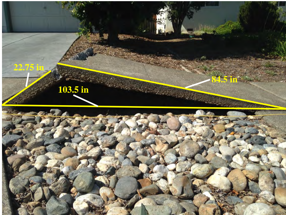
Figure 5.3: Measuring a typical buckled compression zone in sidewalk pavement [NSF-GEER; N 38.3039 W 122.3430; 8/26/2014 15:24]
