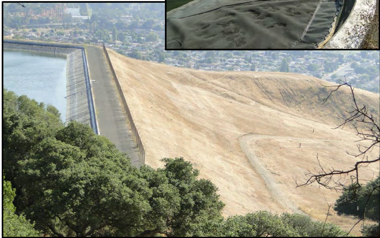
Figure F-8: Views of Summit Reservoir Dam looking southeast [NSF-GEER; Napa, CA; N38.153 W 122.225; Harder, L. F.; 08/27/14]
