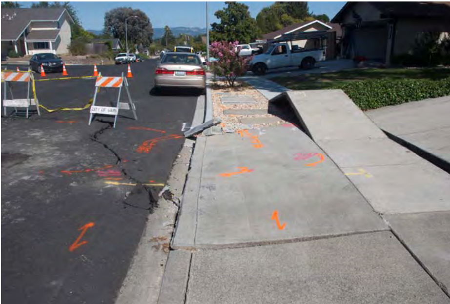
Figure 3-9. Surface rupture disrupting sidewalks and curb on Twin Oaks Drive in Napa. Right-lateral displacement was on the order of 10 – 20 cm at this location [NSF-GEER; GPS 38.3024°, -122.3438°; 08/26/2014]
