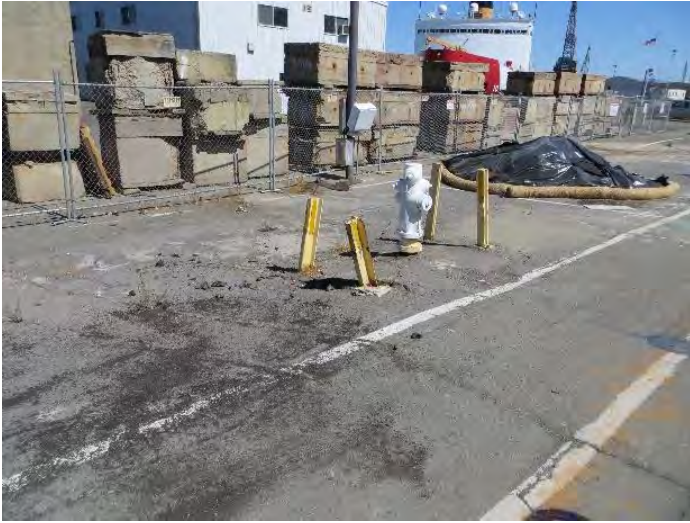
Figure E.18: Hydrant, no damage [NSF-GEER; GPS N38.097 W122.268; 08/24/14; 14:51]
