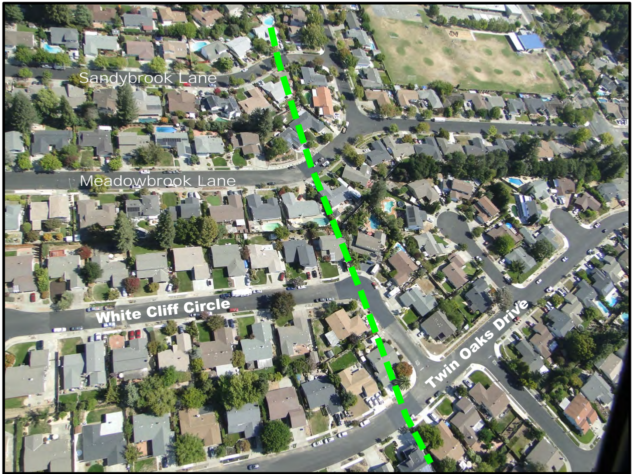
Figure 2: Alignment of surface cracking observed along Alignment A in Browns Valley following August 24, 2014 Magnitude 6 Napa Earthquake - see dark asphalt patches [NSF-GEER; Napa, CA; N 38.304 W 122.344; Harder, L. F.; 09/01/14]
