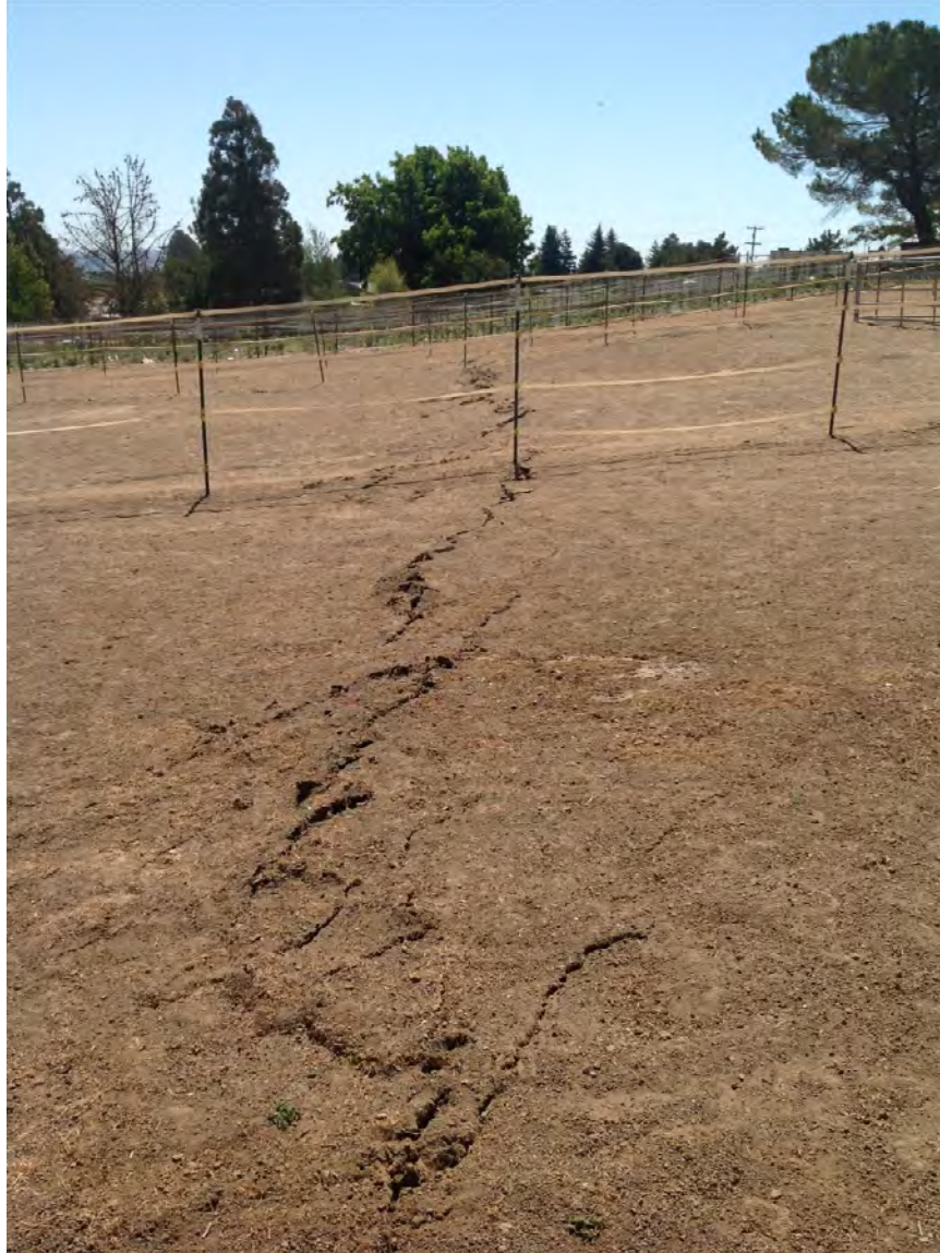
Figure 3-5. Left-stepping pattern of surface fault rupture crossing horse corral near Cuttings Wharf Road. Note variation in width of zone. Offset at this location was initial on the order of ~10 - 20 cm, although offsets later grew due to afterslip. [NSF-GEER; GPS: 38.2555°, -122.3270°; 08/24/2014]
