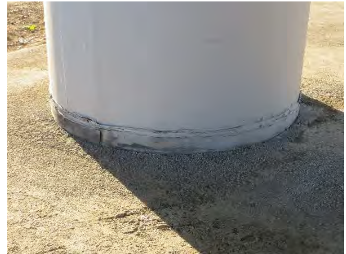
Figure E.25: Highway 37 Bridge pier, no damage [NSF-GEER; GPS N38.122 W122.276; 08/24/14; 18:24]
