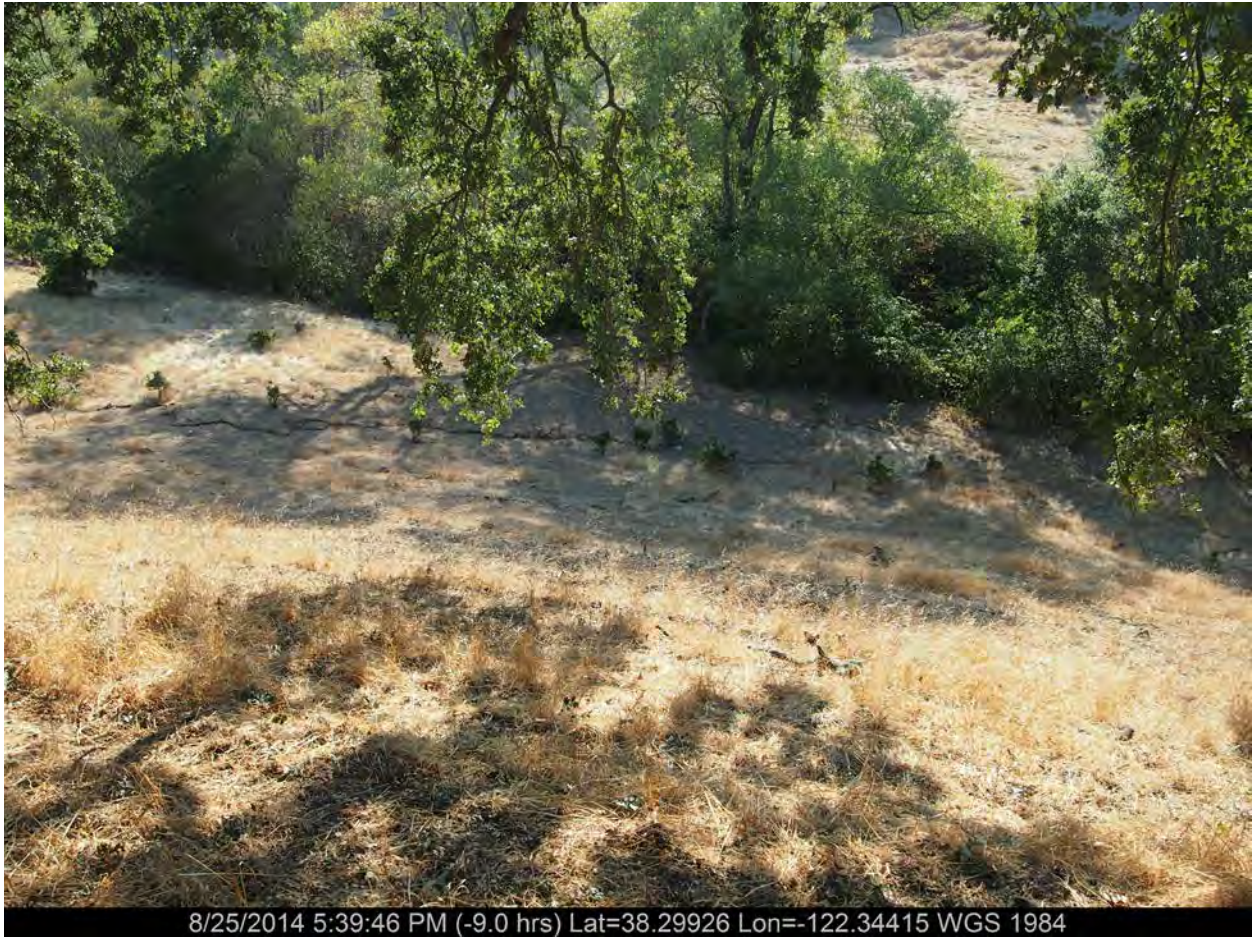
Figure 7. Photograph showing linear mole track in alluvial surface adjacent to unnamed creek. Location is along trend with deformation shown in Figures 5 and 6. Feature estimated at appx.20 m long, with apparent vertical displacement of appx.3-4 cm. [NSF-GEER; N38.2992, W122.3441; 08/25/14; 5:39 PM]
