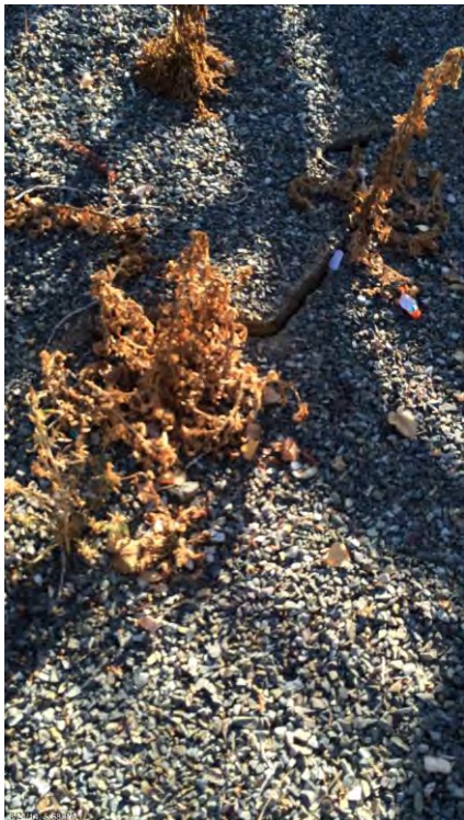
Figure E.43: Crack along sheet pile wall behind the retaining wall in the Pedestrian Bridge [NSF-GEER; N 38.3003 W -122.2881; 08/24/14 17:58]
