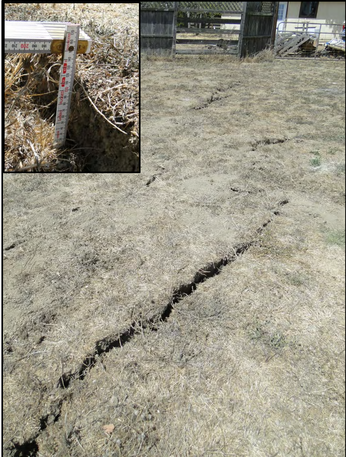
Figure 7: Photograph of ground cracking on property (Congress Valley Road, Point B4) – looking northerly from damaged Old Sonoma Road (Point 5) - vertical offset up to 12 centimeters with west side up [NSF-GEER; Napa, CA; N 38.284 W 122.325; Harder, L. F.; 08/29/14]
