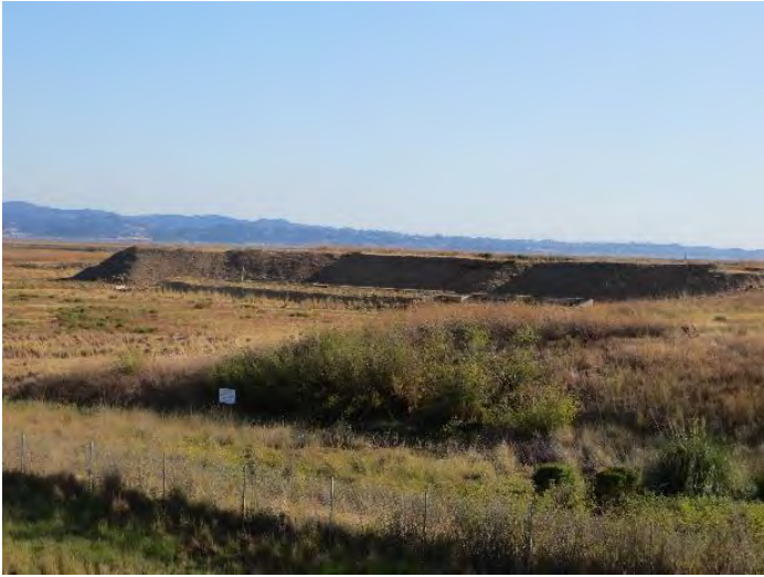
Figure E.22: Slope, no damage [NSF-GEER; GPS N38.092 W122.277; 08/24/14; 17:50]
