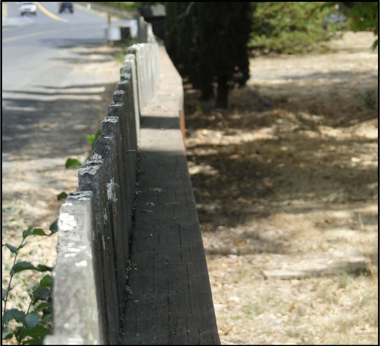
Figure 5: Photograph of wooden fence displaced by ground cracking in front of residence (Congress Valley Road, Point B4) – looking easterly – right lateral fence displacement across ground cracking is approximately 5 to 8 centimeters [NSF-GEER; Napa, CA; N 38.284 W 122.325; Harder, L. F.; 08/29/14]
