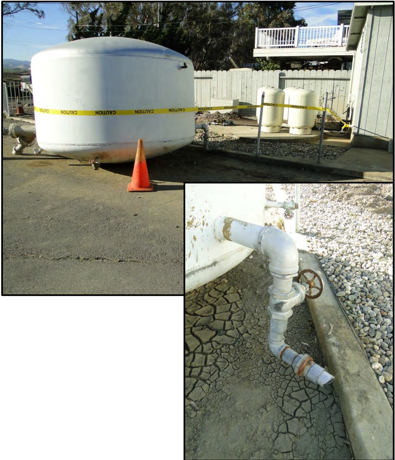
Figure F-22: Photographs of displaced water tank moved off its concrete pad and sheared pipe connection – note replacement tanks on pad in its place - on Edgerley Island south of the epicenter [NSF-GEER; Napa, CA; N38.198 W 122.316; Harder, L. F.; 09/01/14]
