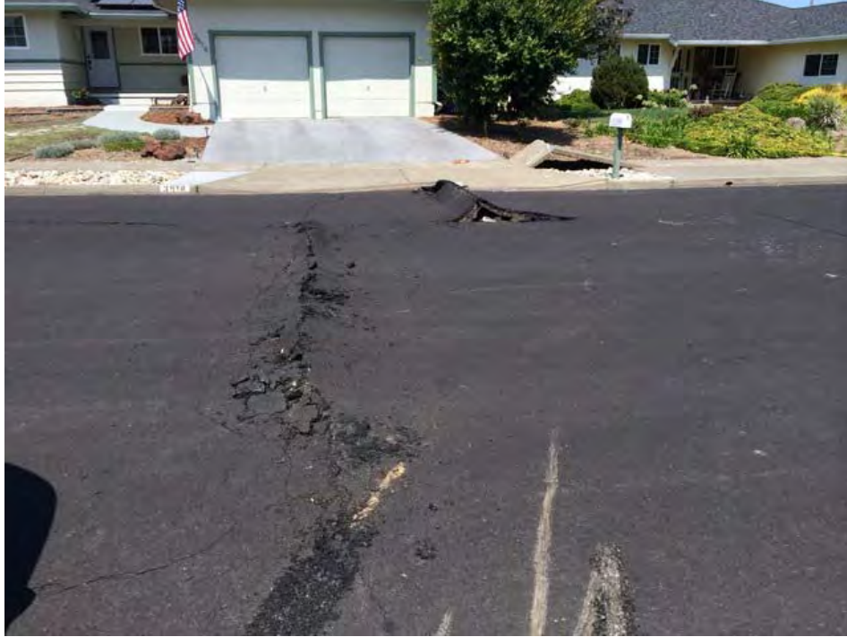
Figure C-H24-3: Asphalt rupture and front of residence (building on right) [NSF-GEER; N 38.3038 W 122.3430; 08/25/14 14:02]
