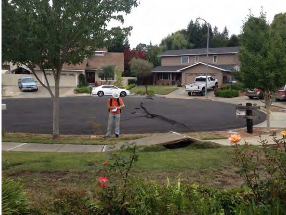
Figure C-P1-3: General view of fracturing [NSF-GEER; N 38.3018 W 122.3437; 08/25/14 10:42]
