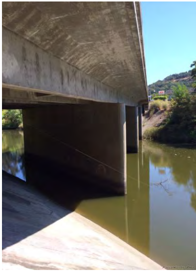
Figure E.29: Lincoln Bridge. No damage was observed. [NSF-GEER; N 38.311 W -122.278; 08/25/14 12:02]
