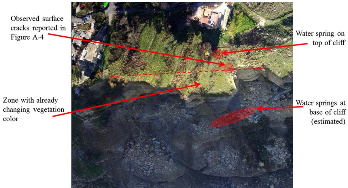
Figure 19: High risk area based on vegetation color change, observed surface cracks and location of existing joints (Picture generated form Point cloud 3D representation)
