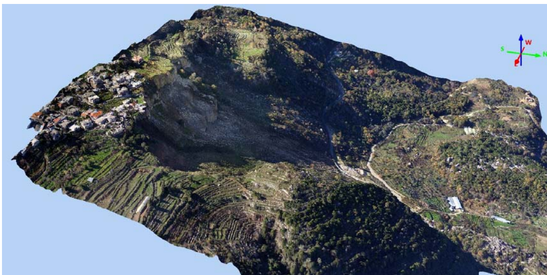
Figure 11: Point cloud 3D representation for Kfarnabrakh landslides
