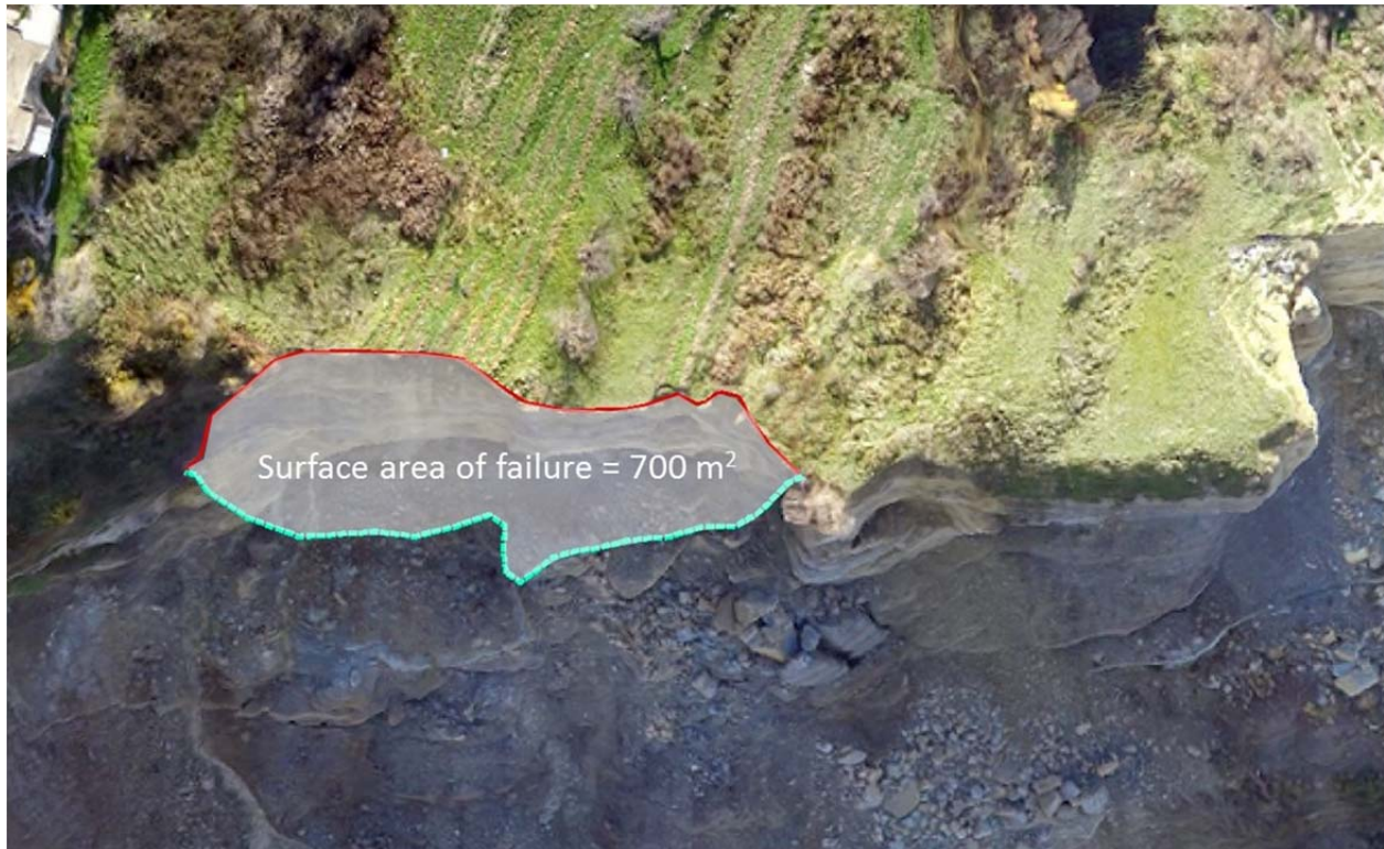
Figure 18: Cross-sectional area of 2015 failure (Picture generated form Point cloud 3D representation)
