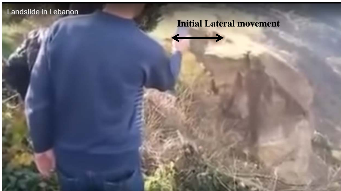
Figure 16: Snapshot from video of landslide showing a lateral displacement of the rock mass with a gap created between it and the stable ground
