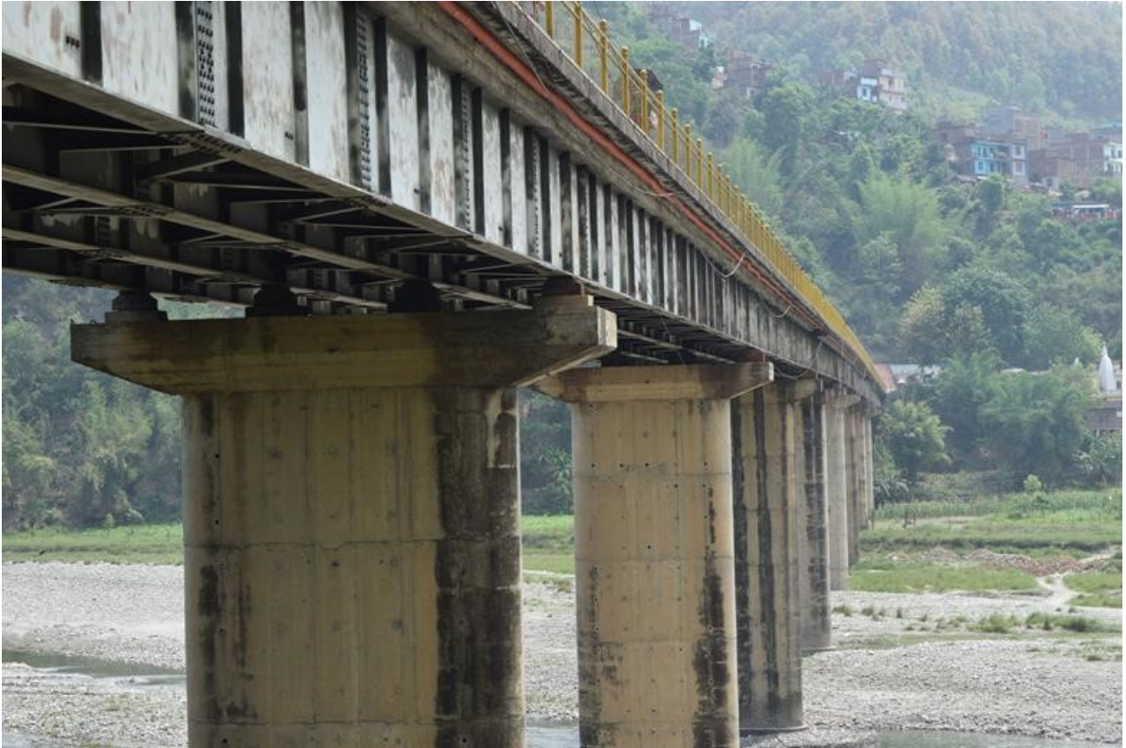
Figure 8-9 Bridge over Madi Khola along Prithvi Highway (27°40'23.1"N 85°20'30.6"E).
