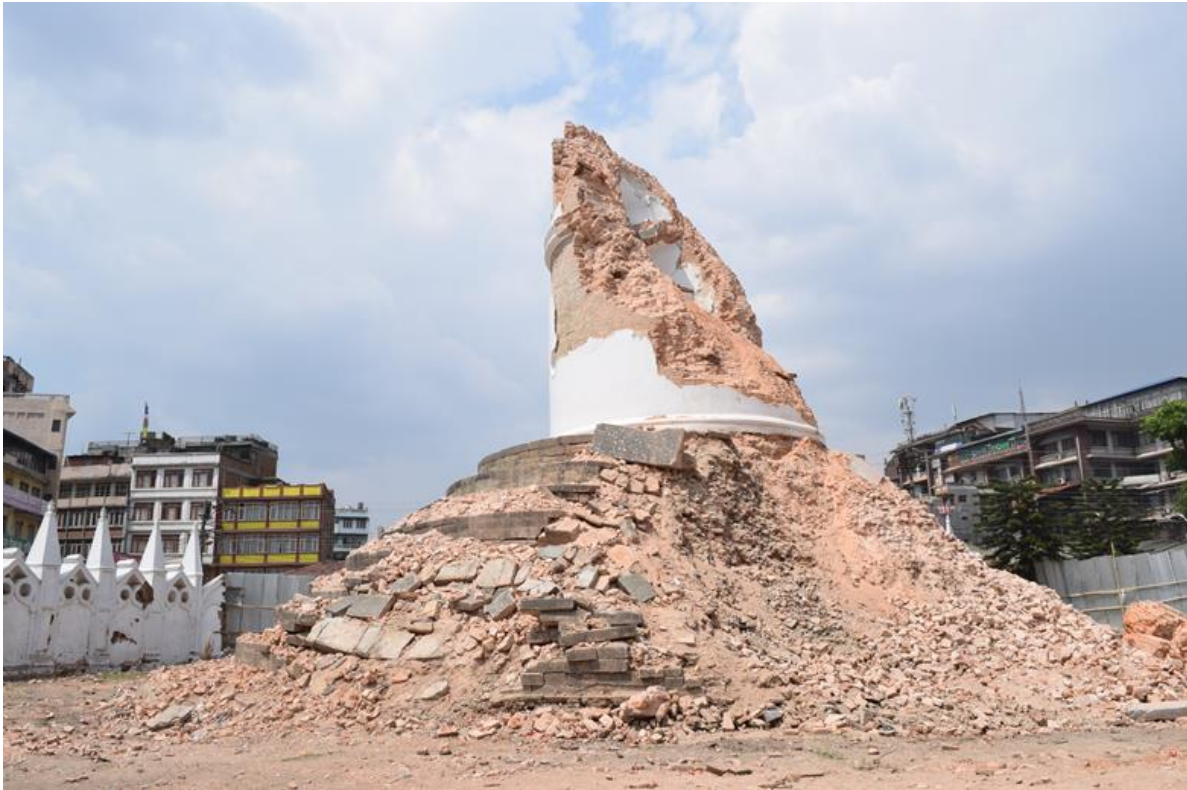
Figure 9-1 Seven story tall Bhimshen Tower collapsed due to earthquake shaking ( 27^{\circ}42' 2.23'' N, 85^{\circ}18'43.11'' E).
