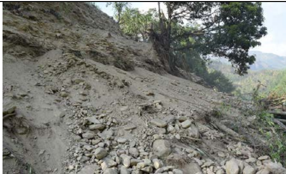
Figure 5-13 Typical rockslide mass observed along the Dolalghat-Lamo Sangu Sector of the Araniko Highway.
