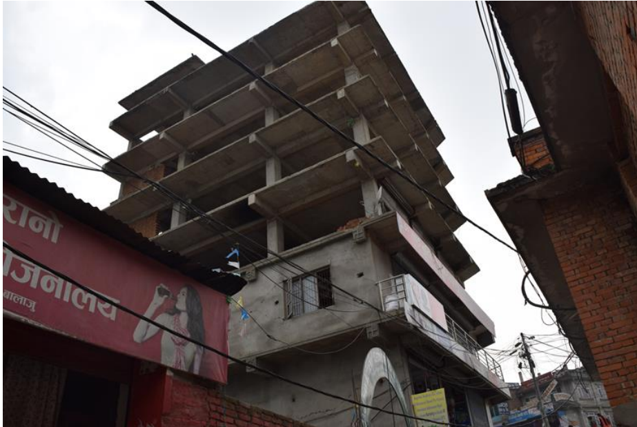
Figure 9-11 Building under construction at Balaju Baisdharma area ( 27^{\circ}44'8.28'' N, 85^{\circ}18'6.91'' E).
