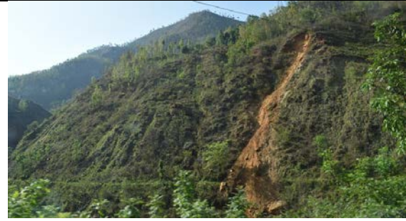
Figure 5-12 Extent of the landslides observed a few kilometers ahead of Dolalghat at Araniko Highway.
