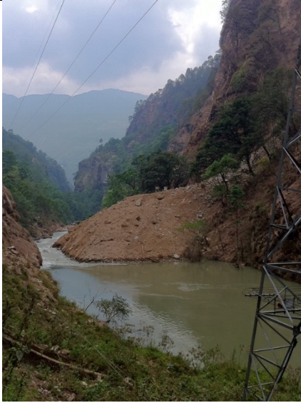
Figure 5-8 Landslide dam near the village of Listikot on the Sunkoshi River adjacent to the Araniko Highway (27° 52' 43.22" N; 85° 54' 12.17" E).
