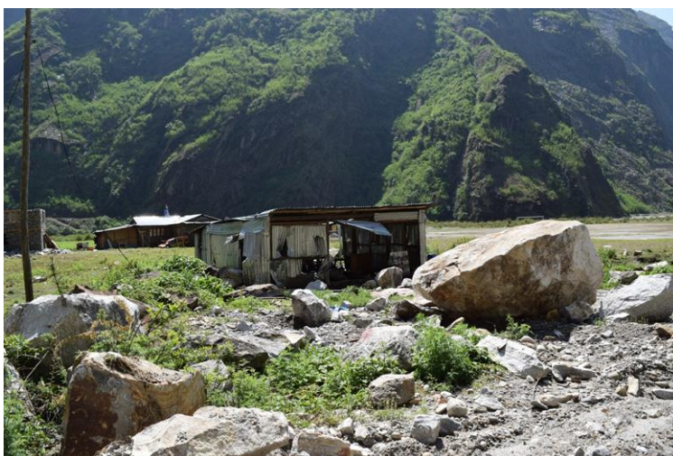
Figure 5-56 Local shop destroyed by the boulder.
