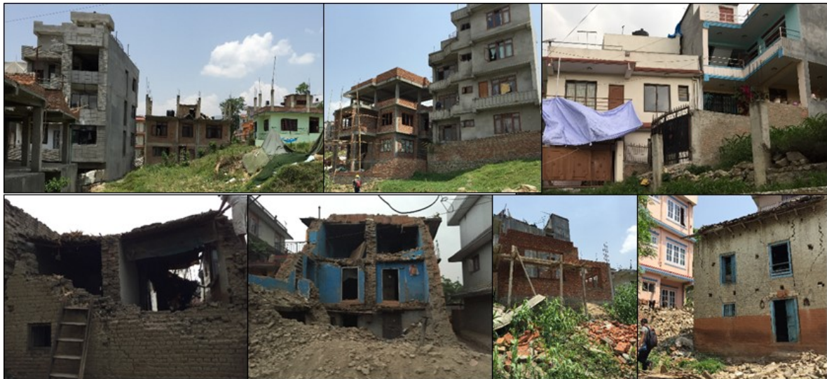
Figure 6-36 Building damage around the surface crack observed in Syuchatar.
