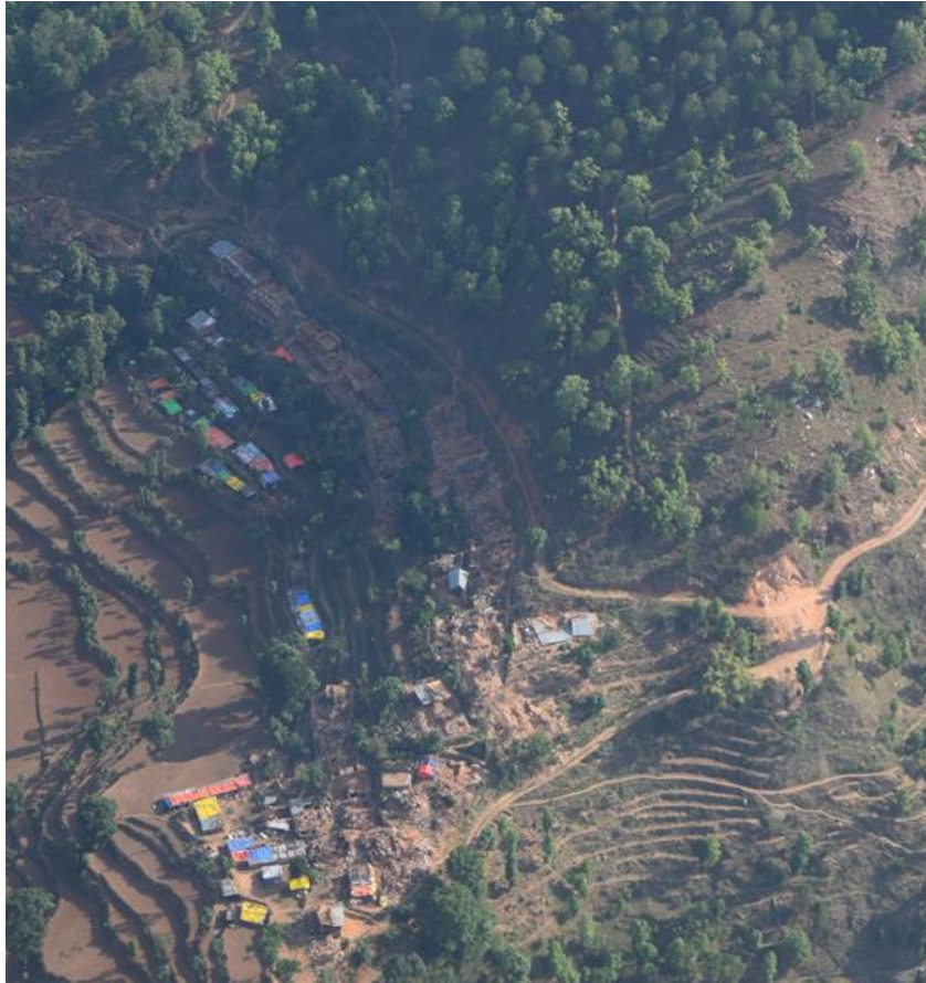
Figure 9-58 An entire village flattened in Sindhupalchowk due to strong ground shaking.
