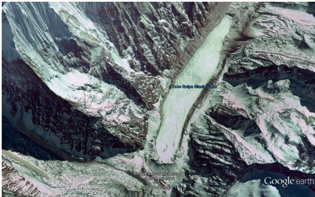
Figure 6-39 Plan view of Tsho Lorpa Glacial Lake Dam ( 27^{\circ} 52' 9.57''N , 86^{\circ} 27' 44''E ).
