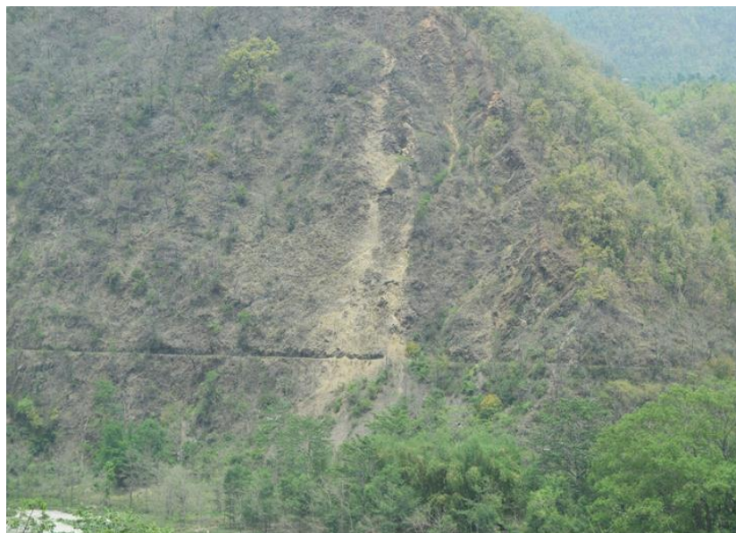
Figure 5-7 An irrigation channel alignment affected by rockslide.
