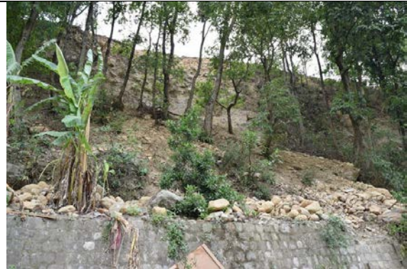
Figure 5-28 Walls performed well during ground shaking.
