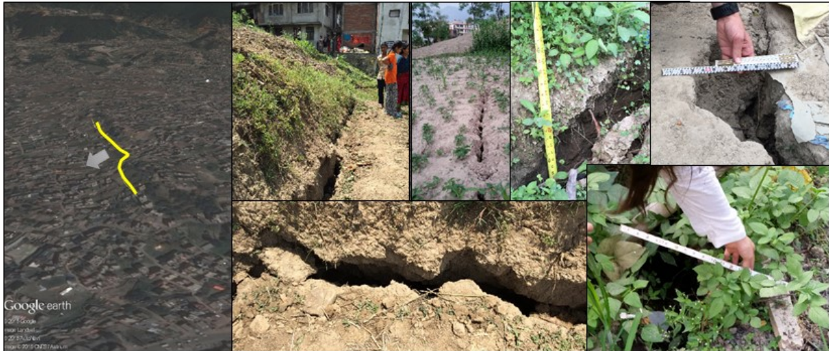
Figure 6-35 Observed surface ~1800 ft. long, ~1 ft. wide, 14ft. deep surface crack in Syuchatar.
