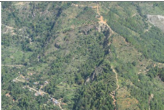
Figure 5-77 Villages below a large pre-existing landslides.
