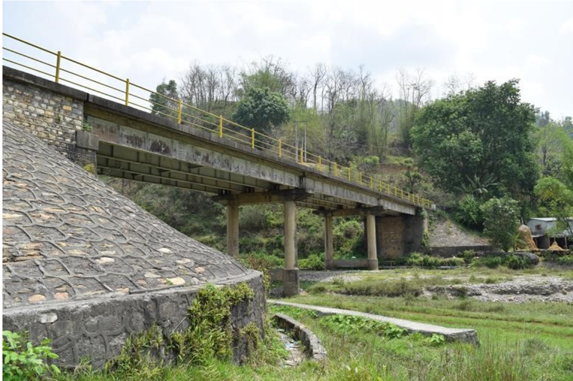
Figure 8-11 Bridge over Kumle Khola at Prithivi Highway ( 28^{\circ}1'44.022''\text{N} 84^{\circ}5'22.182''\text{E} ).
