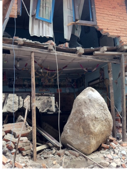
Figure 5-9 Destroyed building along Araniko Highway in Kodari (27° 58' 17.61" N; 85° 57' 43.51" E).
