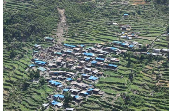
Figure 5-80 A village near Dhunche heavily damaged by the landslide debris originating from a slope above the village.
