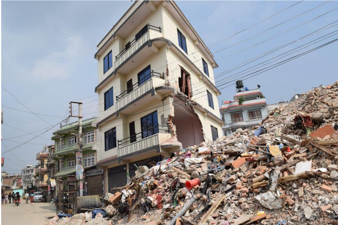
Figure 9-3 A 5.5 story building collapsed at Kapan after the ground shaking due to the M_w 7.8 Gorkha Earthquake. A total of 11 people died at this building ( 27^{\circ}43'30.0'' N, 85^{\circ}21'54.89'' E).
