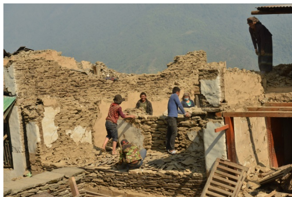
Figure 9-51 Rebuilding Barpak with stone rubble.
