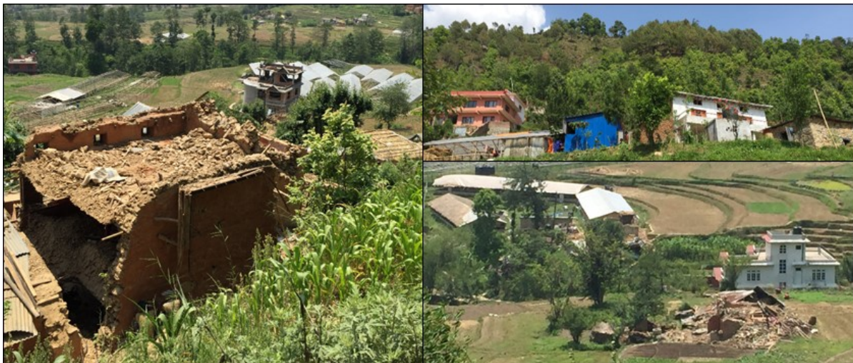
Figure 6-34 Building damage around the surface crack observed in Nagarjun
