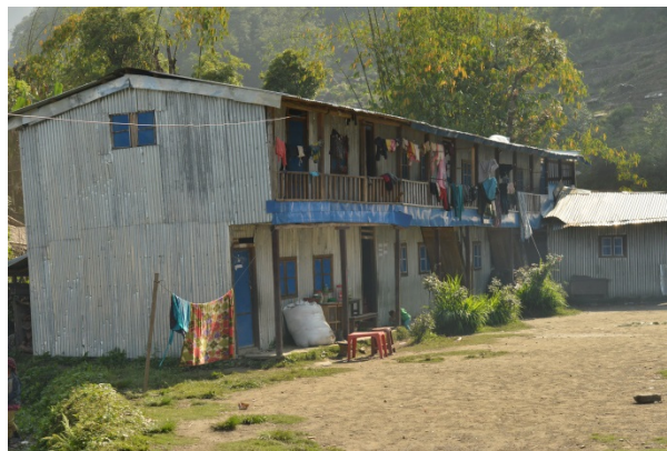
Figure 9-50 The school building of Barpak (wood framing with metal sheet siding).
