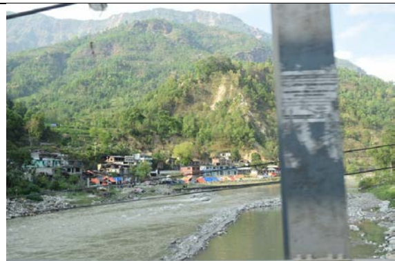
Figure 5-20 Residential area along the Araniko Highway near Lamosangu exposed to potential landslides.
