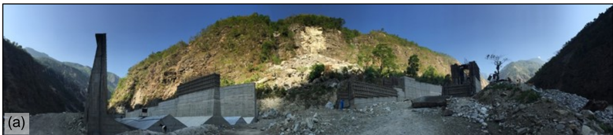
Figure 7-8 View downstream of the Upper Trishuli 3A headworks. Two of the gates are open, two closed. Due to damage to equipment and lack of vehicle access to the site, the remaining two gates cannot be opened before monsoon, which will likely lead to additional damage to the site. Flooding is also expected at the workers colony downstream (28°3'52.35" N, 85°12'20.86" E).
