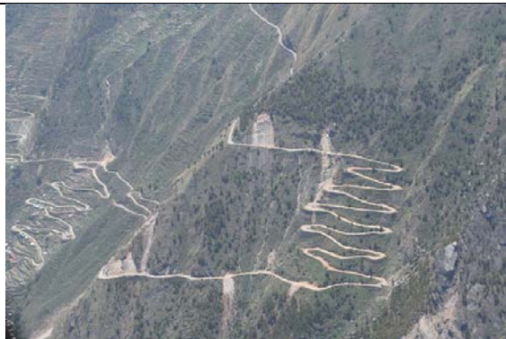
Figure 5-59 Local feeder road to the Trishuli-Rashuwagadi Road impacted by the landslide.
