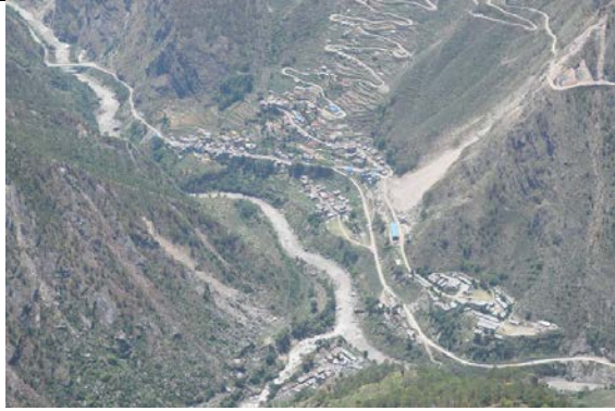
Figure 5-61 Access road to a Hydropower project being affected by the earthquake induced landslides.
