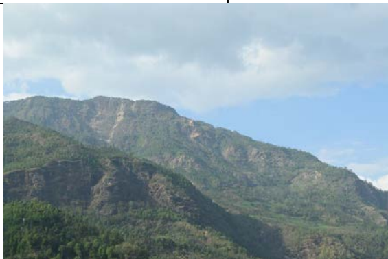
Figure 5-19 Typical cracks observed on the ridge of the mountain which has potential to trigger large scale landslides and block the Sunkoshi River.
