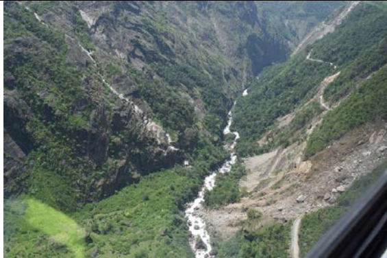
Figure 5-52 Landslide near the dam site of the hydropower project that damaged the road.
