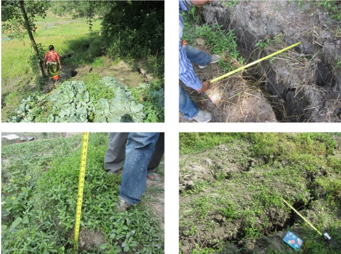
Figure 6-30 Observed surface cracks ~250m long, up to 0.8m wide, and up to 1.5m deep (Location: 27°40'42.20" N, 85°26'13.12" E)
