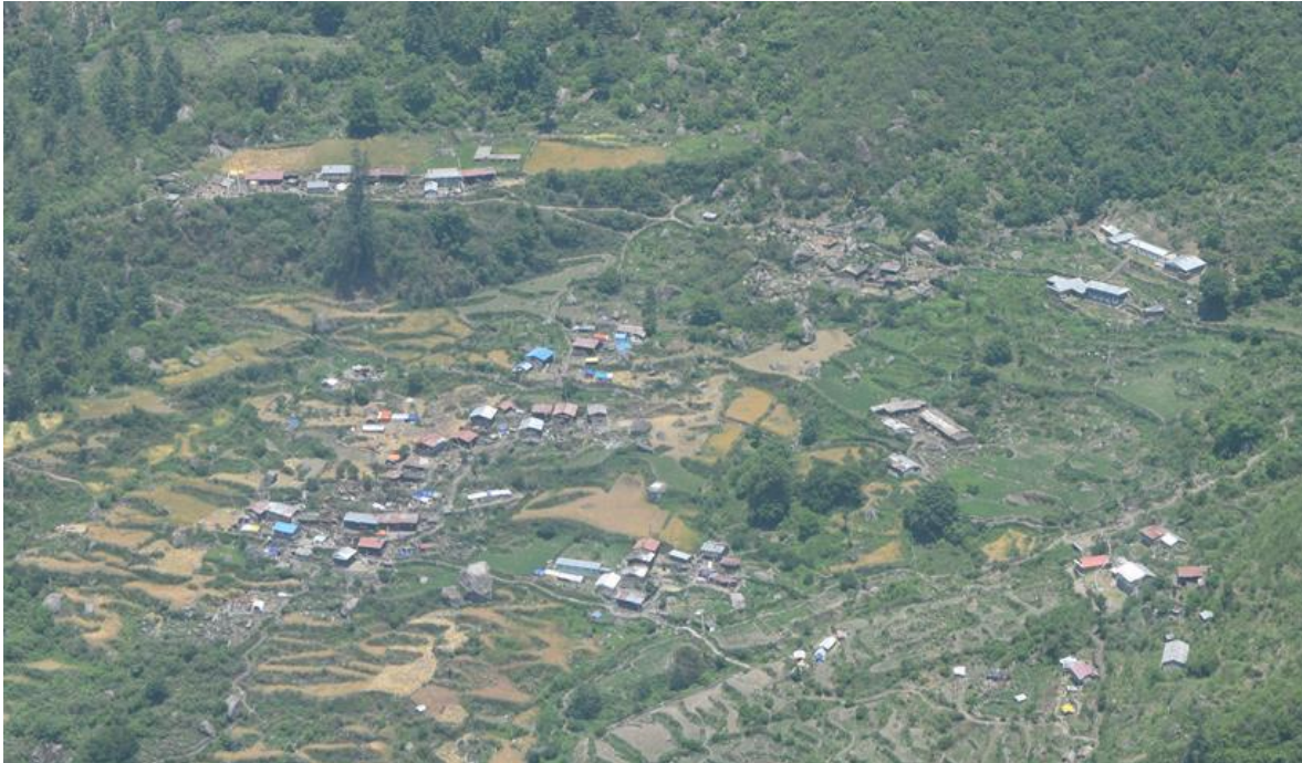
Figure 9-61 Building damage due to seismic shaking near Rasuwagadi of Rasuwa district.
