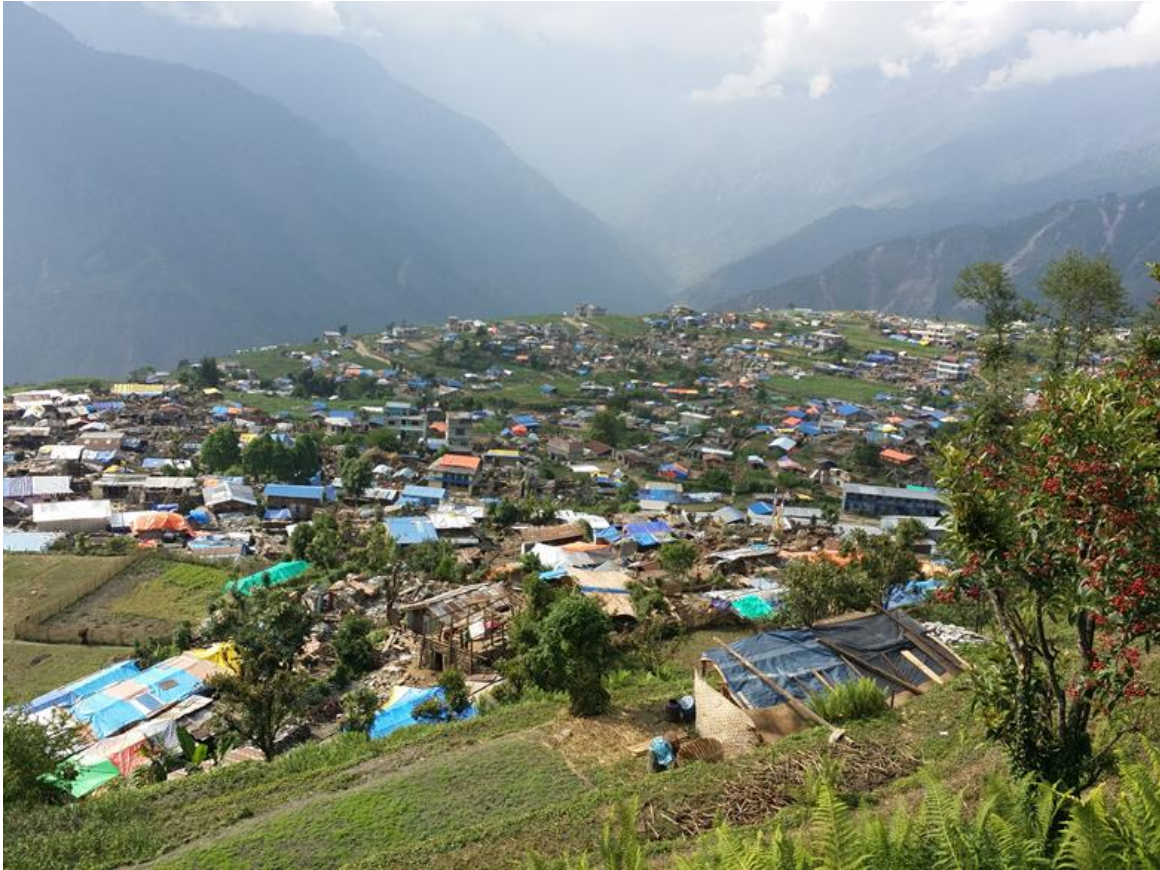
Figure 9-47 A few RCC building at Barpak Village standing well after the earthquake.
