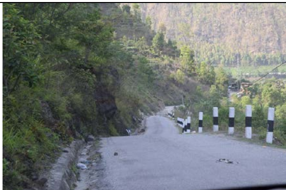
Figure 5-15 Landslide observed along the Dolalghat – Lamosangu sector of the Araniko Highway.
