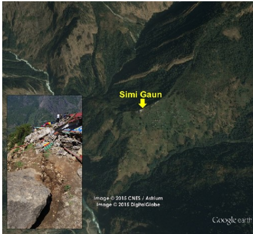
Figure 4-21 Ridge top damage and school collapse, Simi Gaun, near upper Tamakoshi Dam, (27 52' 22.5" N, 86 13' 50.6" E).
