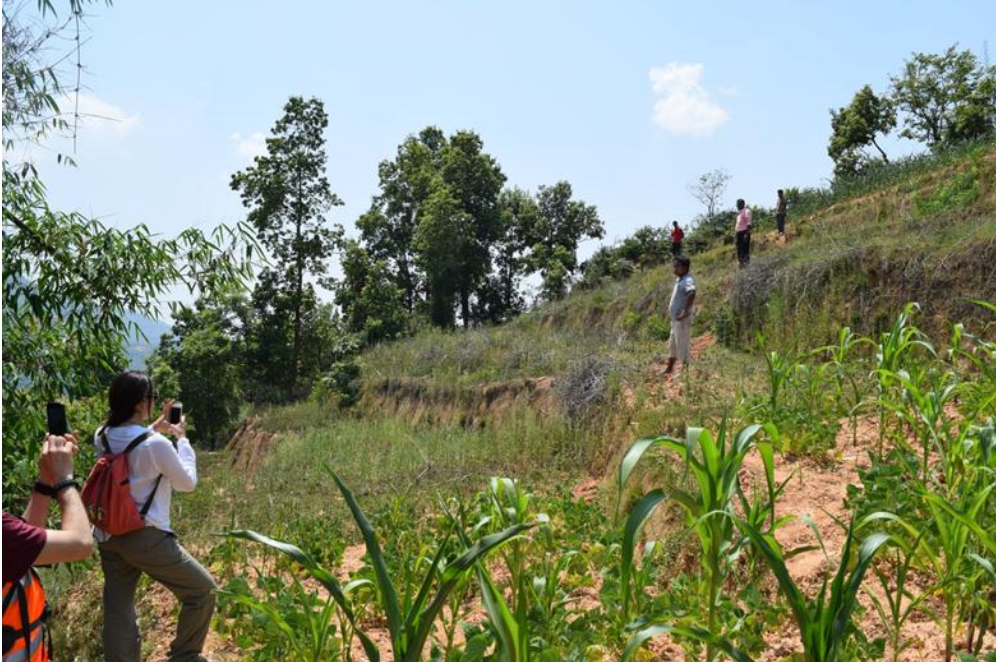
Figure 5-33 Head scarp observed on the ridge of the slope triggered by the 2015 earthquake.
