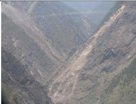
Figure 5-63 Slopes along both banks of the Trishuli River being affected by the seismically triggered landslides.
