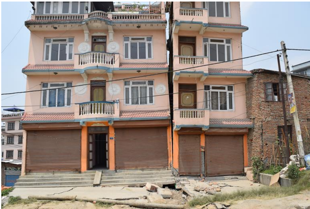
Figure 9-28 House tilted at Lokanthali area due to the lateral spread ( 27^{\circ}40'29.28''\text{N} , 85^{\circ}21'49''\text{E} ).
