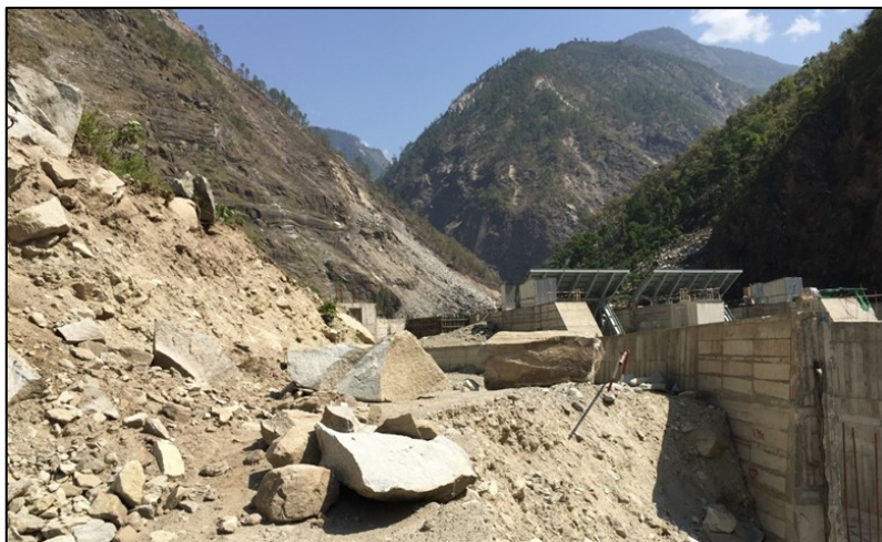
Figure 7-7 Road blocked by rockfalls through the headworks area ( 28^{\circ}3'47.21'' N, 85^{\circ}12'23.25'' E).
