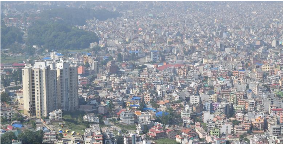
Figure 9-21 Aerial view of the apartment complex.
