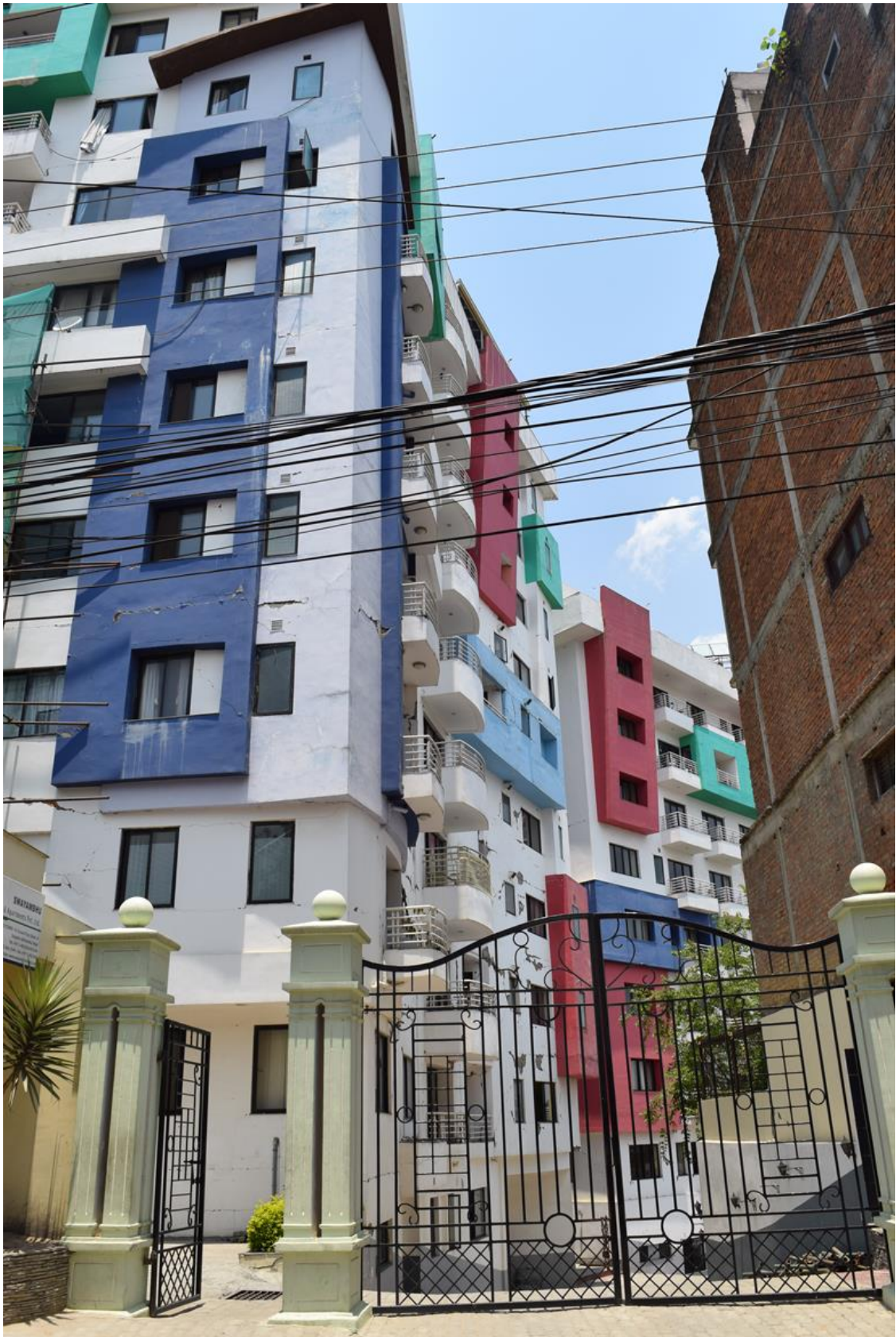
Figure 9-26 Damage observed at an apartment complex in Sitapaila
