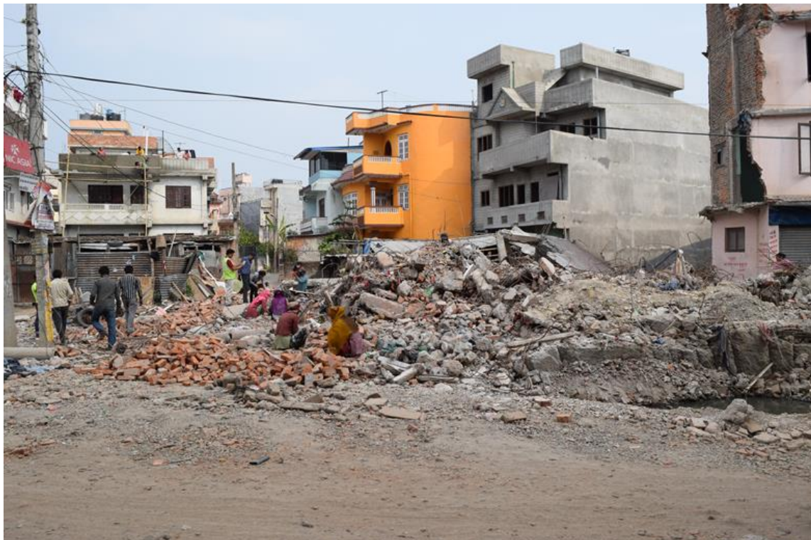
Figure 9-4 A 7 story building collapsed at Kapan after the ground shaking due to the M_w 7.8 Gorkha Earthquake. A total of 40 people died at this building ( 27^{\circ}43'26.15'' N, 85^{\circ}21'30.75'' E).
