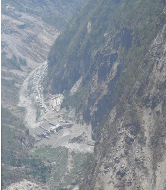
Figure 5-73 Upstream side of a hydropower project affected by large scale landslides.
