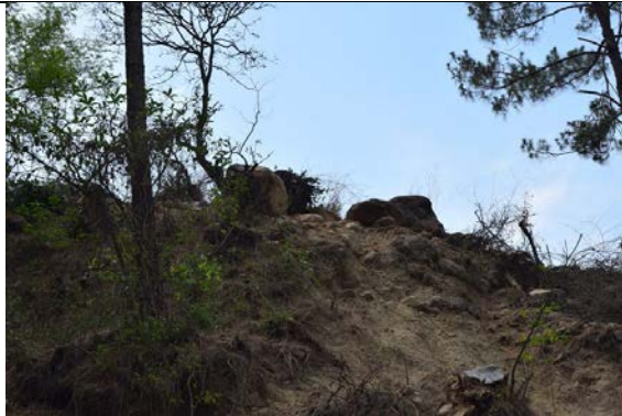
Figure 5-27 Loose boulders on top of a slope.
