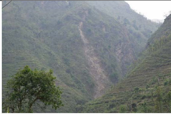
Figure 5-3 Typical landslides observed along Prithivi Highway alignment.
