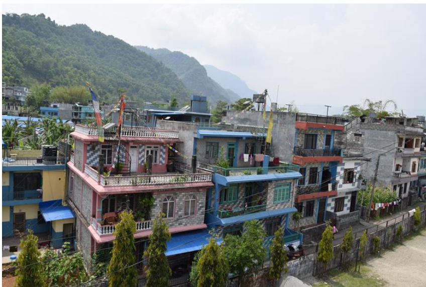
Figure 9-38 Typical building pattern in Pokhara. Majority of these buildings performed well.
