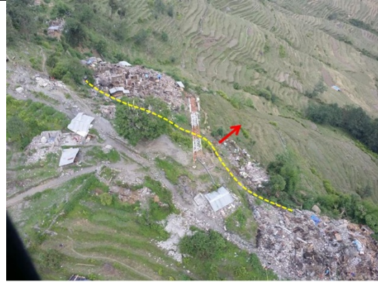
Figure 5-111 Aerial view of the landslide scarp.
