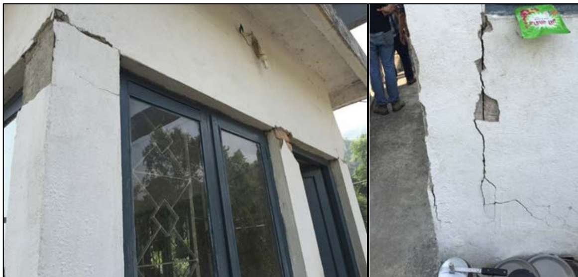
Figure 7-11 Minor damage observed from settling of fill platform adjacent to right abutment of Trishuli diversion dam. (a) foundation of the gate rack structure built on the fill pad (27°57'48.01" N, 85°10'12.52" E) and (b) Several centimeters of dilational cracking between the dam abutment, showing cracking at the edge of a retaining wall at the edge of the fill pad and the gate rack in the background (27°57'47.96" N, 85°10'13.34" E)
