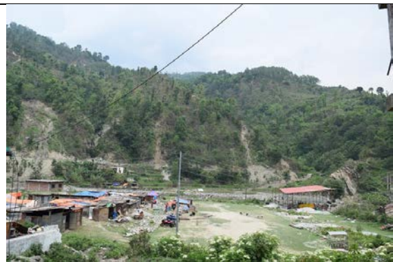
Figure 5-24 Dense landslides along the alignment of Melamchi Water Supply Project Access Road (27°49.8'0"N 85°34.5'0"E).
