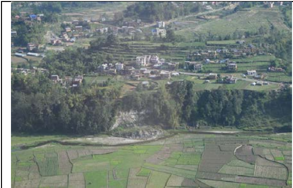
Figure 5-36 Landslide along the river bank at Indrayani, near Kathmandu Valley.
