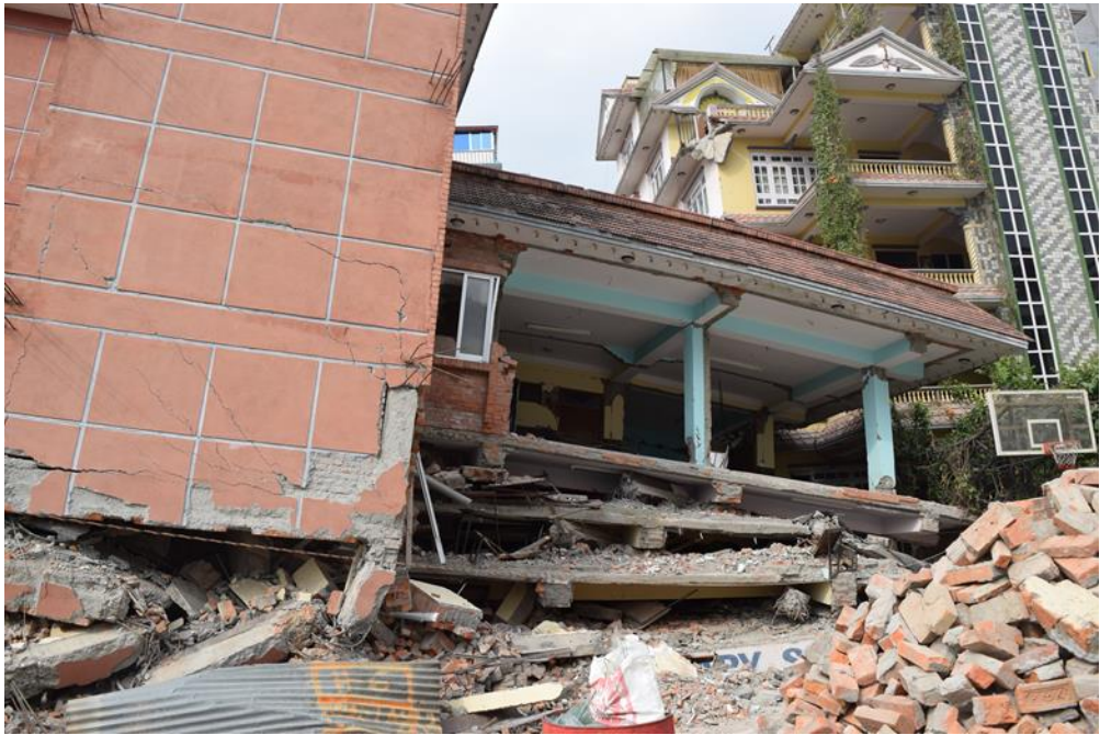
Figure 9-6 Soft story collapse of a six-story school building during the earthquake shaking (27°44'15.5" N, 85°18'33.8" E).
