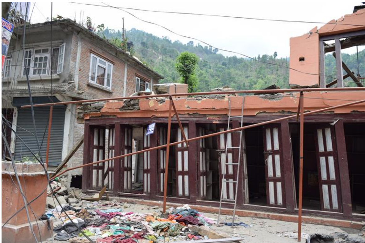
Figure 9-55 Comparison of performance of unreinforced and reinforced buildings in Melamchi, Sindhupalchowk.
