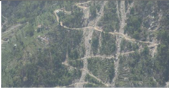
Figure 5-75 Regular road sector of the Trishuli-Rasuwagadi Road affected by landslides.
