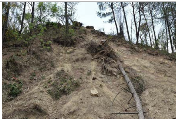
Figure 5-23 Typical rockfall source observed along the Melamchi Water Supply Project Access Road.
