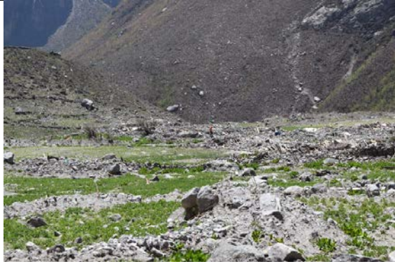
Figure 5-103 Closeup view of the debris field in the Langtang Valley. The buildings were flattened towards the direction of air blast induced by the avalanche.
