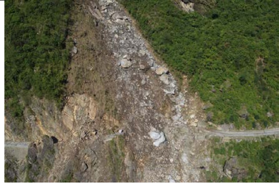
Figure 5-51. Large scale landslides that affected the Charikot-Lamabagar Road sector
