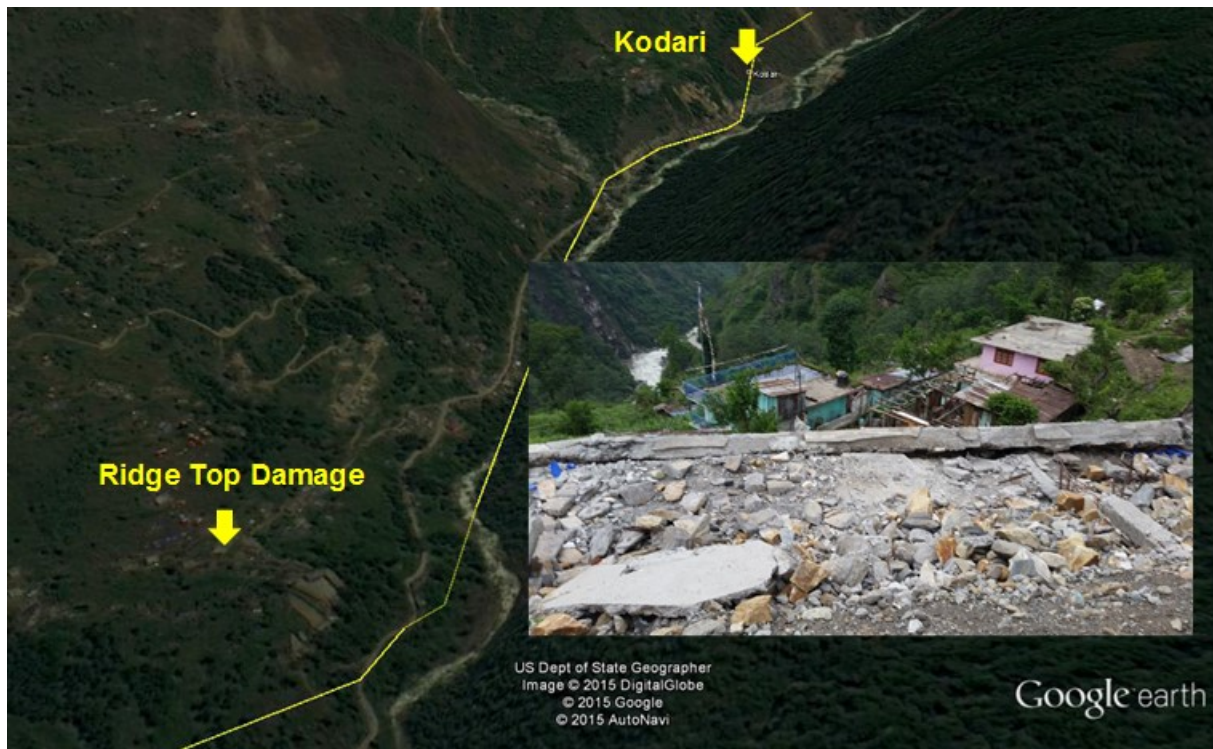
Figure 4-22 Ridge top damage and structure collapse, south of Kodari, near Chinese border (27 57' 31.9" N, 85 57' 17.7" E).
