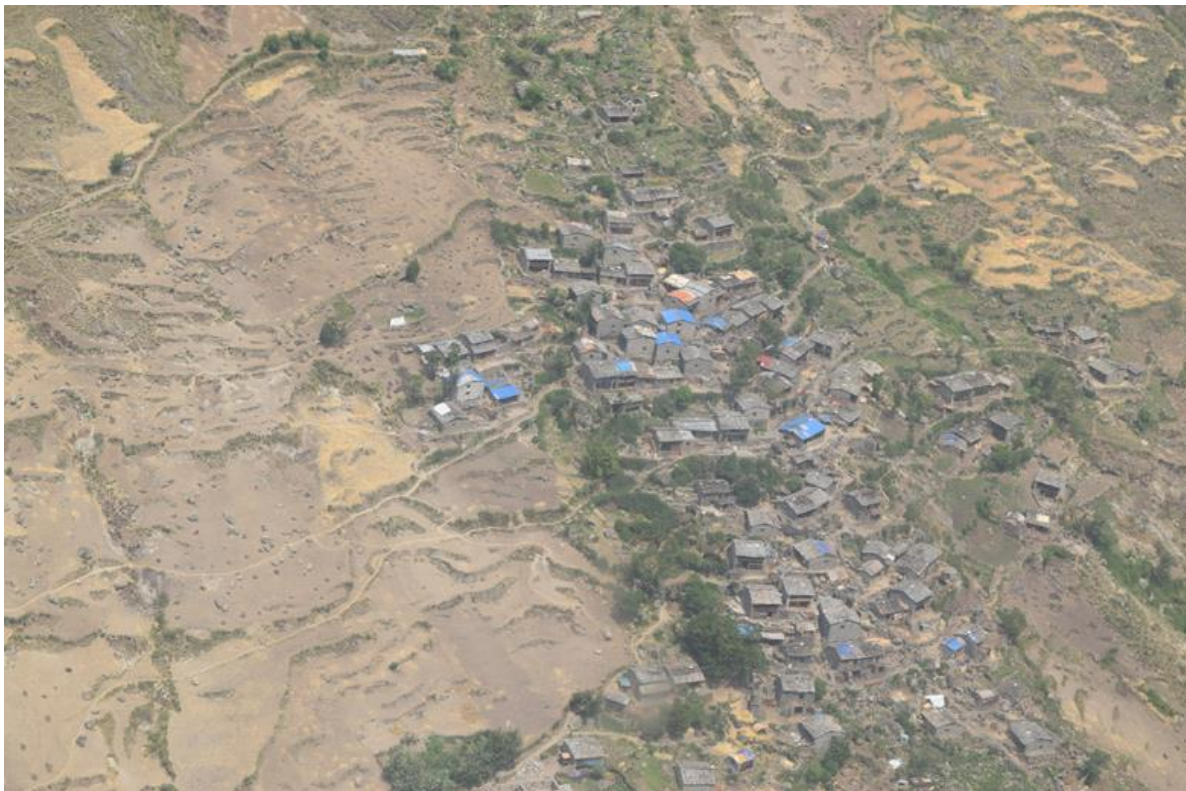
Figure 9-69 A village near Prok of Gorkha was devastated due to the seismic induced damage of unreinforced masonry structures.
