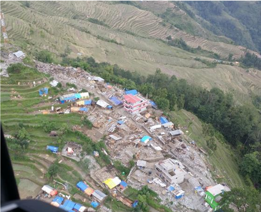
Figure 9-46 A closer look at the damage pattern in Barpak Village.
