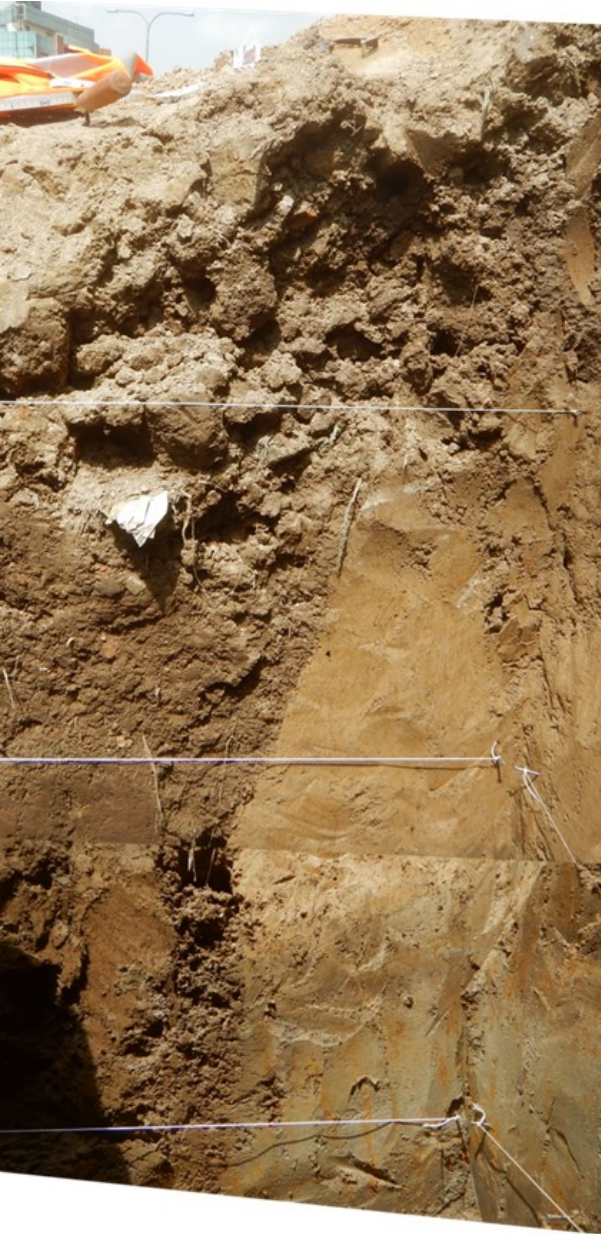
Figure 6-20. Cross section of failure plane on wall of trench at EMT04. Horizontal string is separated vertically by 0.5 m (27.67439 N, 85.36267 E).
