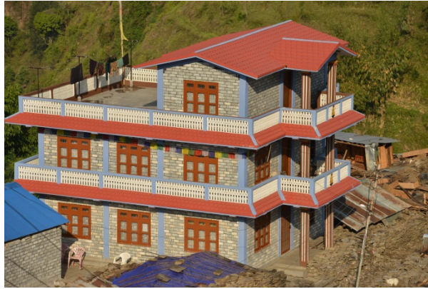
Figure 9-49 Typical condition of RCC structures in Barpak.
