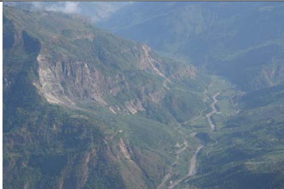
Figure 5-42 Slope vulnerable to post-earthquake rainfall induced landslides that could potentially block the natural stream.
