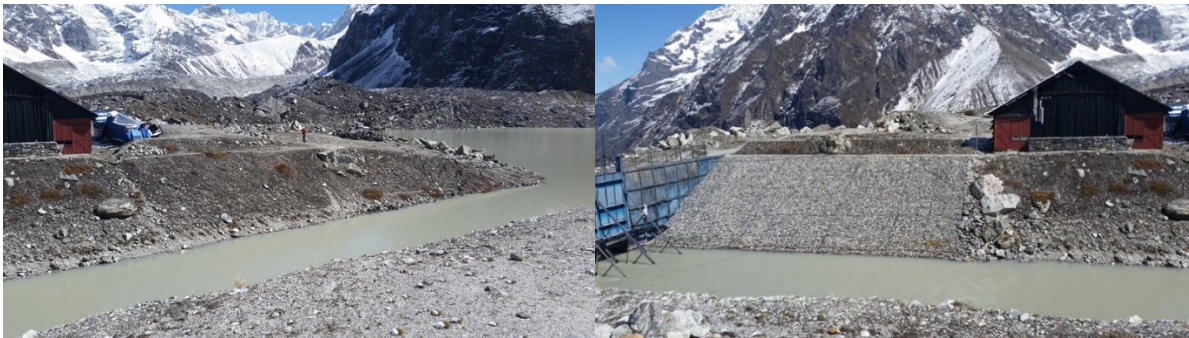
Figure 6-41 Spillway of Glacial Lake (27° 52' 9.57"N, 86° 27' 44"E).
