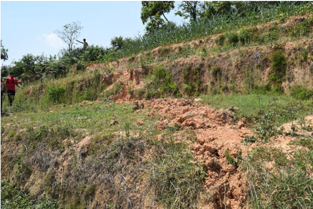
Figure 5-34 Head scarp crack was wider than 15 cm.
