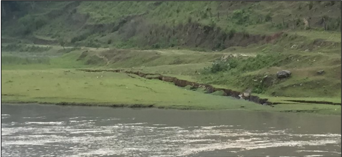
Figure 7-13 Lateral spreading around a settling pond along the canal system between the Trishuli headworks and powerhouse (27°56'15.18" N, 85°9'22.28" E).
