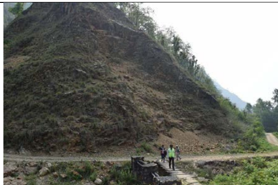
Figure 5-6 Rockslides observed at the Marshyangdi Hydropower Project dam site during the 2015 earthquake mainshock.
