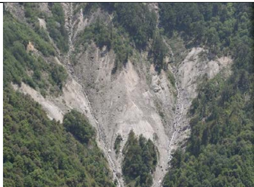
Figure 5-85 Several large scale landslides along the bank of the Langtang River.
