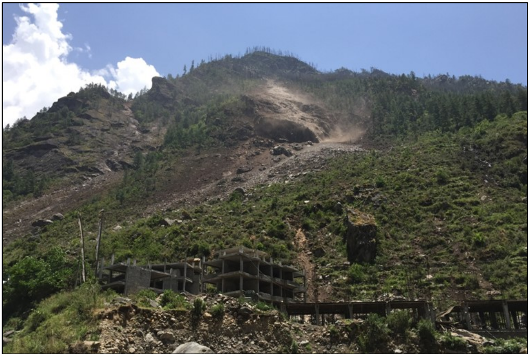
Figure 7-4 New hydro camp buildings located between the headworks and powerhouse have been impacted by some rock fall debris from above ( 28^{\circ}15'55.10'' N, 85^{\circ}22'30.11'' E).
