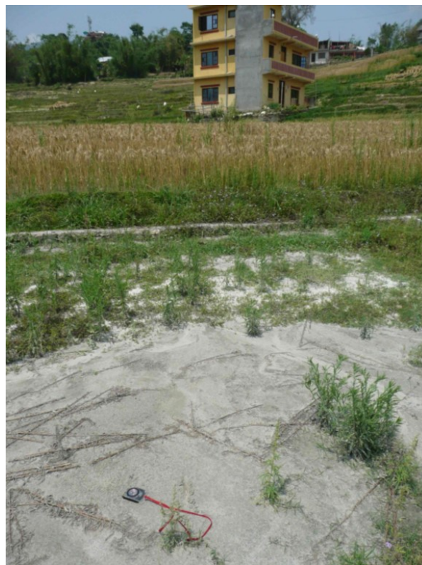
Figure 6-6. Liquefaction ejecta in agricultural field. Material was very fine, primarily silt with some sand. No damage to the building in the background (27.711025°N, 085.262290°E).
