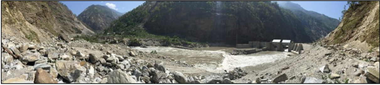
Figure 7-8 View downstream of the Upper Trishuli 3A headworks. Two of the gates are open, two closed. Due to damage to equipment and lack of vehicle access to the site, the remaining two gates cannot be opened before monsoon, which will likely lead to additional damage to the site. Flooding is also expected at the workers colony downstream (28°3'52.35" N, 85°12'20.86" E).
