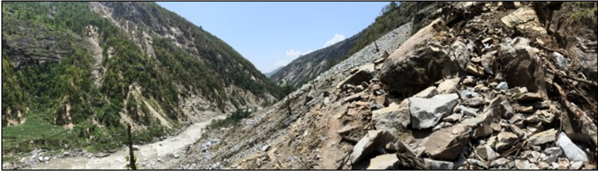
Figure 7-6 Continuous rockfalls block the main access road to the Upper Trishuli 3A headworks. The large pile of boulders on the right marks the location of the road. A walking path has been worn into the rockfall debris by villagers and dam workers. Tallus slopes in the background are all from fresh rockfalls. Vegetated debris cones on the left side provide evidence for previous rockfalls that were not reactivated during the 2015 earthquake. View is to the southwest ( 28^{\circ}2'53.76'' N, 85^{\circ}12'4.27'' E).
