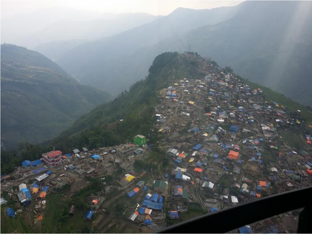
Figure 9-45 An aerial view of seismic damage at Barpak Village.
