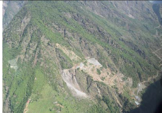
Figure 5-47 Locations with large scale landslide potential along the Charikot-Lamabagar Road.
