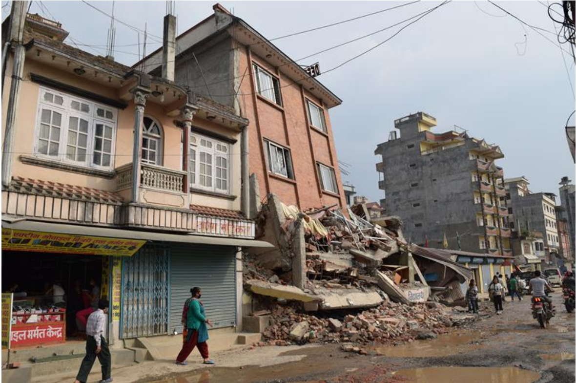
Figure 9-7 Structural damage of a RCC frame structure at Gogabu Bus Park near Balaju (27°44'7" N, 85°18'29" E).
