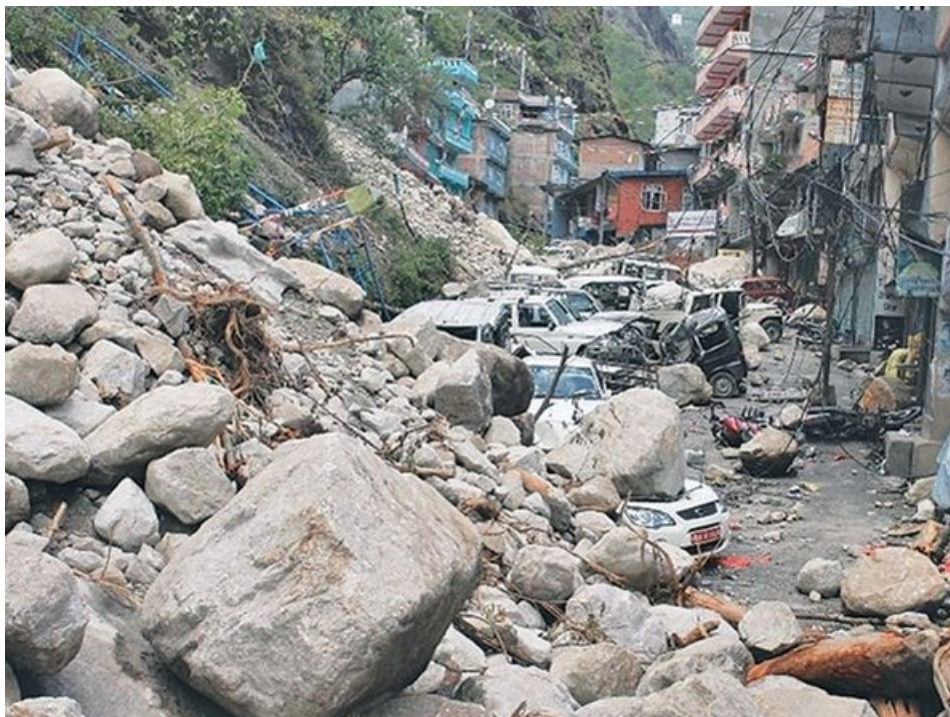
Figure 8-3 Rock falls triggered by the earthquake interrupted transportation along the Arniko Highway in Sindhupalchock. (Ref: http://www.ekantipur.com/ )
