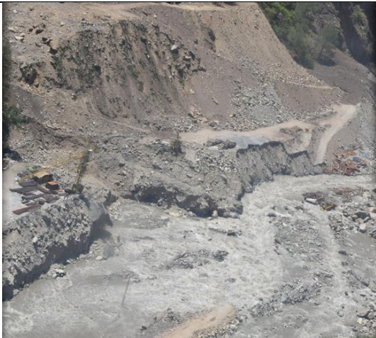
Figure 5-65 Landslide debris partially blocks the Trishuli River near a hydropower project.
