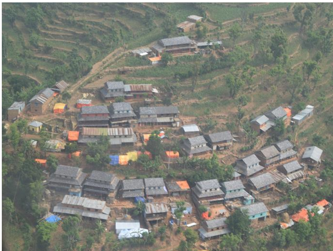
Figure 9-65 Villages near Sundarbazar did not show similar extent of damage as was observed in Rasuwa and Sindhupalchowk.
