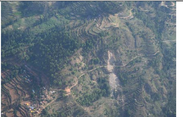
Figure 5-37 Mountain roads that have been affected by landslide triggered by the 2015 Earthquake.
