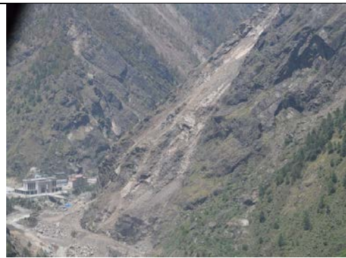
Figure 5-82 Trishuli River near the Chinese border at Rasuwagadi partially blocked by large landslides.
