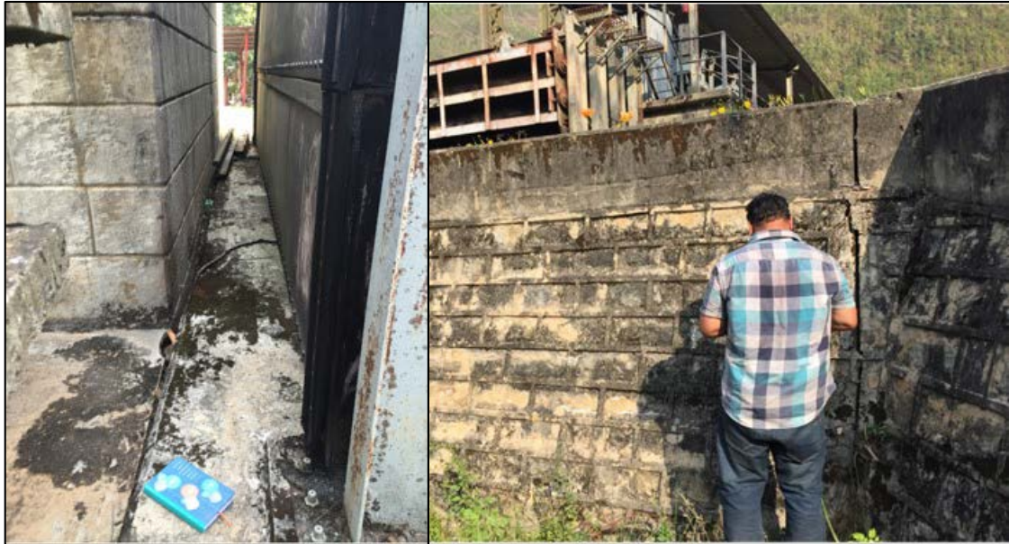
Figure 7-11 Minor damage observed from settling of fill platform adjacent to right abutment of Trishuli diversion dam. (a) foundation of the gate rack structure built on the fill pad (27°57'48.01" N, 85°10'12.52" E) and (b) Several centimeters of dilational cracking between the dam abutment, showing cracking at the edge of a retaining wall at the edge of the fill pad and the gate rack in the background (27°57'47.96" N, 85°10'13.34" E)
