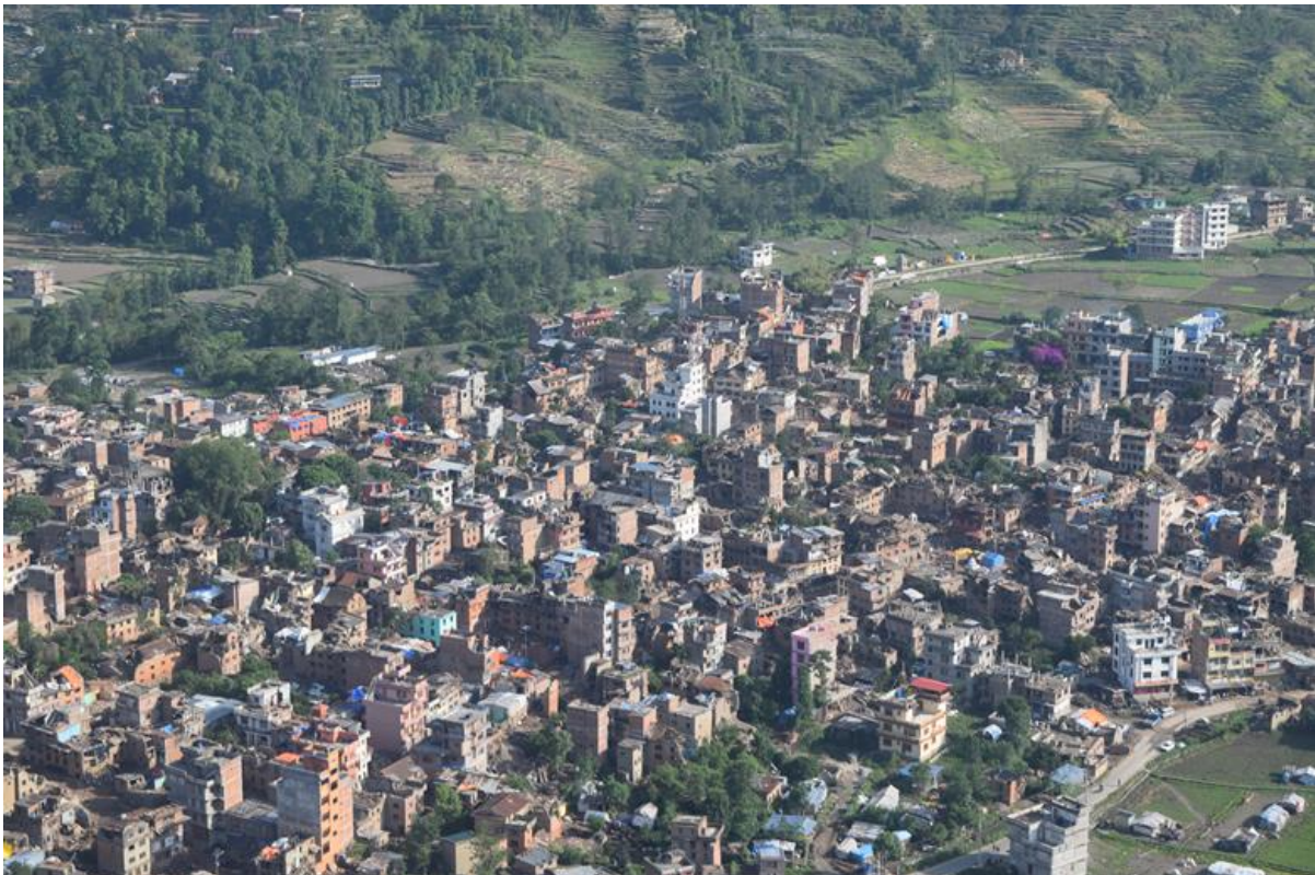
Figure 9-31 Aerial view of damage in Bhaktapur
