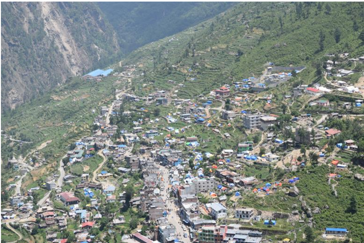
Figure 9-63 Several modern RCC structures at Dhunche of Rasuwa District performed well during the earthquake.
