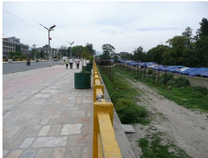
Figure 6-7. Singa Durbar Bridge (27.698793°N, 85.320060° E). To the right of the bridge can be seen the deep foundation that is currently being installed for a building.
