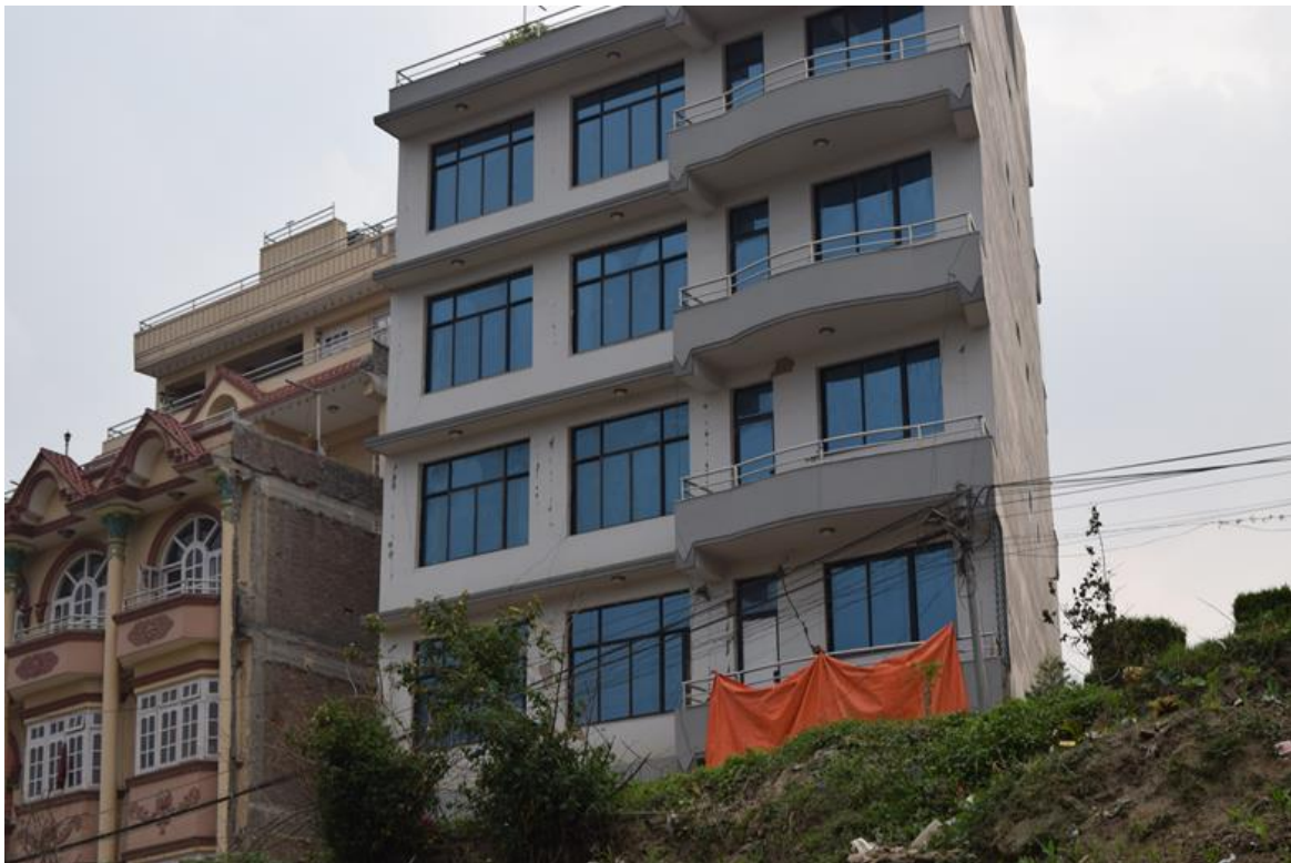
Figure 9-14 Recently constructed buildings at Sitapaila height also sustained significant damage although did not collapse ( 27^{\circ}42'51'' N, 85^{\circ}16'58'' E).
