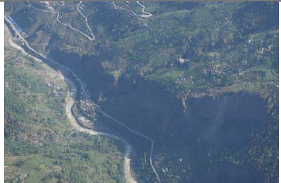
Figure 5-43 Settlement at along a bank near a potential landslide.
