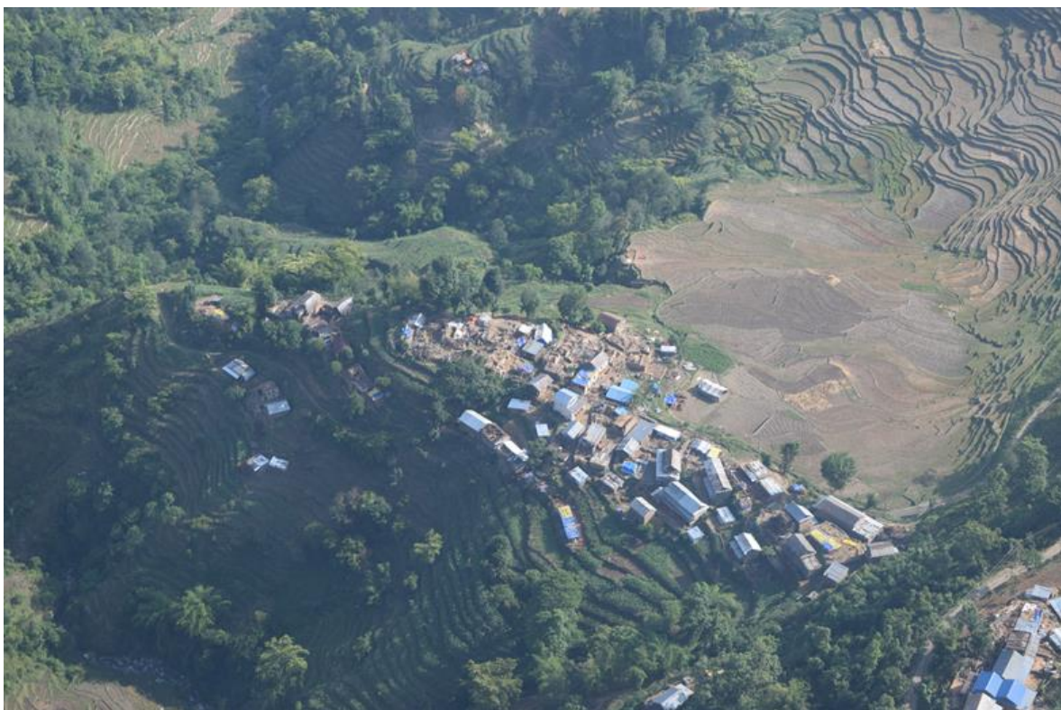
Figure 9-57 Aerial view of building damage at a ridge in Sindhupalchowk – aerial way to Lamabagar.
