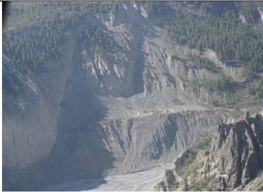
Figure 5-115 Loose sediment mass along the trekking route from Manang to Lake Tilicho ( 28^{\circ}4.97'0''N 85^{\circ}13.8'0''E ).
