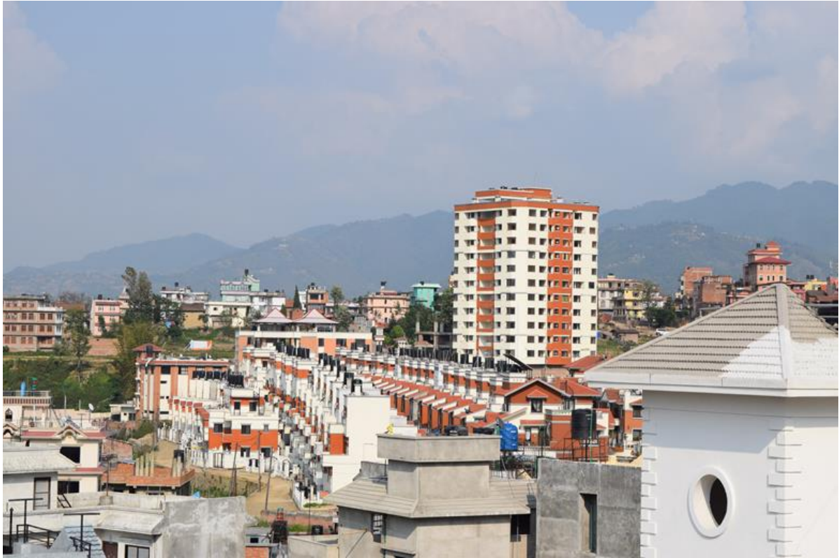
Figure 9-23 High rise apartment complex at Hattiban that sustained some damage due to earthquake shaking ( 27^{\circ}38'59'' N, 85^{\circ}19'46'' E).
