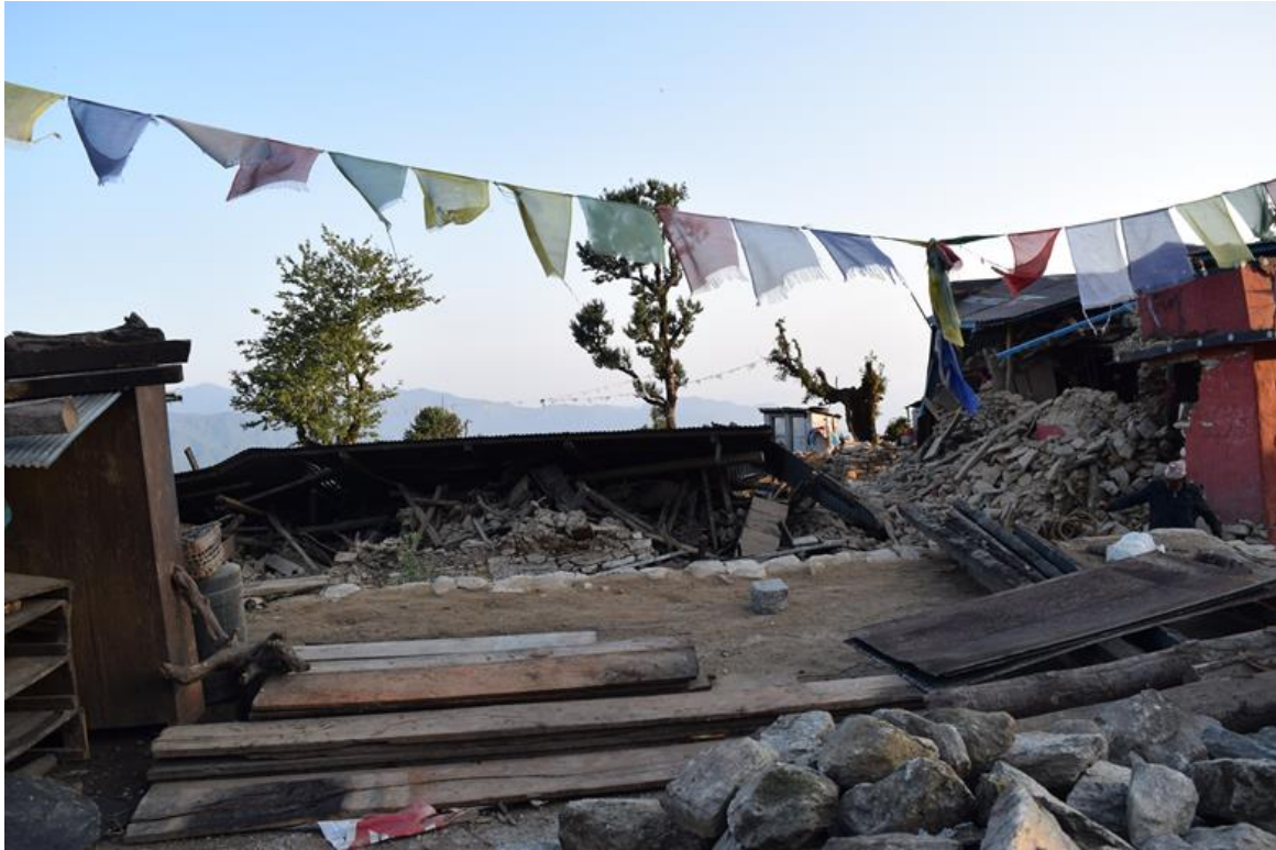
Figure 9-54 Several old unreinforced masonry buildings collapsed in Mude, Dolakha.
