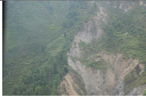
Figure 5-116 Landslides that damaged the road along Arughat-Arukhet road sector.
