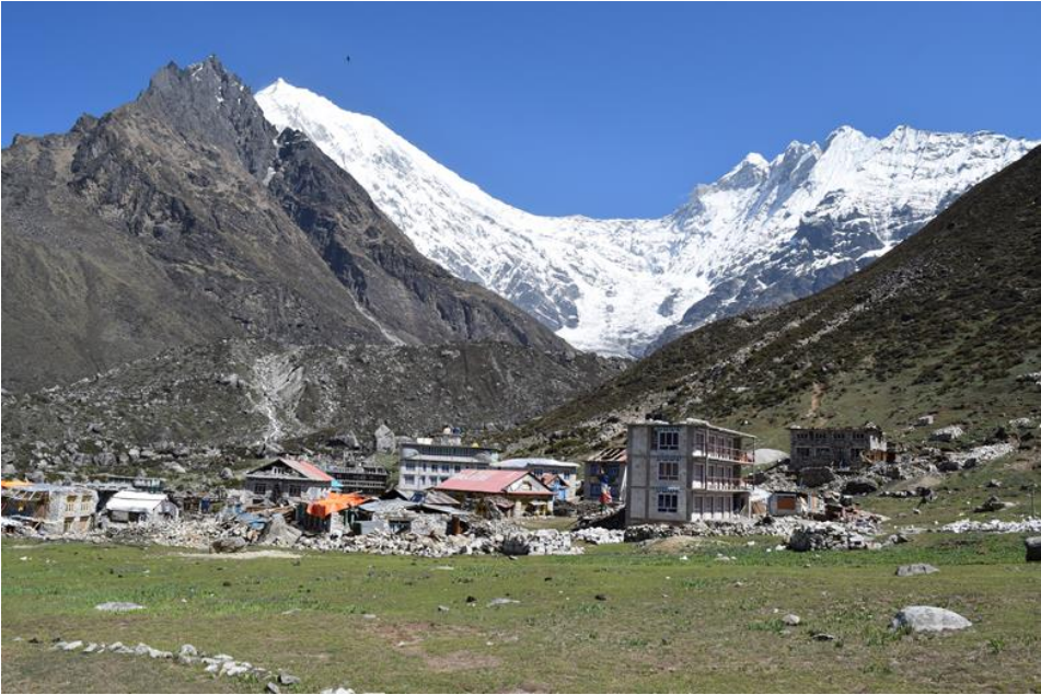
Figure 9-60 RCC structures at Kangjun Gumba, Langtang Trekking Route performed well whereas the unreinforced stone masonry walls flattened due to seismic shaking (28°12.7'0" N, 85°34.1'0" E).
