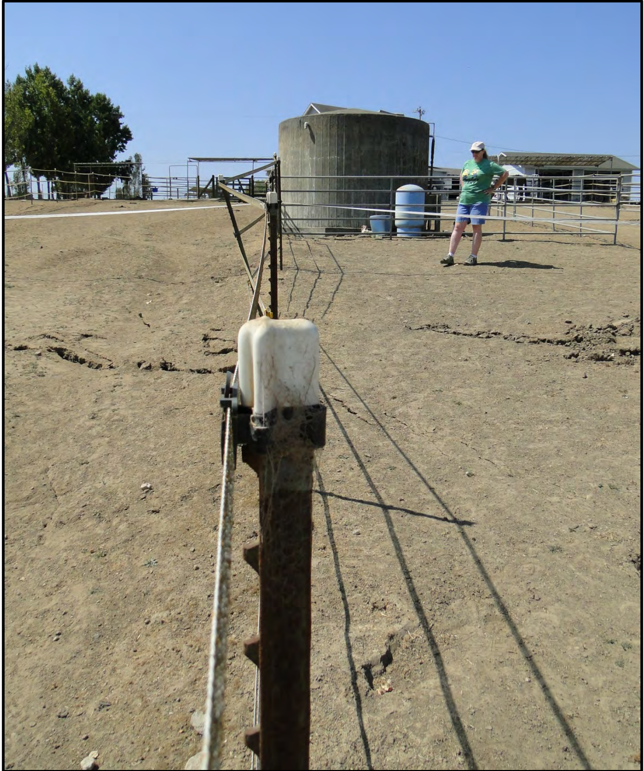
Figure 10: Photograph of electrical fence in horse pasture along Cuttings Wharf Road south of Highway 12/121 (Point A10) with approximately 4 centimeters of right lateral offset induced by ground cracking – view towards the west [NSF-GEER; Napa, CA; N 38.253 W 122.326; Harder, L. F.; 09/01/14]
