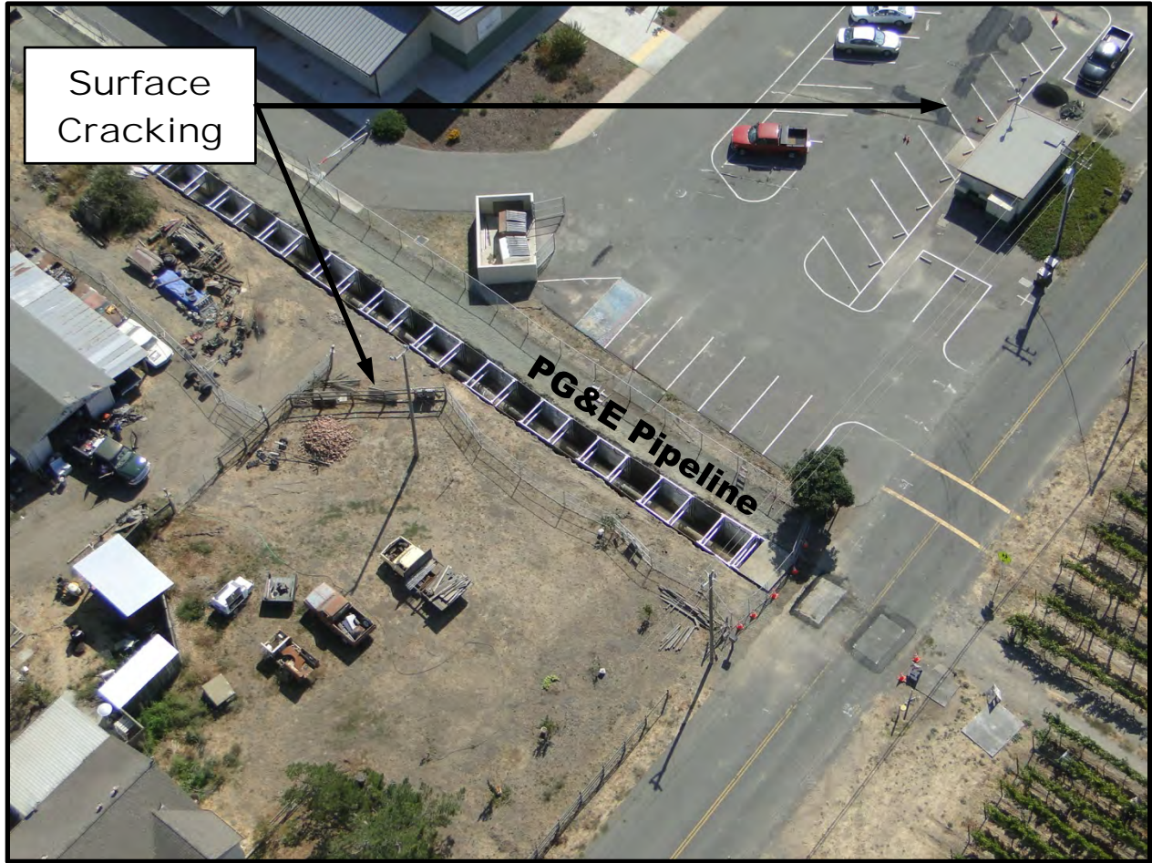
Figure 12: Aerial photograph of ground cracking crossing PG&E natural gas pipeline on Los Carneros Road near Stone Bridge School (Point A12) – view looking towards the southeast [NSF-GEER; Napa, CA; N 38.243 W 122.321; Harder, L. F.; 09/01/14]
