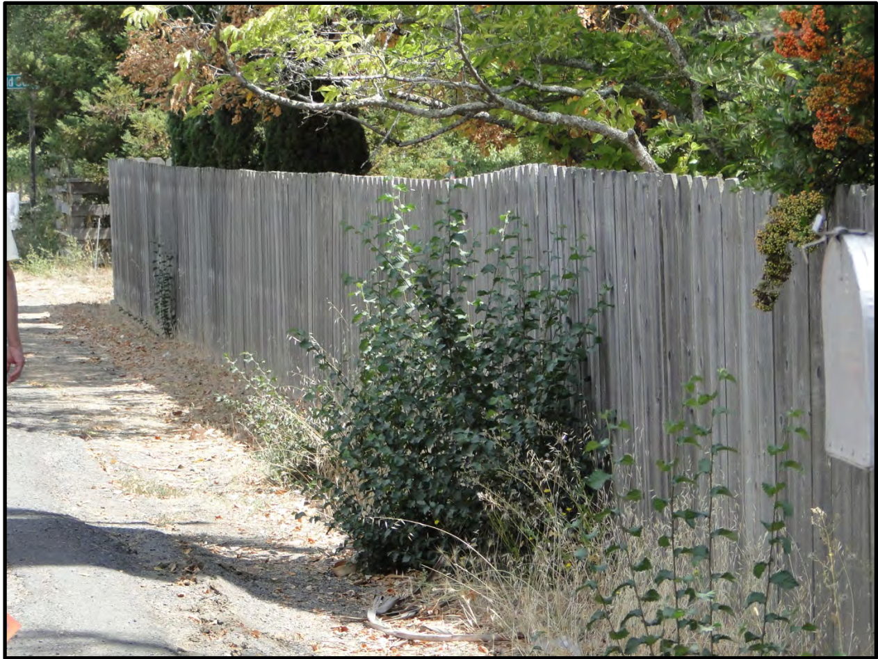
Figure 4: Photograph of wooden fence displaced by ground cracking in front of residence (Congress Valley Road, Point B4) – looking easterly – vertical fence displacements across ground cracking are approximately 8 to 12 centimeters with west side up [NSF-GEER; Napa, CA; N 38.284 W 122.325; Harder, L. F.; 08/29/14]
