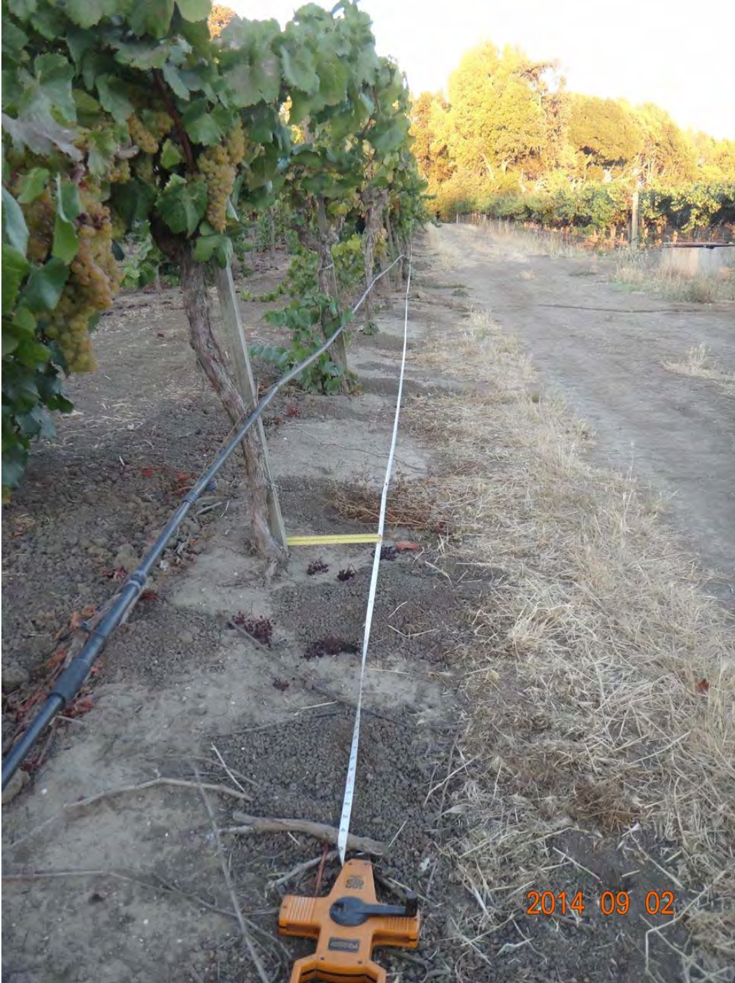
Figure 18. Surface fault rupture at Poseidon Vineyard south of Las Amigas Road (1.2 km NW of epicenter), showing measurement alignment along azimuth 090. Yellow engineer's scale is located west of fault zone, showing 20 to 25 cm of apparent offset. [NSF-GEER; GPS N38.2314 W122.3153; 09/02/14: 7:17 pm]
