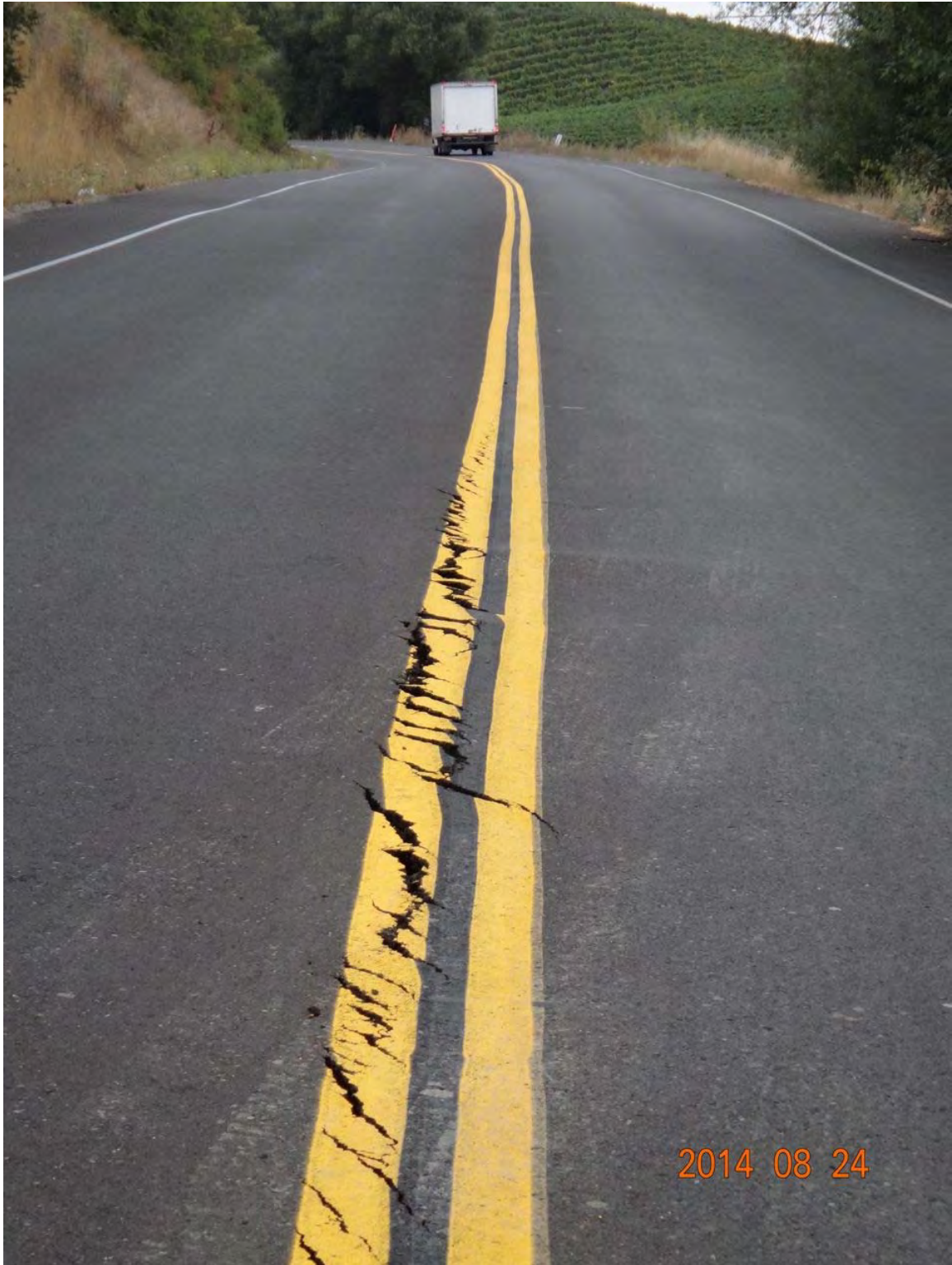
Figure 22. Surface deformation at Old Sonoma Road (5.4 km NW of epicenter, photograph taken at 0730, about 4 hours after main shock). Compare with photograph in Figure 23 [NSF-GEER; GPS N38.2659 W122.3338; 08/24/14: 7:34 am].
