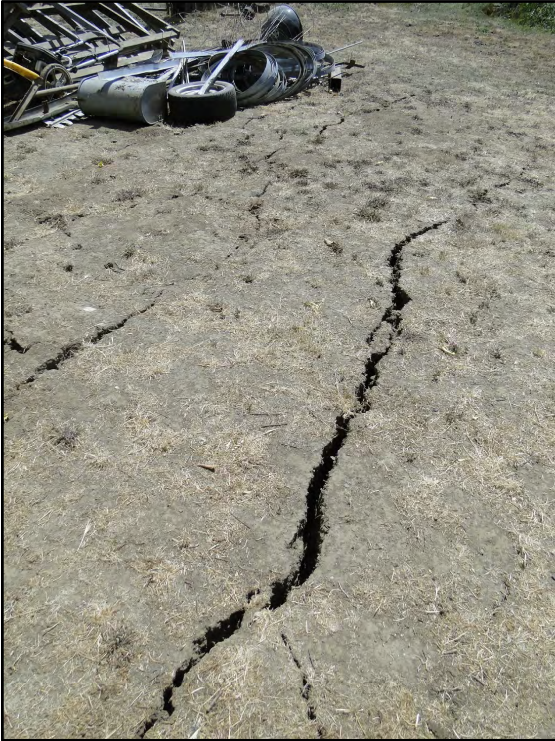
Figure 6: Photograph of ground cracking on property (Congress Valley Road, Point B4) – looking southerly between front wooden fence and towards damaged Old Sonoma Road (Point B5) [NSF-GEER; Napa, CA; N 38.284 W 122.325; Harder, L. F.; 08/29/14]
