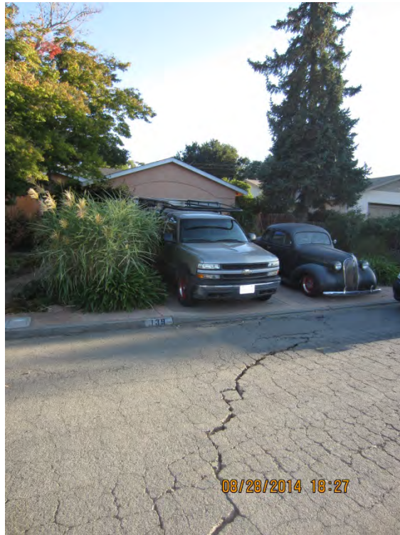
Figure C-H14-3: Street Crack. [NSF-GEER; N 38.3082 W 122.3427; 08/28/14, 18:27]
