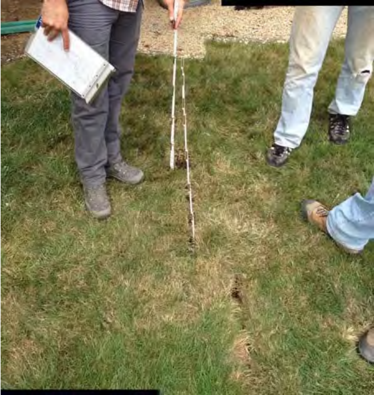
Figure C-H35-2: Fracture in grass [NSF-GEER; N 38.3015 W 122.3440; 08/25/14 10:49]
