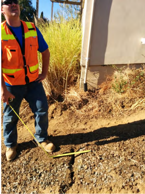
Figure C-H06-2: Soil fissure looking North. [NSF-GEER; N 38.3124 W 122.3431; 08/28/14, 17:31]
