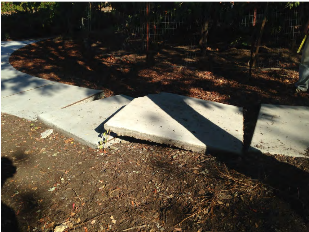
Figure D-4: Overlapping compression zone in pavement parallel to fault, near road crossing [NSF-GEER; N 38.3054 W 122.3455; 8/26/2014 17:20]
