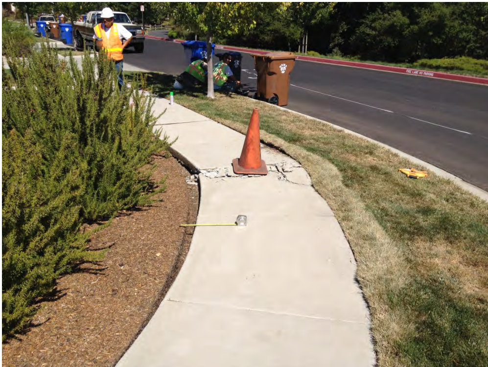
Figure D-12: Crushed section in pavement parallel to fault with compression features in curb strip perpendicular to fault, across from creek [NSF-GEER; N 38.3055 W 122.3467; 8/28/2014 14:30]
