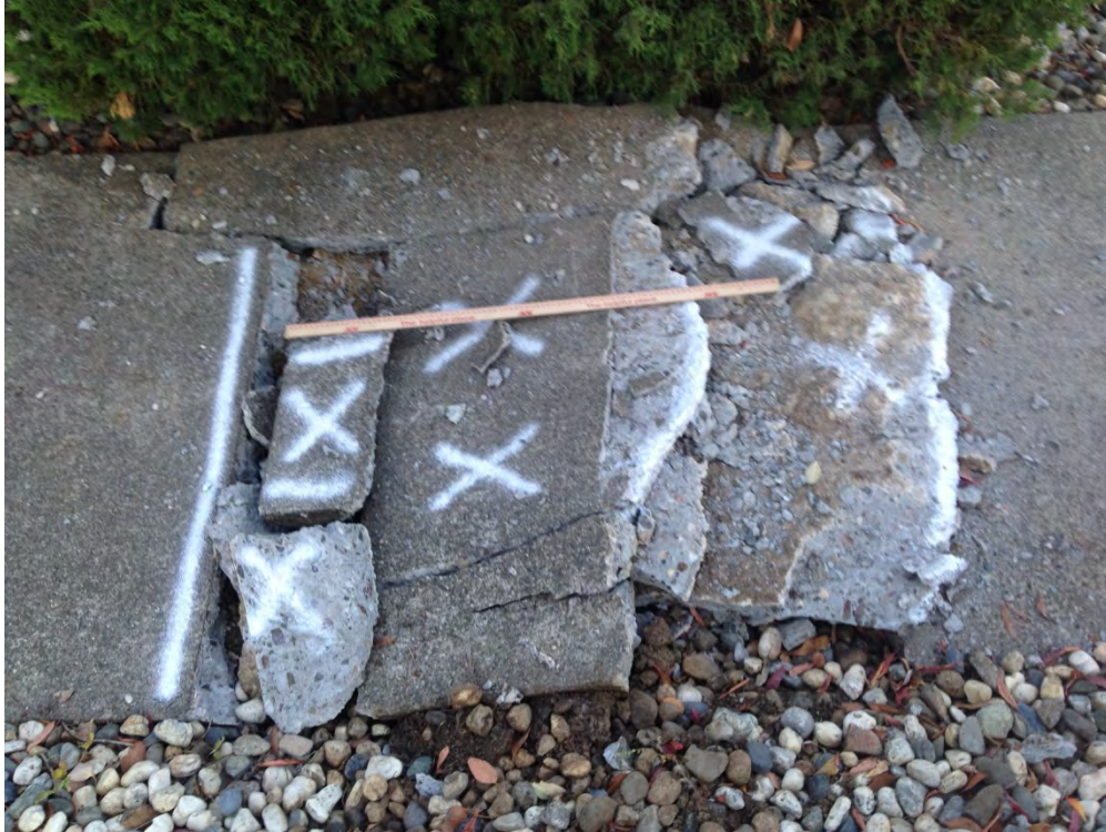
Figure D-5: Buckled and crushed compression zone in pavement parallel to fault [NSF-GEER; N 38.3048 W 122.3460; 8/26/2014 18:52]
