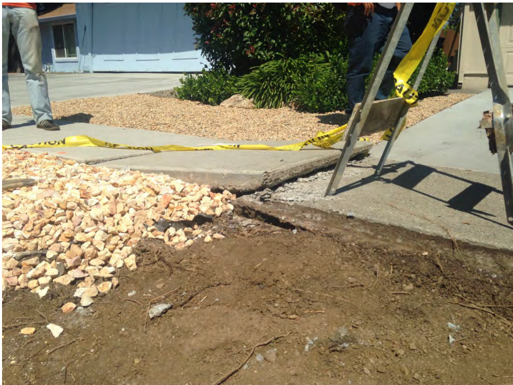
Figure D-6: Overlapping compression zone in pavement perpendicular and adjacent to fault [NSF-GEER; N 38.3025 W 122.3436; 8/27/2014 12:01]
