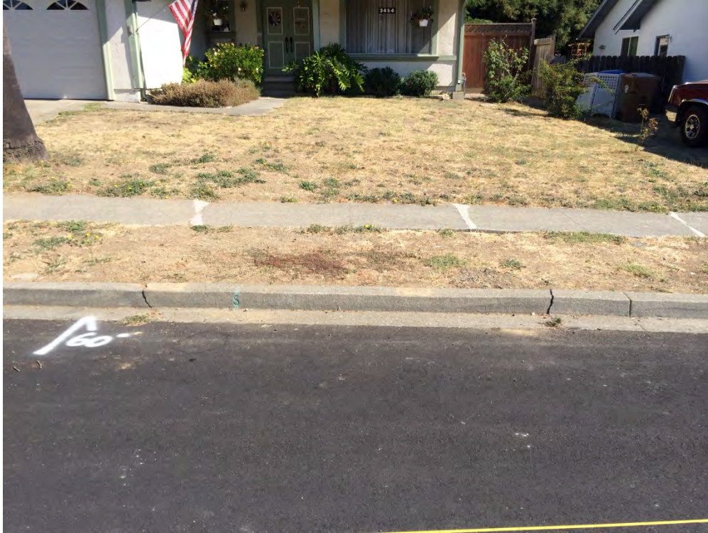
Figure D-19: Buckled curb adjacent to pavement perpendicular to fault trace; visible cracking in soil aligns with cracks in curb [NSF-GEER; N 38.3027 W 122.3407; 8/28/2014 10:25]
