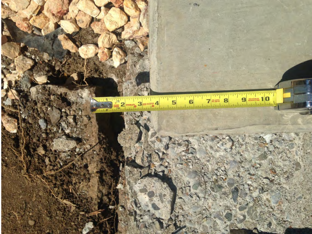
Figure D-7: Lateral offset of overlapping compression zone in pavement perpendicular and adjacent to fault; offset is parallel to fault [NSF-GEER; N 38.3026 W 122.3437; 8/27/2014 12:02]
