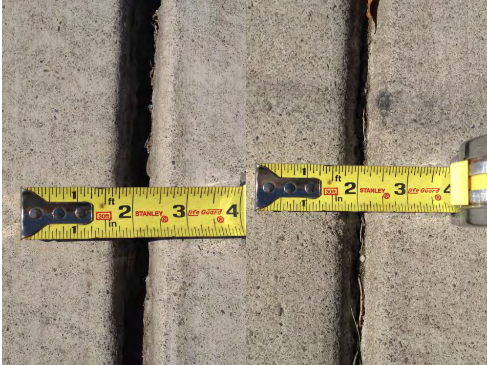
Figure D-9: Typical extension cracks in thermal joints of sidewalk pavement parallel to fault; ~13mm gap (left), ~7mm gap (right) [NSF-GEER; N 38.3067 W 122.3464; 8/28/2014 15:18]
