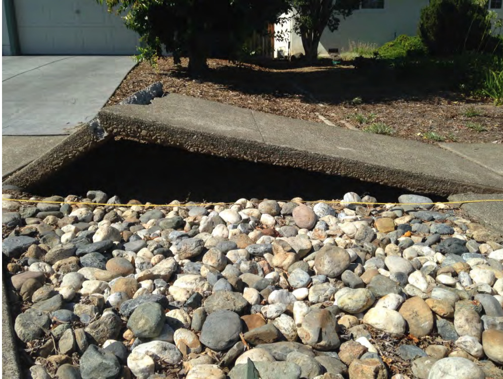
Figure D-3: Typical buckled compression zone in pavement perpendicular to fault, near observed fault trace [NSF-GEER; N 38.3039 W 122.3430; 8/26/2014 15:24]
