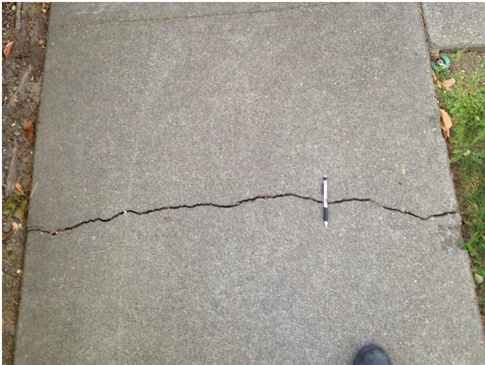
Figure D-10: Extension crack in sidewalk pavement parallel to fault; ~3mm gap [NSF-GEER; N 38.3055 W 122.3454; 8/26/2014 18:30]
