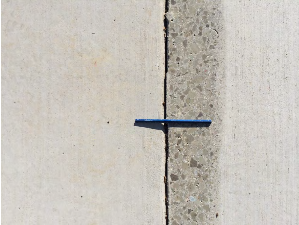
Figure D-11: Example of extension crack not considered due to shaved concrete [[NSF-GEER; N 38.3021 W 122.3430; 8/28/2014 09:17]
