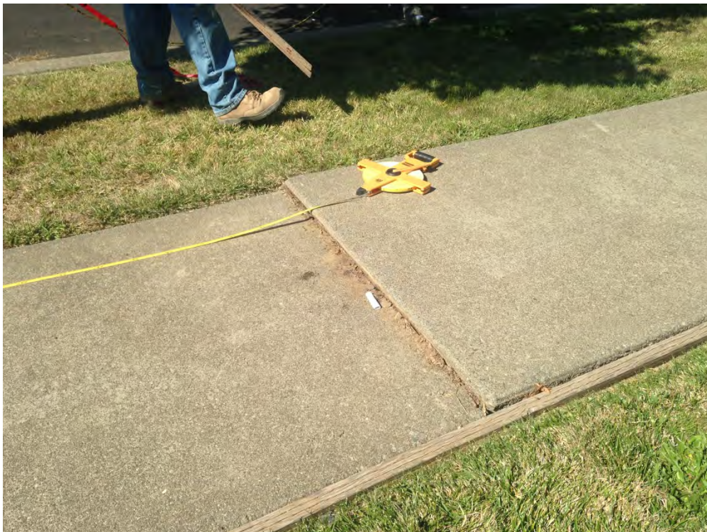
Figure D-8: Slight uplift in compressed zone of pavement perpendicular and near fault [NSF-GEER; N 38.3037 W 122.3430; 8/26/2014 15:48]
