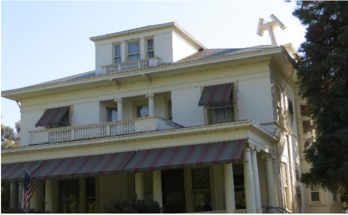
Figure E.10: Metal chimney, no damage [NSF-GEER; GPS N38.097 W122.272; 08/24/14; 17:06]
