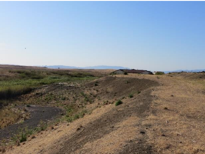
Figure E.24: Surcharge slope, no damage [NSF-GEER; GPS N38.092 W122.277; 08/24/14; 17:51]
