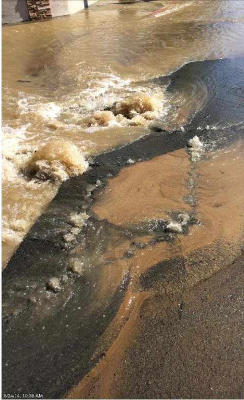
Figure E.26: Water main break at Napa Valley Mobile Home Park [NSF-GEER; N 38.3465 W -122.330; 08/24/14 10:39]
