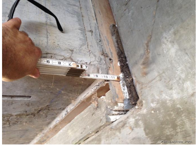
Figure E.38: of the deck in 3 rd St. Bridge East abutment [NSF-GEER; N 38.2981 W -122.284; 08/24/14 14:44]
