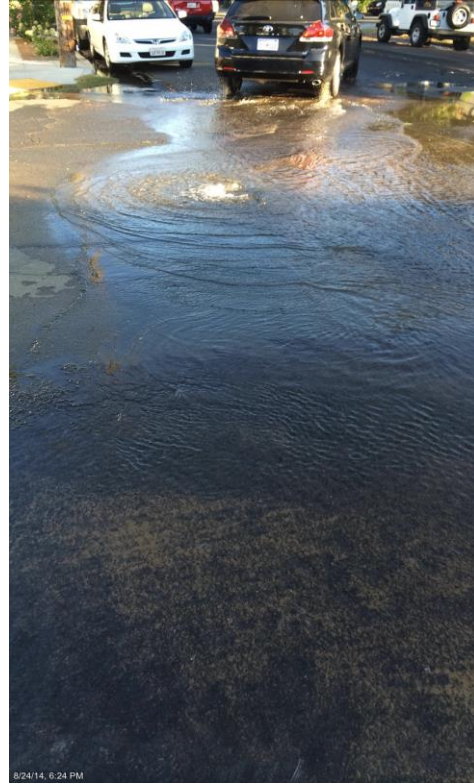
Figure E.27: Water main break at Brown St. (Downtown Napa) [NSF-GEER; N 38.3016 W -122.288; 08/24/14 18:24]
