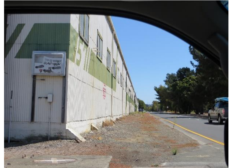
Figure E.7: Corrugated siding, no damage [NSF-GEER; GPS N38.110 W122.283; 08/24/14; 13:54]
