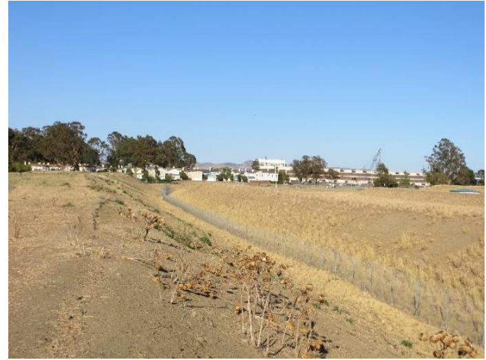
Figure E.23: Slopes, no damage [NSF-GEER; GPS N38.092 W122.277; 08/24/14; 17:53]
