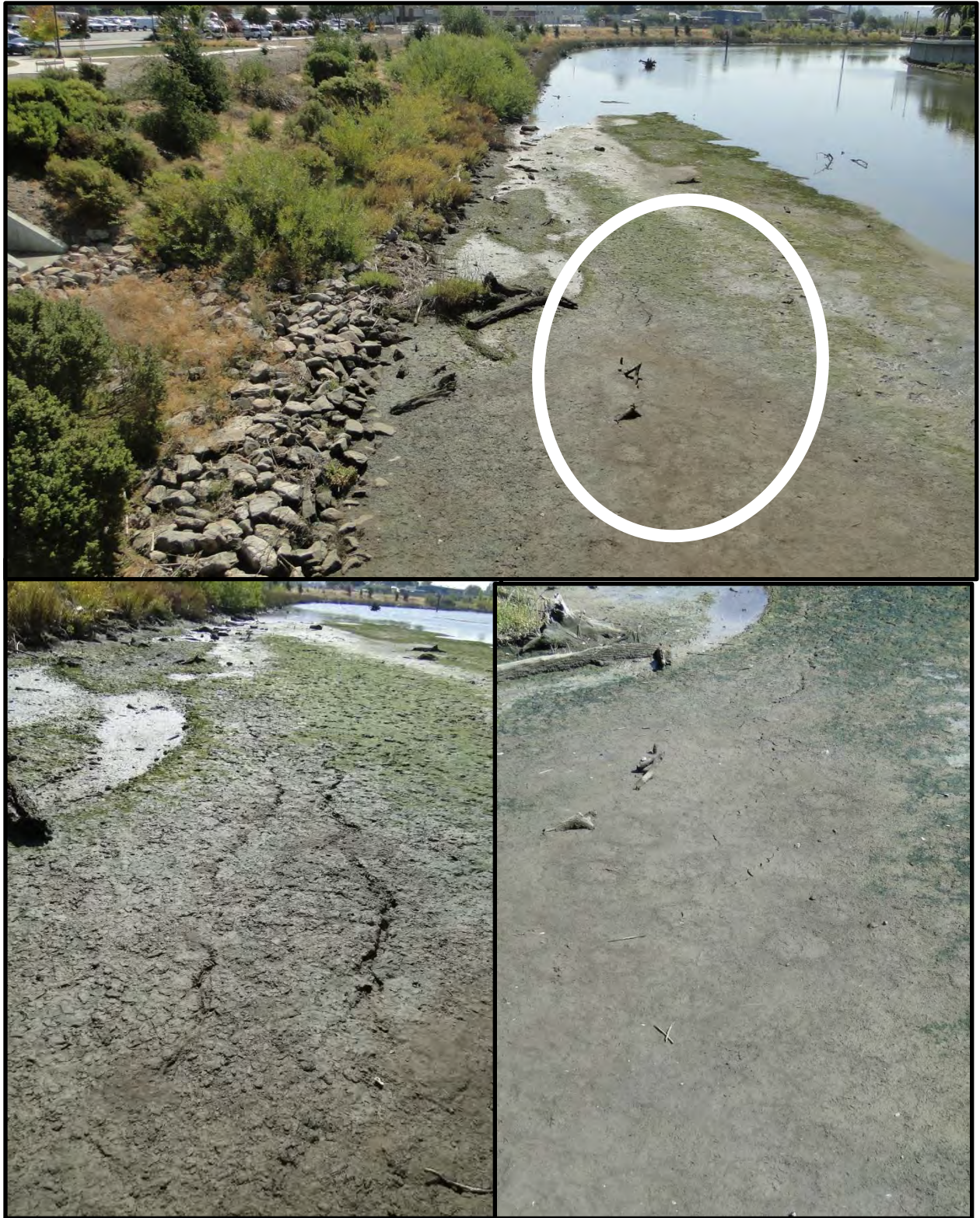
Figure F-18: Remnant cracking and sand boils in sand bar along left bank of Napa River looking downstream from Third Street Bridge [NSF-GEER; Napa, CA; N38.298 W 122.283; Harder, L. F.; 09/04 and 09/07/14]
