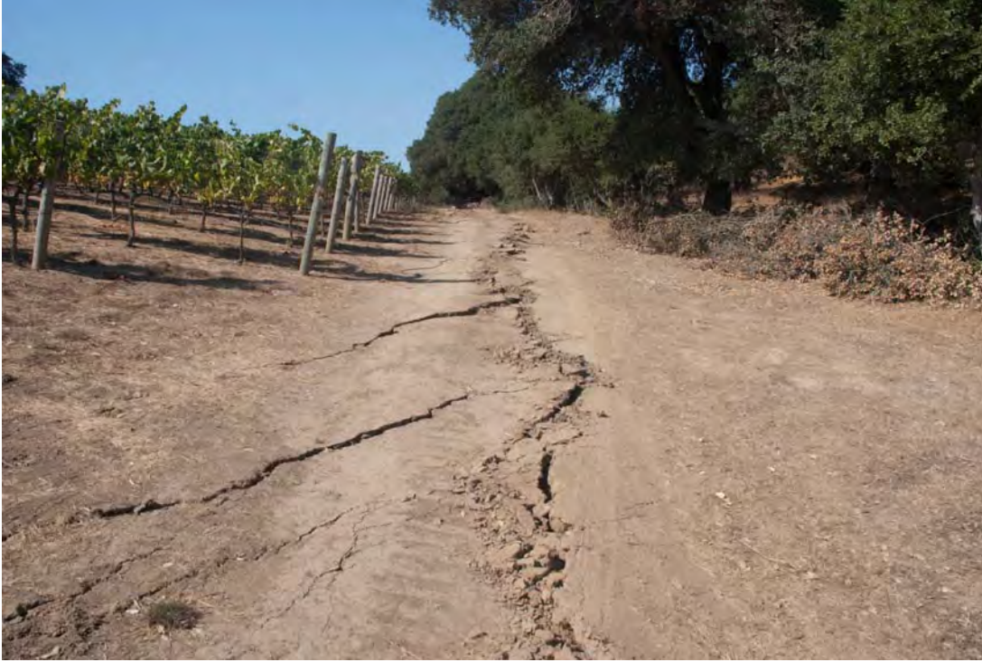
Figure 3-8. Rupture west of Buhman Avenue. Right-lateral displacement was on the order of 40 cm, with a small amount (~12 cm) of up-on-the-west vertical displacement. [NSF-GEER; GPS: 38.2924°, -122.3432°; 08/25/2014]
