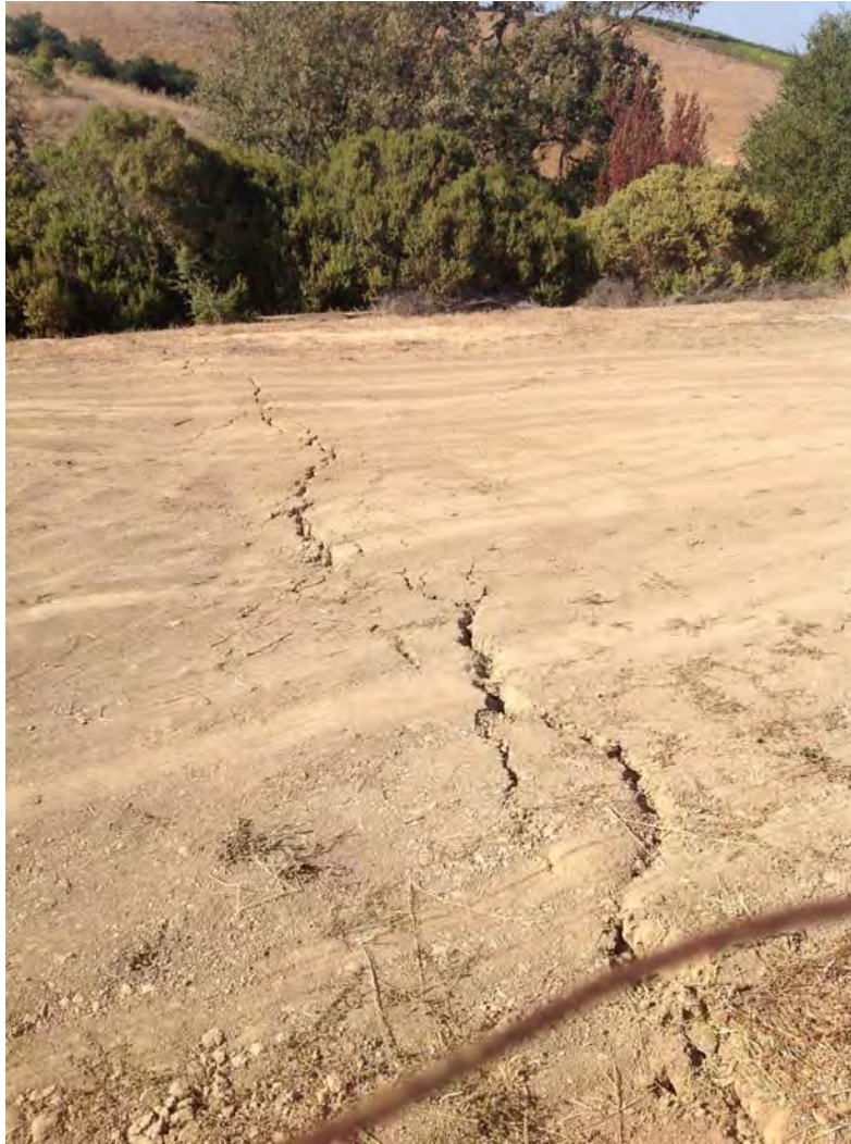
Figure 3-11. Surface rupture near northern boundary of Alston Park. Note left-stepping pattern of extensional cracking, suggestive of right-lateral displacement, which was about 4-5 cm at this location. [NSF-GEER; GPS 38.3263°, -122.3459°; 09/01/2014]
