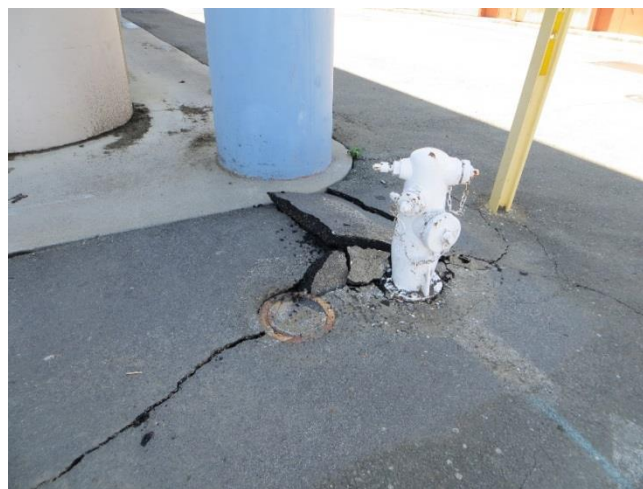
Figure 6.5: Pavement damage at hydrant; [NSF-GEER; Mare Island, Vallejo, CA; GPS N38.098 W122.269; 08/24/14; 14:37]
