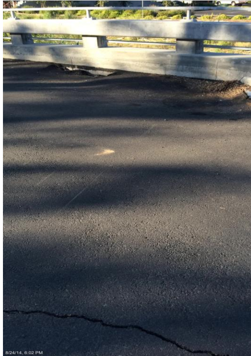
Figure 6.12: Settlement of backfill near the retaining wall in the pedestrian bridge [NSF-GEER; N 38.3003 W -122.2881; 08/24/14 17:58]
