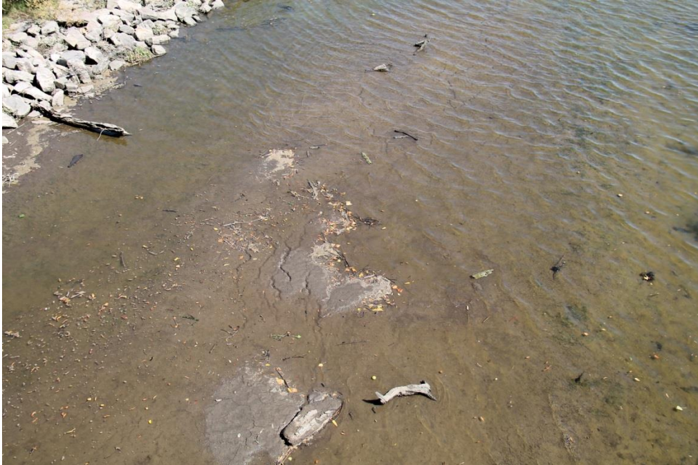
Figure 6.7: Ground cracking and submerged sand boils due to liquefaction in Napa River point bar, east bank, south of 3 rd St. Bridge [NSF-GEER; N 38.2980 W -122.2830; 08/24/14 14:44]
