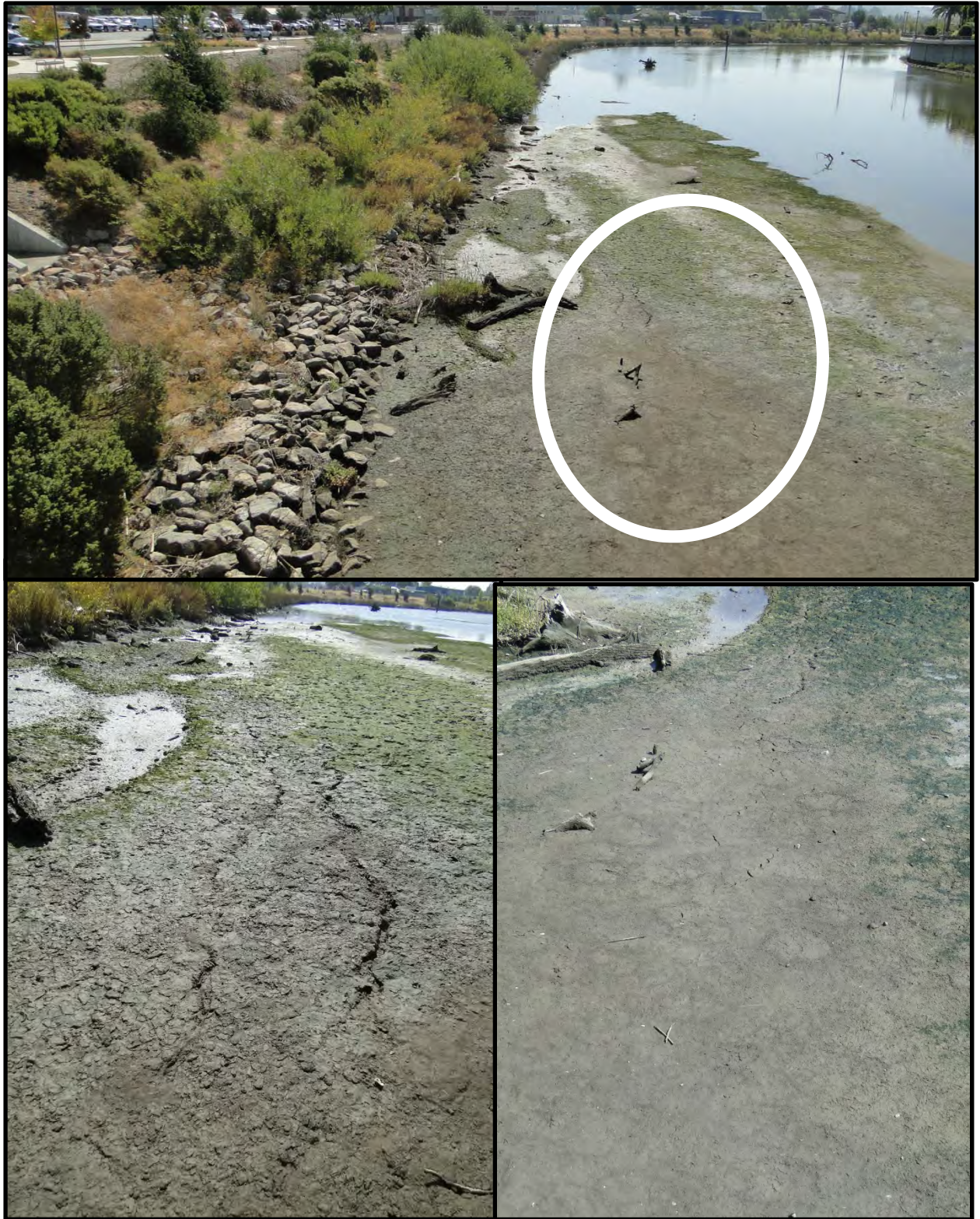
Figure 7-13: Remnant cracking and sand boils in sand bar along left bank of Napa River looking downstream from Third Street Bridge [NSF-GEER; Napa, CA; N38.298 W 122.283; Harder, L. F.; 09/04 and 09/07/14]
