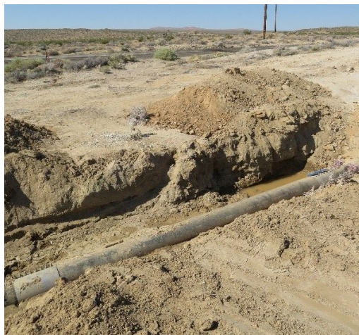
Figure 29. Pipeline damage at M6.4 surface rupture crossing. (a) broken pipeline at west side of rupture zone photographed before repair on 7/4/2019 (B. Brooks, USGS). (b) repaired pipeline at west side of fault zone. (c) repaired pipeline at east side of fault zone. (d) leak within fault zone after M7.1 earthquake. (35.6443, -117.5369)
