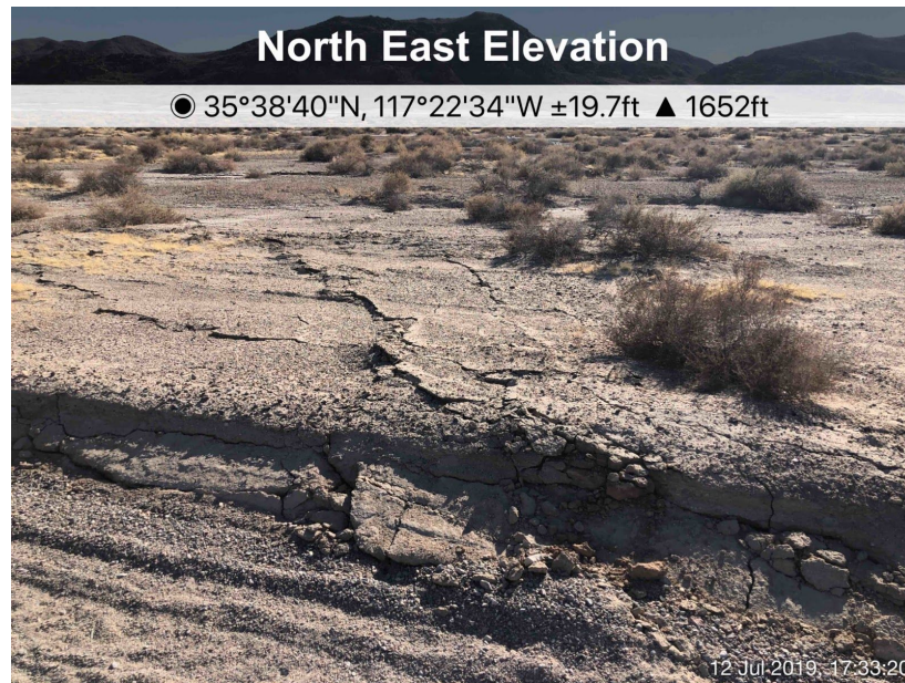
Figure 27. Example of cracks observed along Pinnacles Road. This specific picture was taken at zone 3 and shows where the cracks cut the Pinnacles Road.
