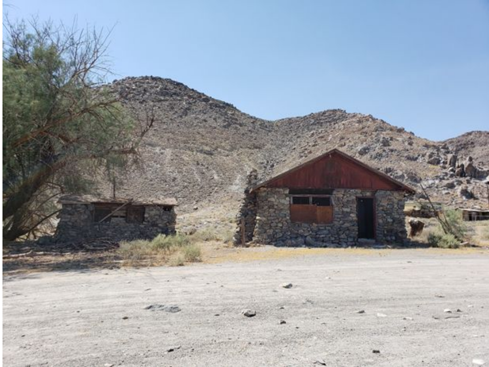
Figure 45. Example of less-heavily damaged Structure A2, not in vicinity of liquefaction – induced ground effects (at base of mountain). (35.7484, -117.3988)
