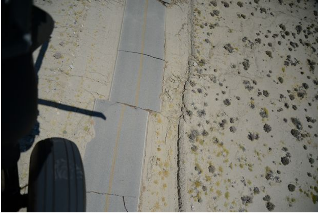
Figure 8. Helicopter overflight viewing access road fault offset. The CGS and USGS, along with National Guard and Navy personnel, view road damage showing 2.5 \pm 0.2 m of right-lateral motion along the primary rupture associated with the magnitude 7.1 event. This offset access road was broken by the mainshock fault rupture about 800 m southeast of the China Lake playa (Credit: Ken Hudnut, USGS. Public domain)
