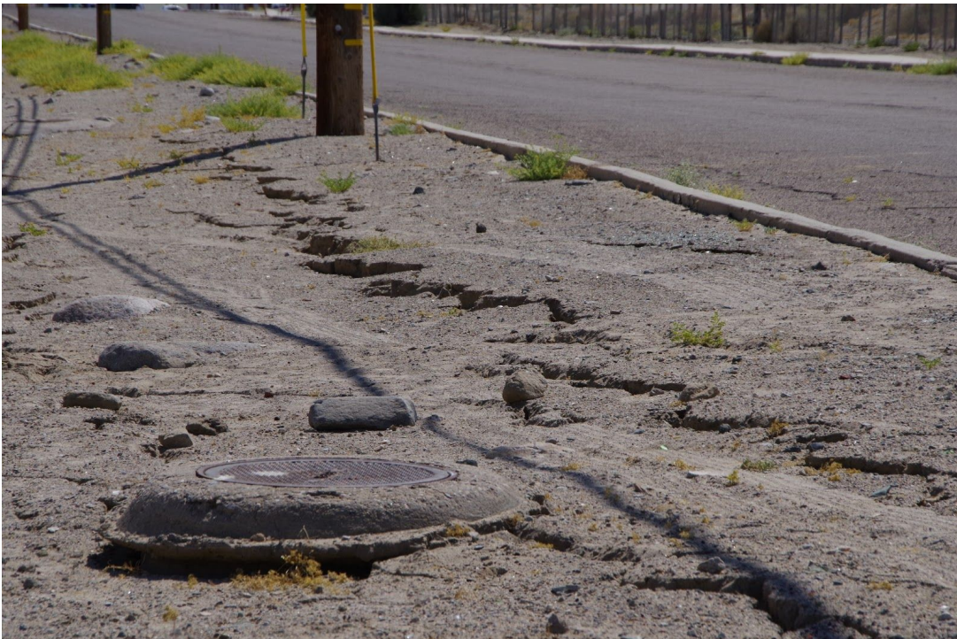
Figure 35. Ground cracks due to liquefaction-induced lateral spreading in Trona. Photo by Scott Brandenburg, (35.7626, -117.3731).
