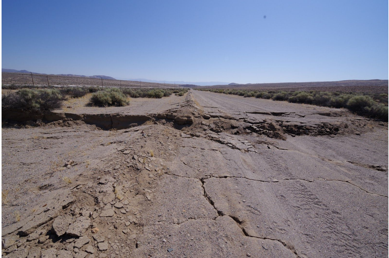
Figure 24. Fault rupture from the M7.1 event showing at a road crossing south of Highway 178 (35.6468, -117.4800). Photo credit Scott Brandenburg.
