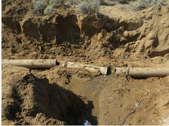
Figure 30. Offset of buried concrete segmented pipeline crossing the M7.1 surface fault rupture. (35.6492, -117.4822).
