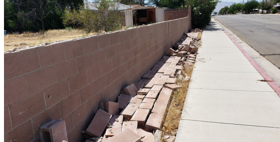
Figure 51. Damages to Masonry components after the M7.1 event (a: 35.7595, -117.7357, b: 35.7592, -117.3766, c: 35.7595, -117.7357, d: 35.6444, -117.6720) Photo credit: Christine Goulet and Jawad Fayaz
