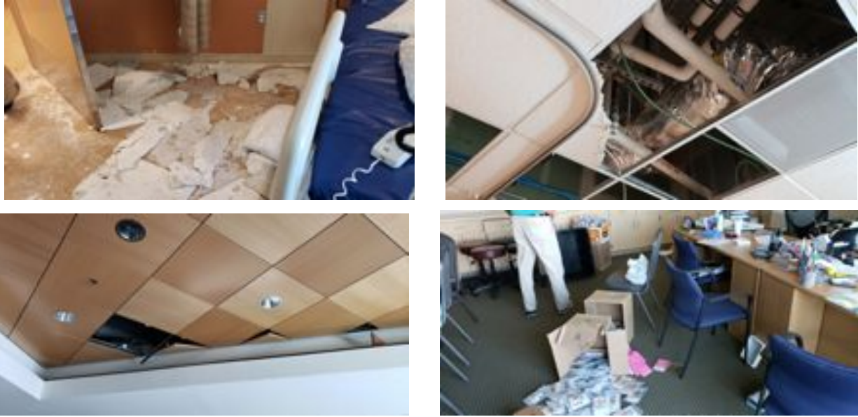
Figure 50. Damages to Ridgecrest Regional Hospital after the M7.1 event (35.6410, -117.6707) Photo credit: Jawad Fayaz
