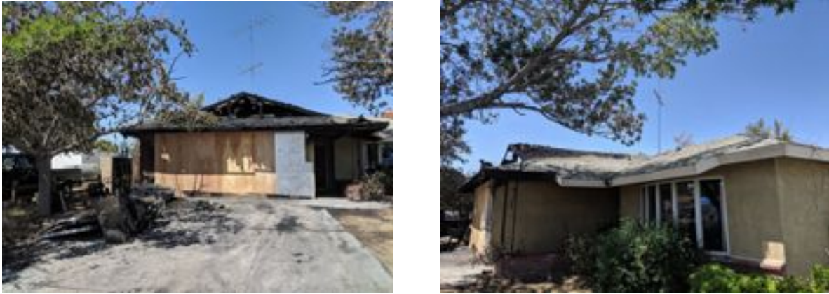
Figure 46. Damaged wood-frame house due to gas leak fire in Ridgecrest (35.6202, -117.6612) Photo credit: Farzin Zareian
