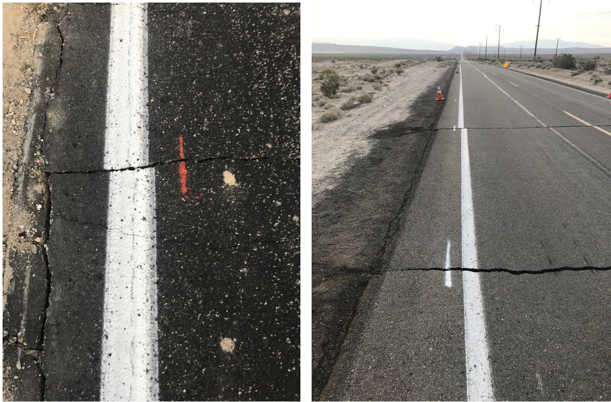
Figure 13. Pavement of Highway 178 offset by M6.4 event fault rupture (shown by white lines) and short painted lines used to monitor afterslip. Locations: Left 35.649, -117.4824 (red line), Right 35.6441, -117.537 (white line). Photo credits: Ben Brooks, USGS
