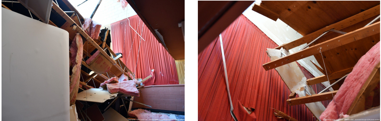
Figure 52. Observation of collapsed roof in Ridgecrest Cinema after M7.1 event (35.6499, --117.6715) Photo credit: Fred Turner
