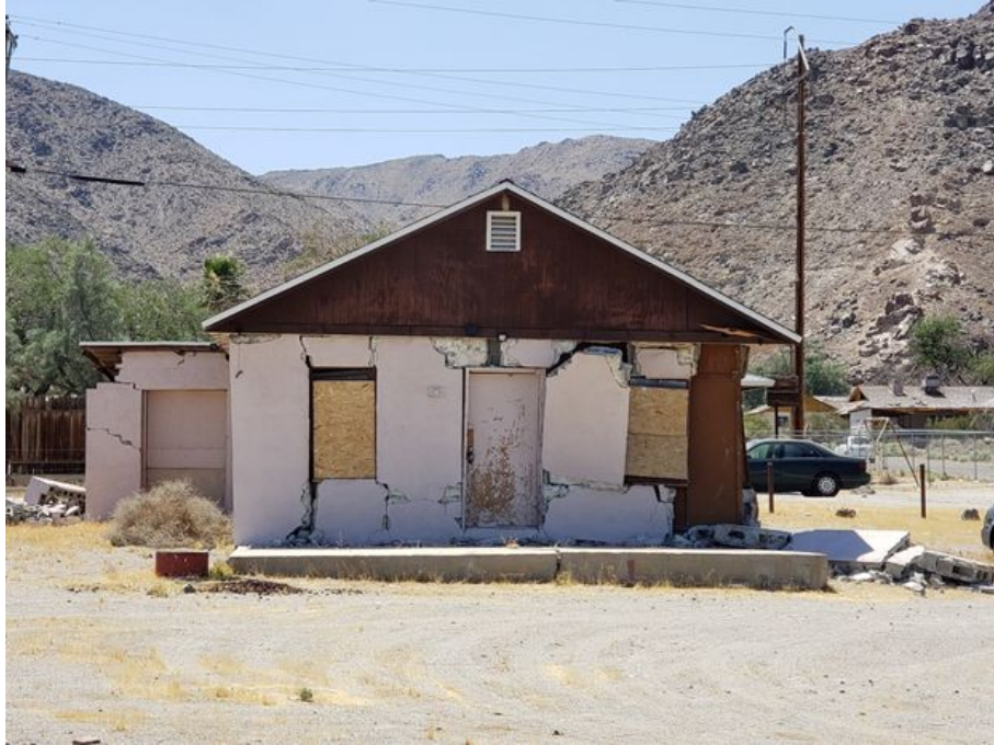
Figure 43. Example of more heavily damaged Structure A1 in vicinity of liquefaction – induced ground cracking (upon alluvial fan deposits – see canyon visible behind structure). (35.7457, -117.3964)
