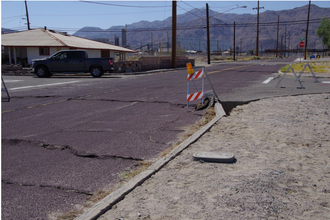
Figure 36. Ground compression, including buckled curb, due to liquefaction-induced lateral spreading in Trona. Photo by Scott Brandenburg, (35.7623, -117.3725).
