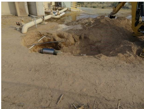
Figure 28. Hilltop Tank elephant foot buckle, pipe repair and continued leaking (35.6260, -117.5916).
