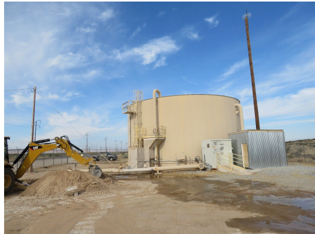
Figure 28. Hilltop Tank elephant foot buckle, pipe repair and continued leaking (35.6260, -117.5916).
