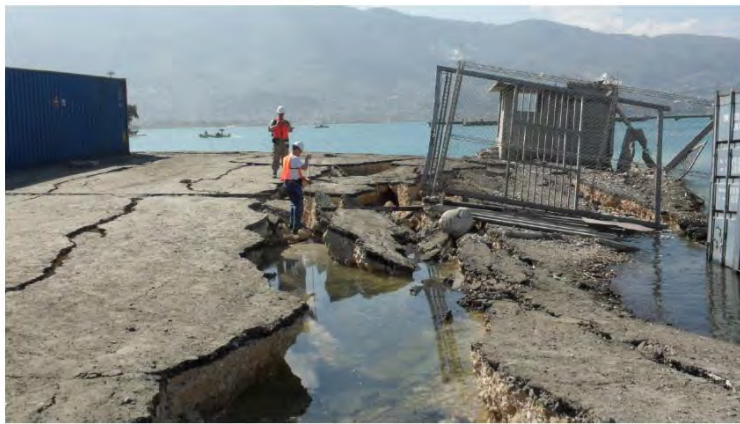
Figure 6.9 Lateral spreading under the two metal warehouses. Photo taken facing south with the metal warehouses to the left. (N18.557075, W72.352045)
