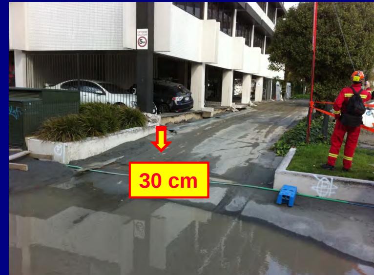
Settlement of Ground next to Piled Bldg.
