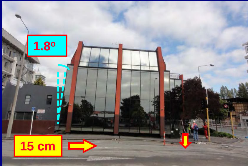
Tilting and Sliding of Buildings
