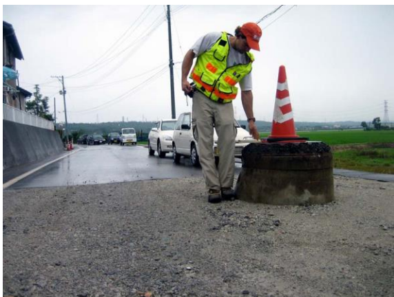
Figure 1. GEER investigator measures buoyant civil-municipal utilities in liquefied soil, Kashiwazaki, Japan, 2007 (Site RK-14,
